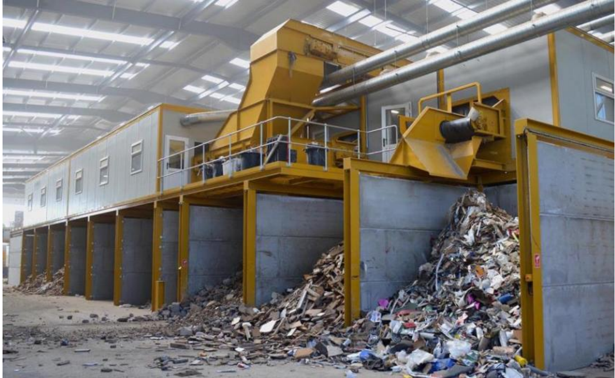
Figure 8: Construction & demolition waste recycling facility
