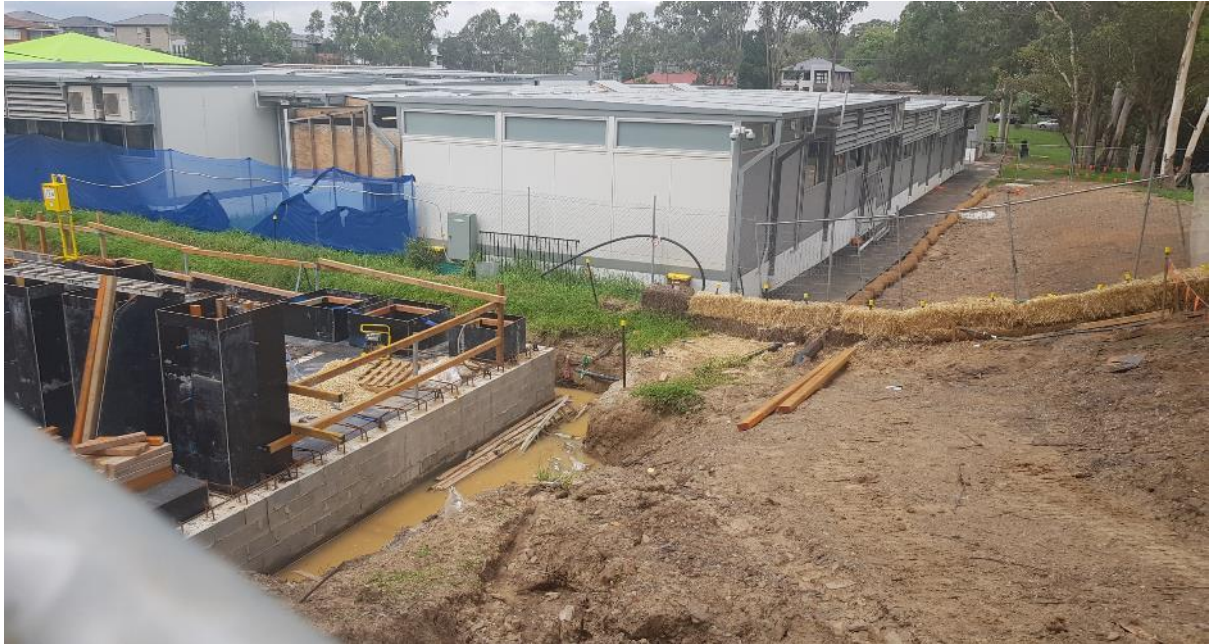
Photo 9: Location of OSD Tank overflow and discharge from 10/02/20. Note remedial works and
