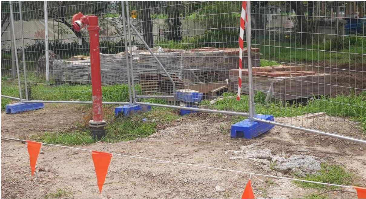
Photo 6: Material stored within TPZ
