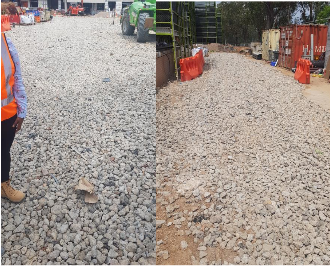
Photo 5a and 5b: Fresh placement of rock on internal haul road following rain events in February 2020.
