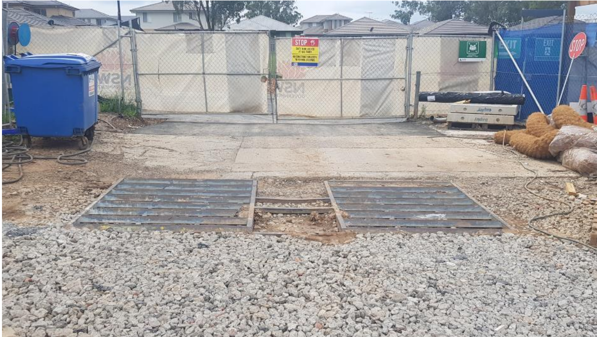
Photo 4: St Albans Road exit. No issues.
