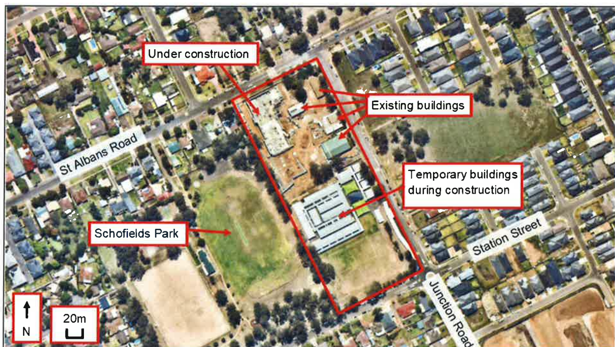
Figure 2 | Existing School Site (Base source: Nearmap 2019)
