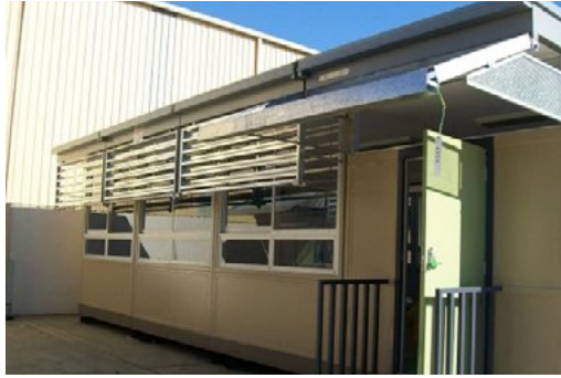
Photograph 01: Old system demountable showing typical wall panels and windows – view from front
