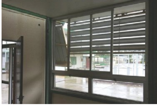
Photograph 05: Typical windows – view from inside demountable
