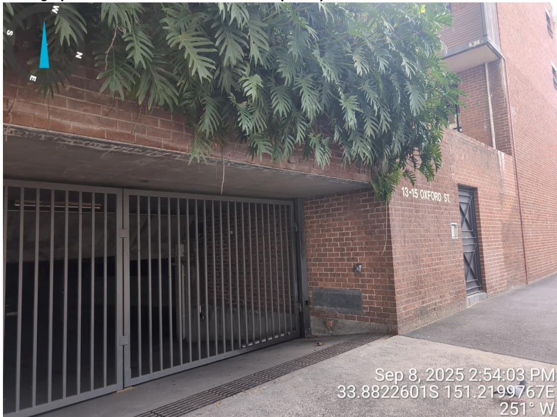
Photograph 2: Front view of 13-15 Oxford Street (8/9/25)
