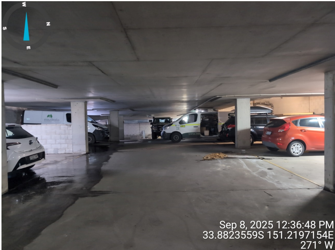
Photograph 5: View of basement 2 carpark 13-15 Oxford Street, facing west (8/9/25)
