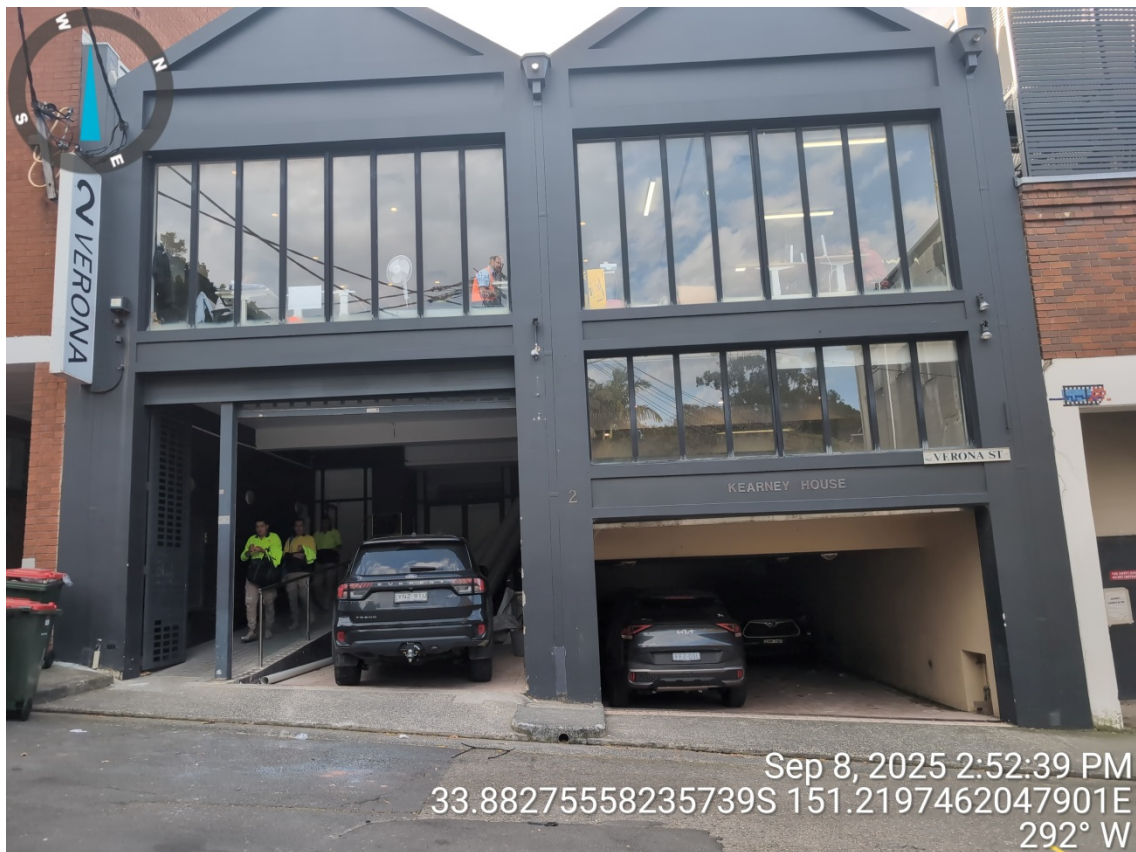
Photograph 1: Front view of 2 Verona Street (8/9/25).
