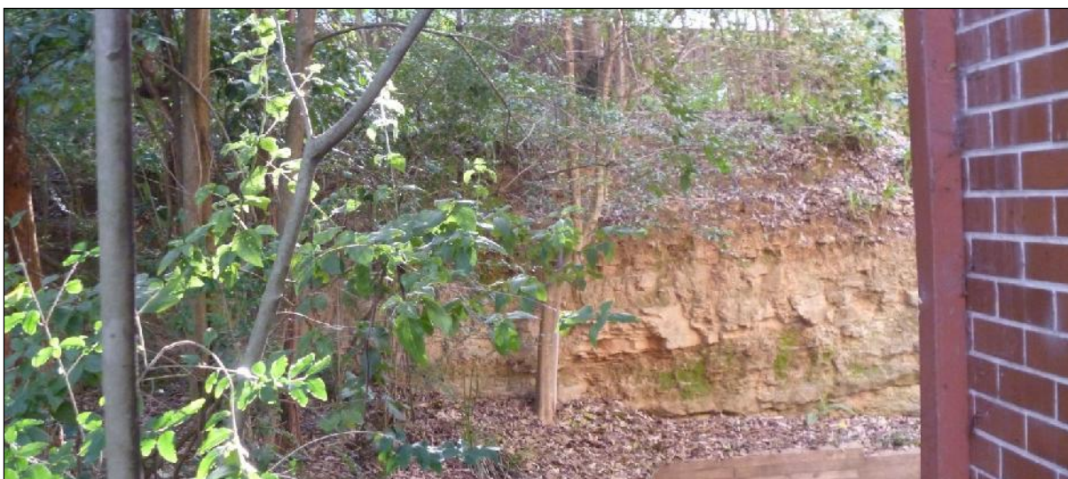
Figure 3: Exposed rock face at rear of 10 Ivanhoe Place.
