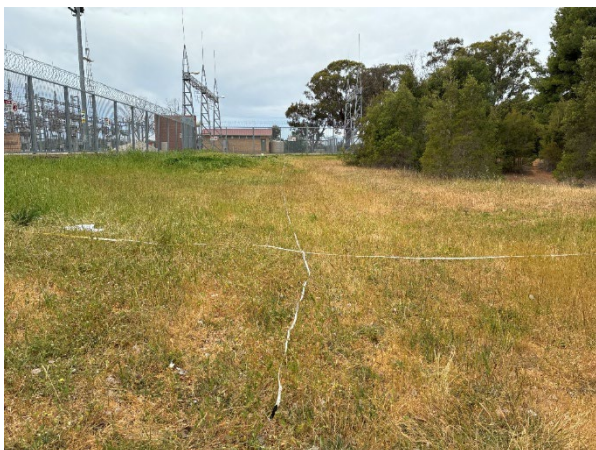
Photograph 4-11 PCT 76 DG Substation within the Subject Land
