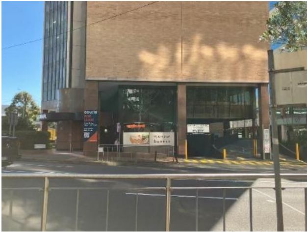
Figure 20 – View north from Help st, showing ground level
