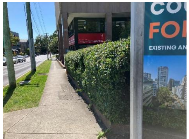
Figure 23 – view north along Pacific Highway showing underground services
