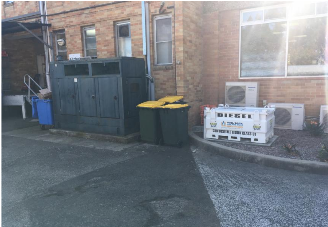
Photo 9 - Generator and diesel fuel tank
