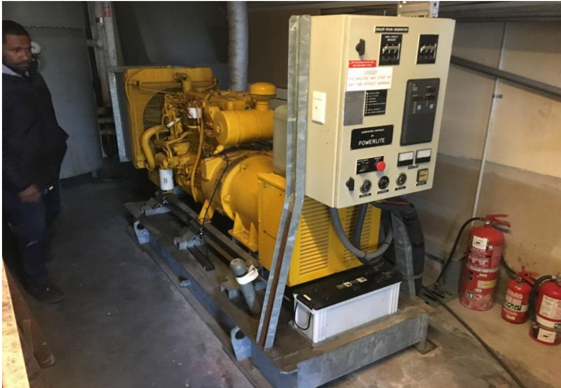
Photo 11 - Internal generator with diesel storage in base
