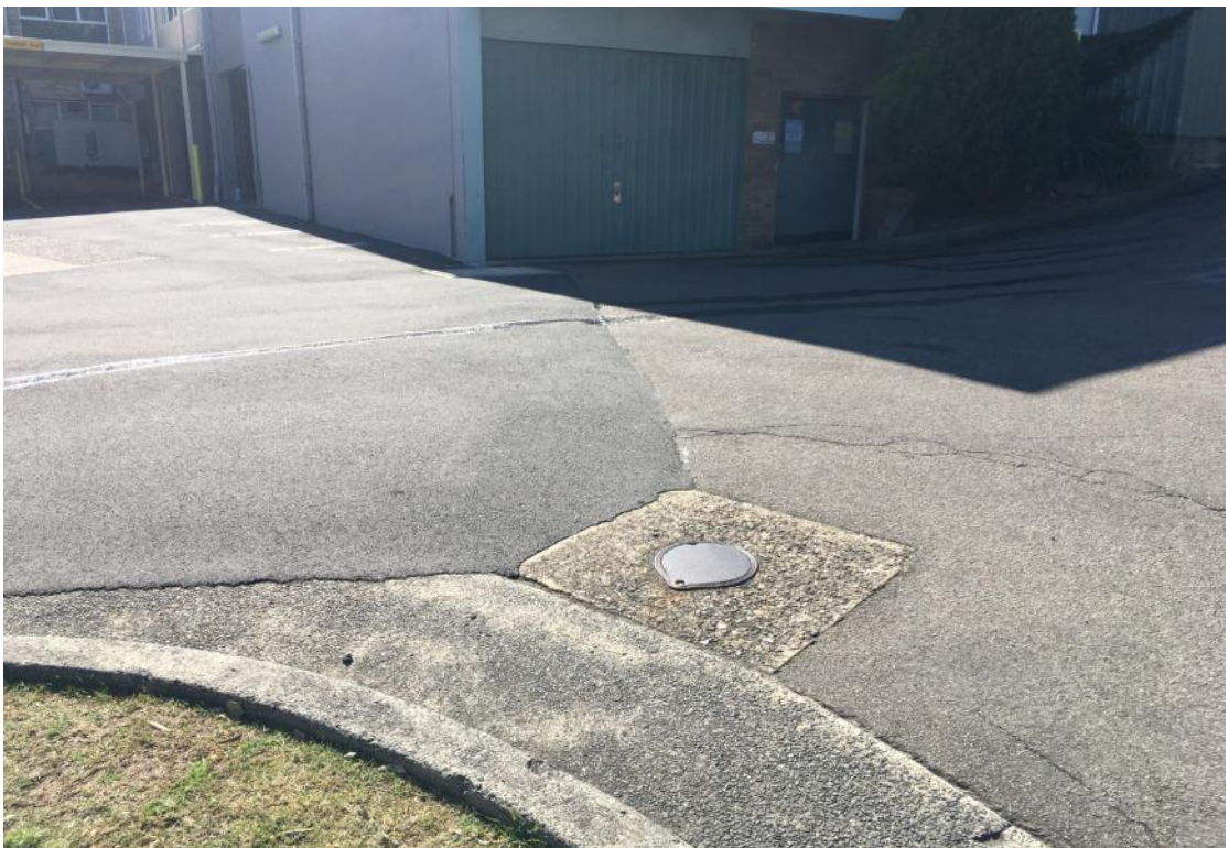
Photo 18 - Possible UST fill point (unconfirmed)
