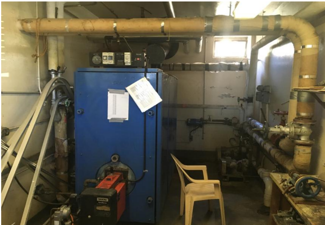
Photo 12 - One of two gas-fired boilers
