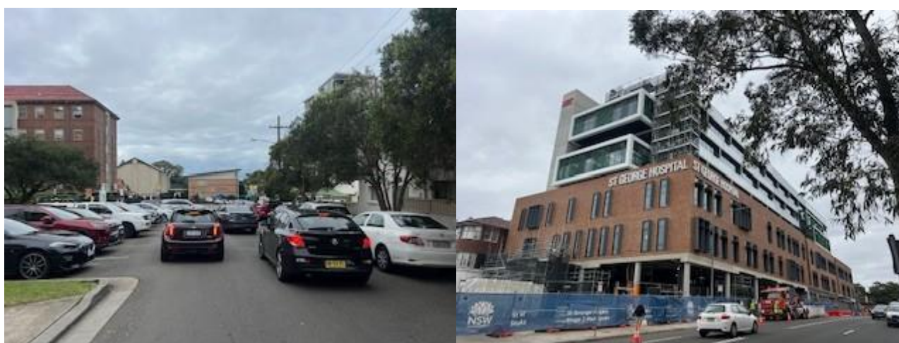
Figure 4.7 Example of Existing Congestion and SG Public Hospital Redevelopment Construction
