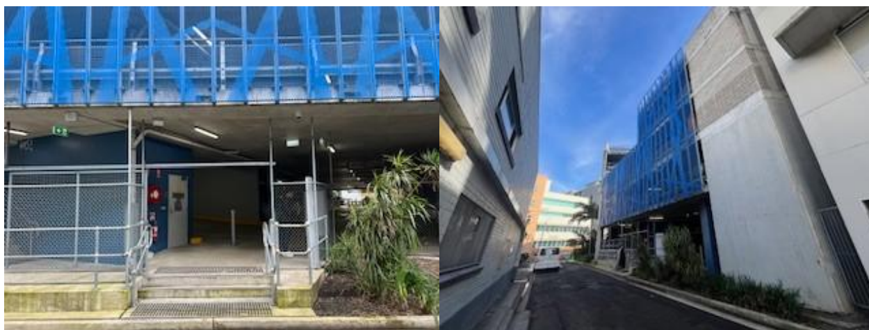
Figure 4.6 Access to the Multi-Story Carpark Access on Bank Lane
