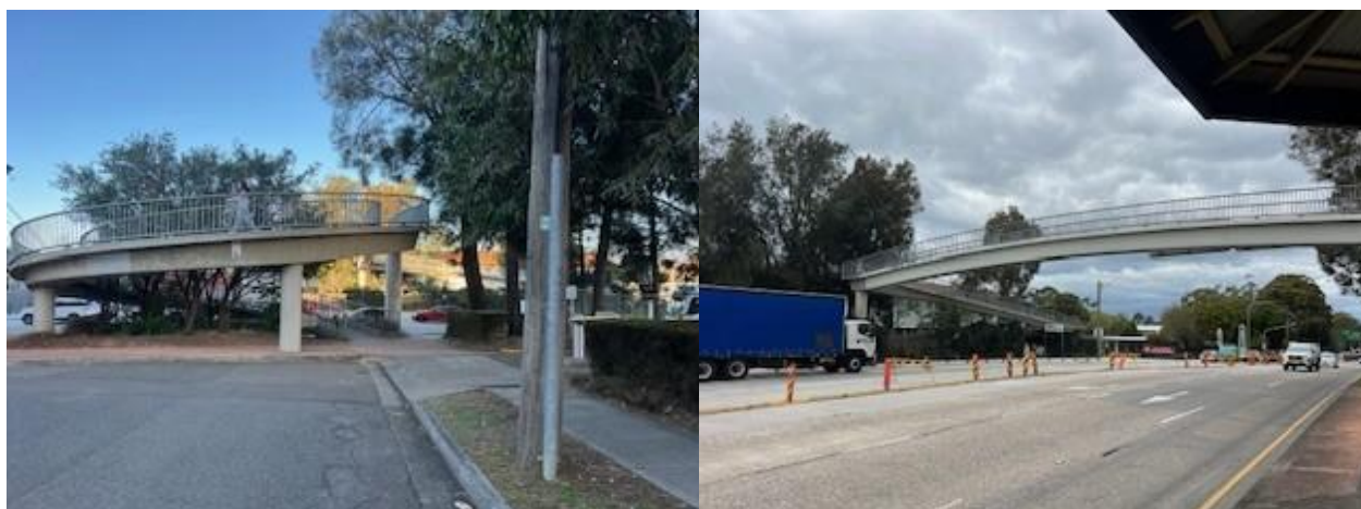
Figure 4.3 Footbridge Access on Hogben St and View from Princes Hwy
