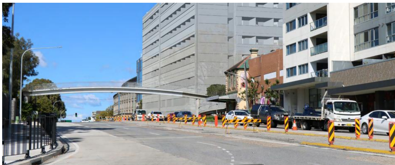
Figure 4.18 Princes Highway & President Avenue Intersection Viewpoint
