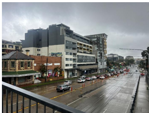
Photo 4.8 View west to the 'Shop and Residence' (#I193) item. Photo taken from the public bridge across the Princes Highway, outside the Project Area
