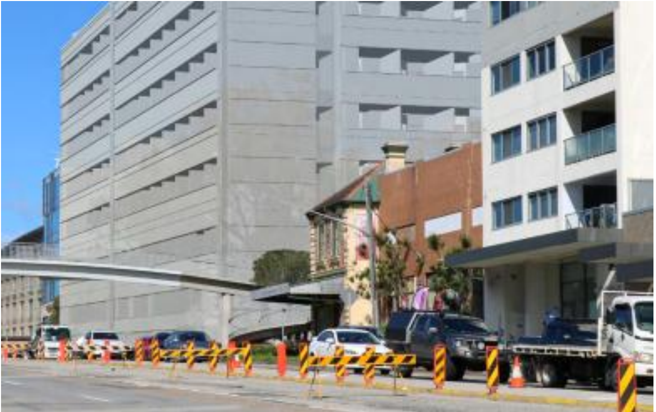
Photo 6.2 Photomontage showing the northern portion of the Project Area and #1193 'Shop and residence, view south
