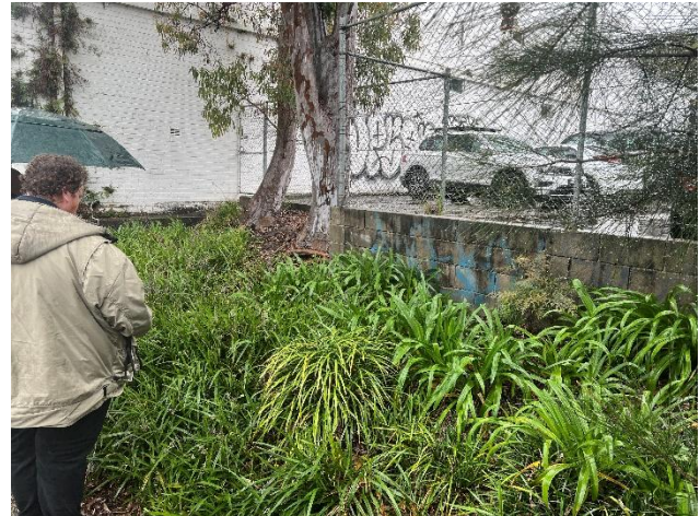
Photo 4.2 Project Area – North: View of the truncated landform and retaining wall on the eastern side of the public carpark. View south-west
