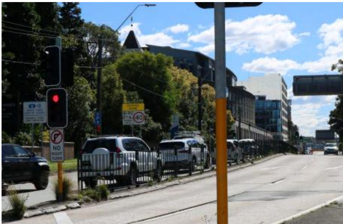
Photo 6.6 Photo montage showing the southern portion of the Project Area and #I165 'St Patrick's Catholic Church'
