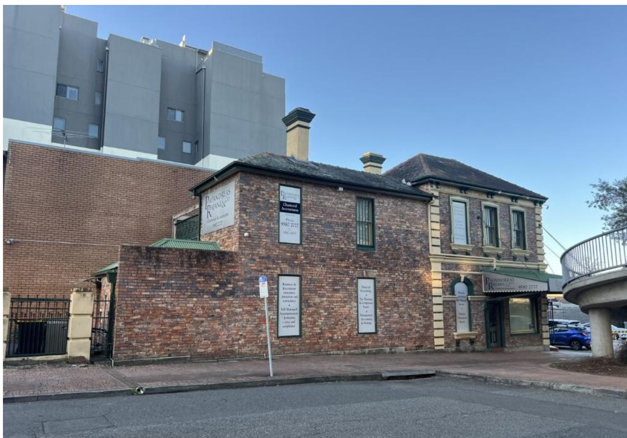
Photo 6.1 View of #193 ‘Shop and residence’, view north from the northern portion of the Project Area
