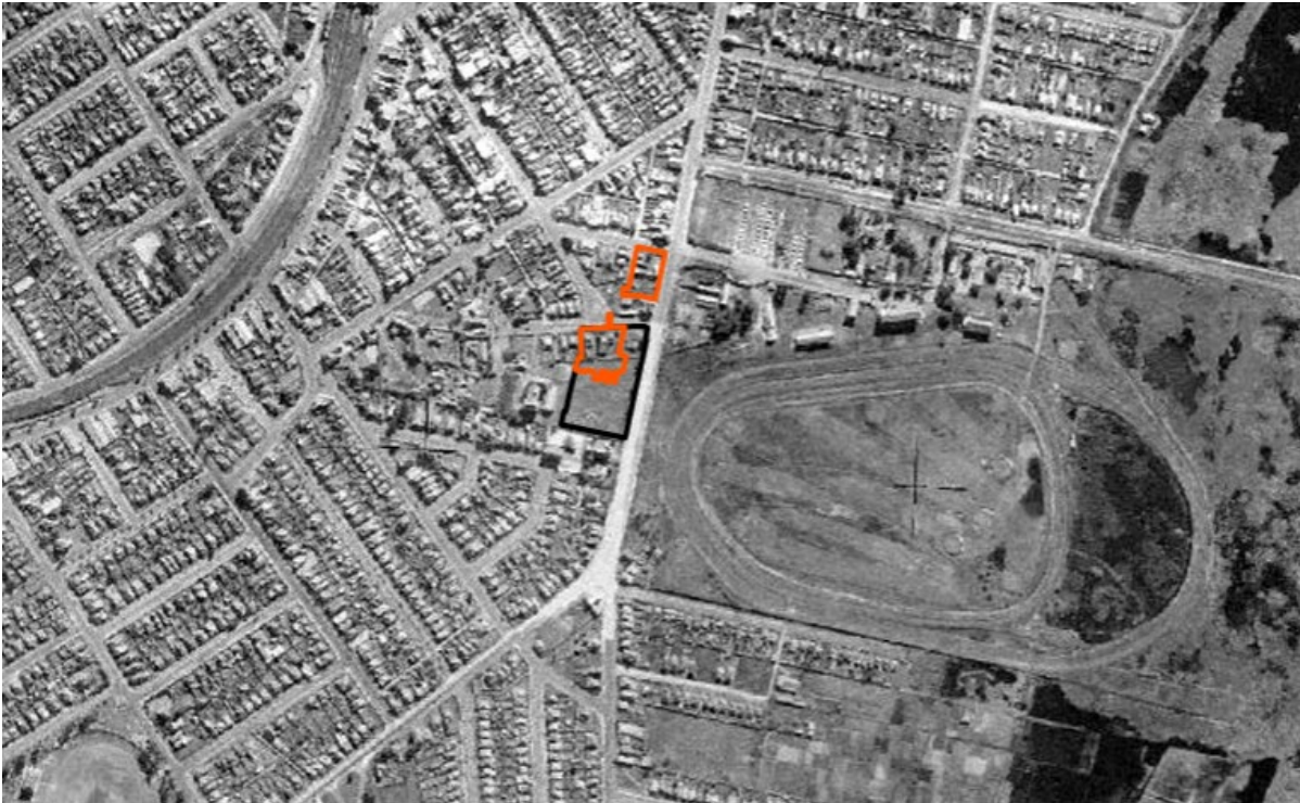
Figure 4.2 Historical Aerial Image of the Project Area (1943)
