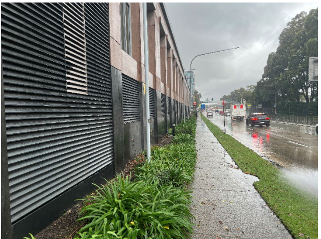
Photo 7.8 Eastern boundary of the Project Area from Princes Highway facing north
