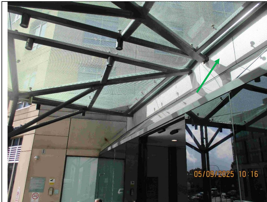
Photo 3 Northside entry bulkhead, compressed fibro cement cladding. Refer ESP Sample E89676. No asbestos detected.
