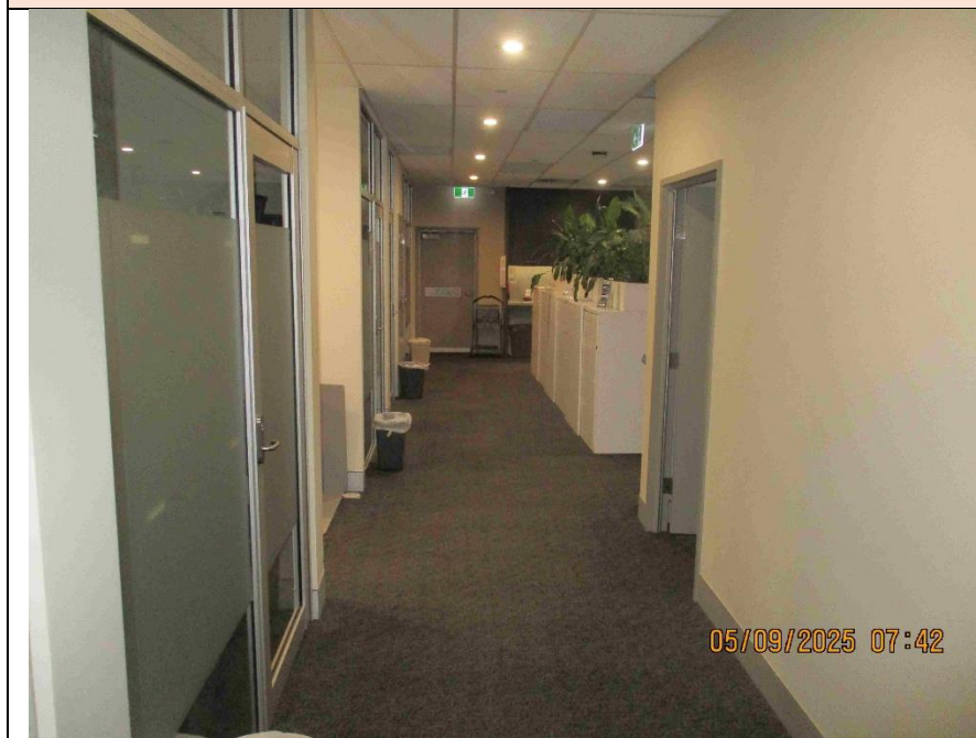
Photo 10 Typical Executive office area. No asbestos materials identified. Floor, carpet. Walls, plasterboard. Ceiling, SMF acoustic tiles.
