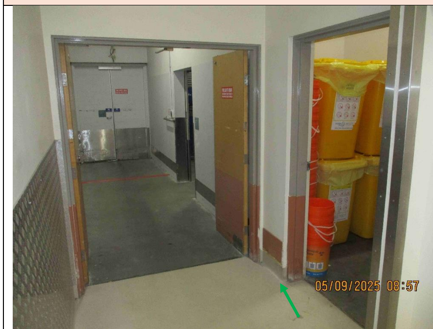
Photo 12 Corridor at Waste Bin Rooms. Floor, vinyl sheet. ESP Sample E89675. No asbestos detected.
