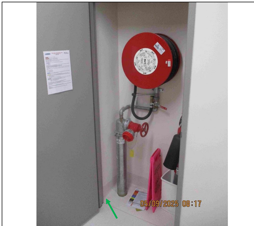
Photo 7 Fire Hose Reel cupboard at corridor to Discharge Lounge. Floor, vinyl sheet. ESP Sample E89673. No asbestos detected.
