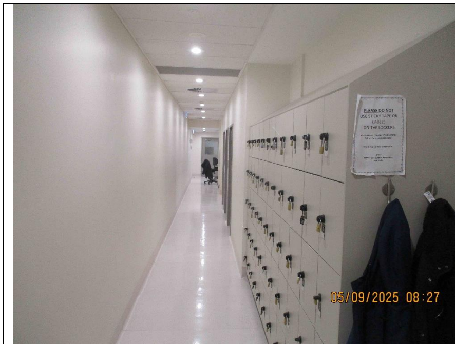
Photo 9 Corridor behind Reception area. No asbestos materials identified. Floor, vinyl. Walls, plasterboard. Ceiling, plasterboard & SMF acoustic tiles.
