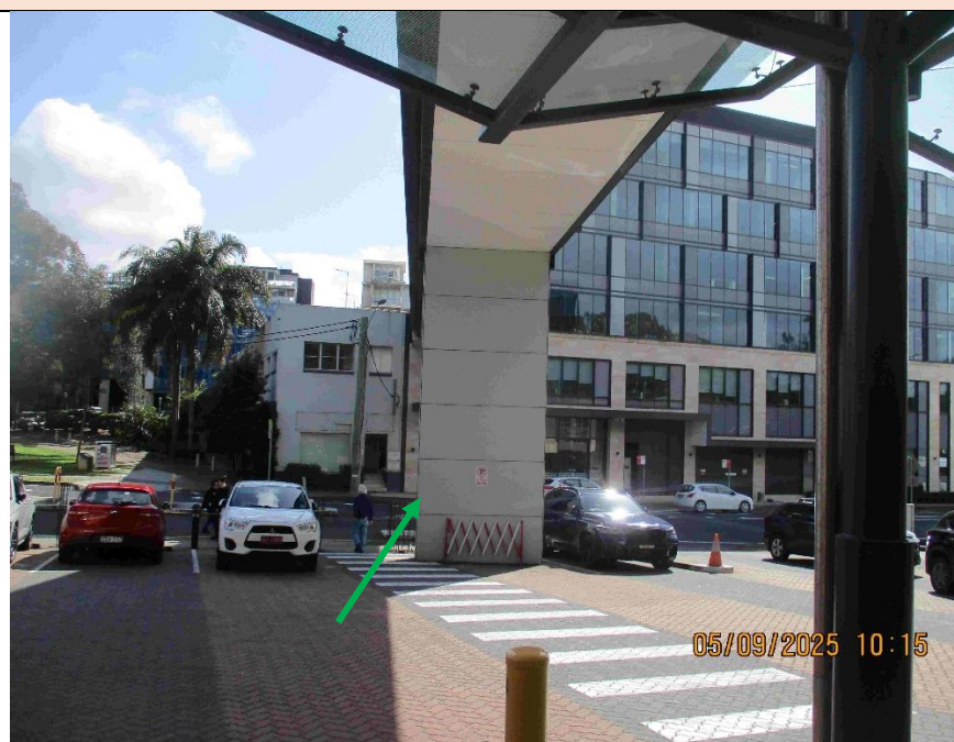
Photo 2 Northside column to overhead walkway, compressed fibro cement cladding. ESP Sample E89676. No asbestos detected.
