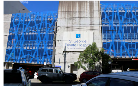
Image 12 St George Private Hospital Complex
