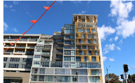
Image 5 Residential Apartment Complex
