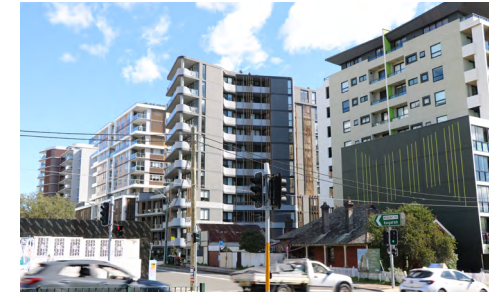
Image 6 Residential Apartment Complex
