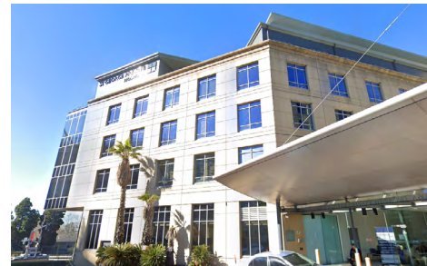
Image 14 St George Private Hospital Complex
