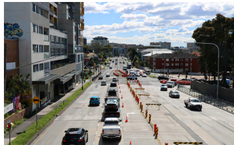
Image 4 Princes Highway Over Bridge Facing North
