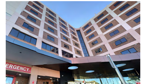
Image 15 St George Public Hospital Complex
