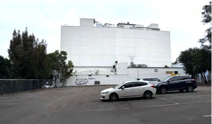
Heavily Modified Landscape - Highway / Carpark
