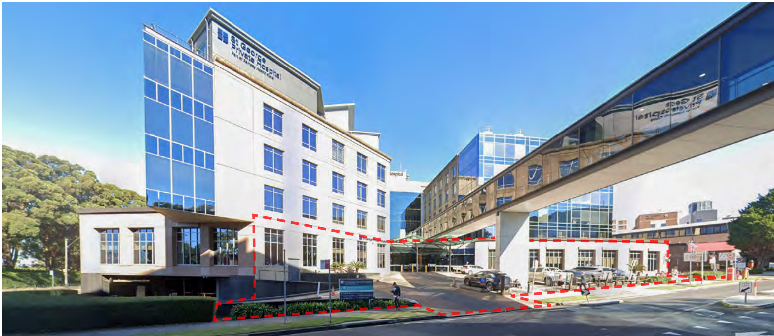
Site A - Existing Entrance and Forecourt to St George Private Hospital
