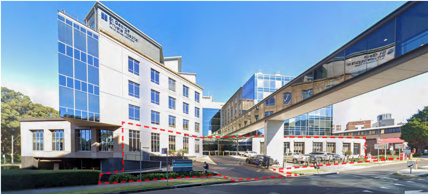
Site A - Existing Entrance and Forecourt to St George Private Hospital
