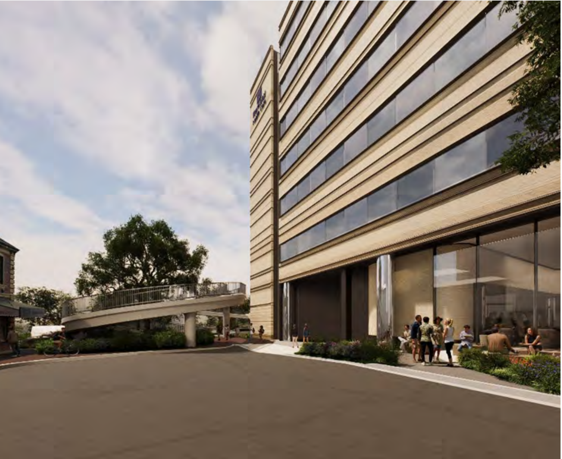
Hogben Street East End Termination Zone
