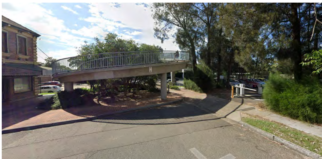
HOGBEN STREET – EXISTING CONDITION STREET TERMINATION AND CARPARK ENTRY
