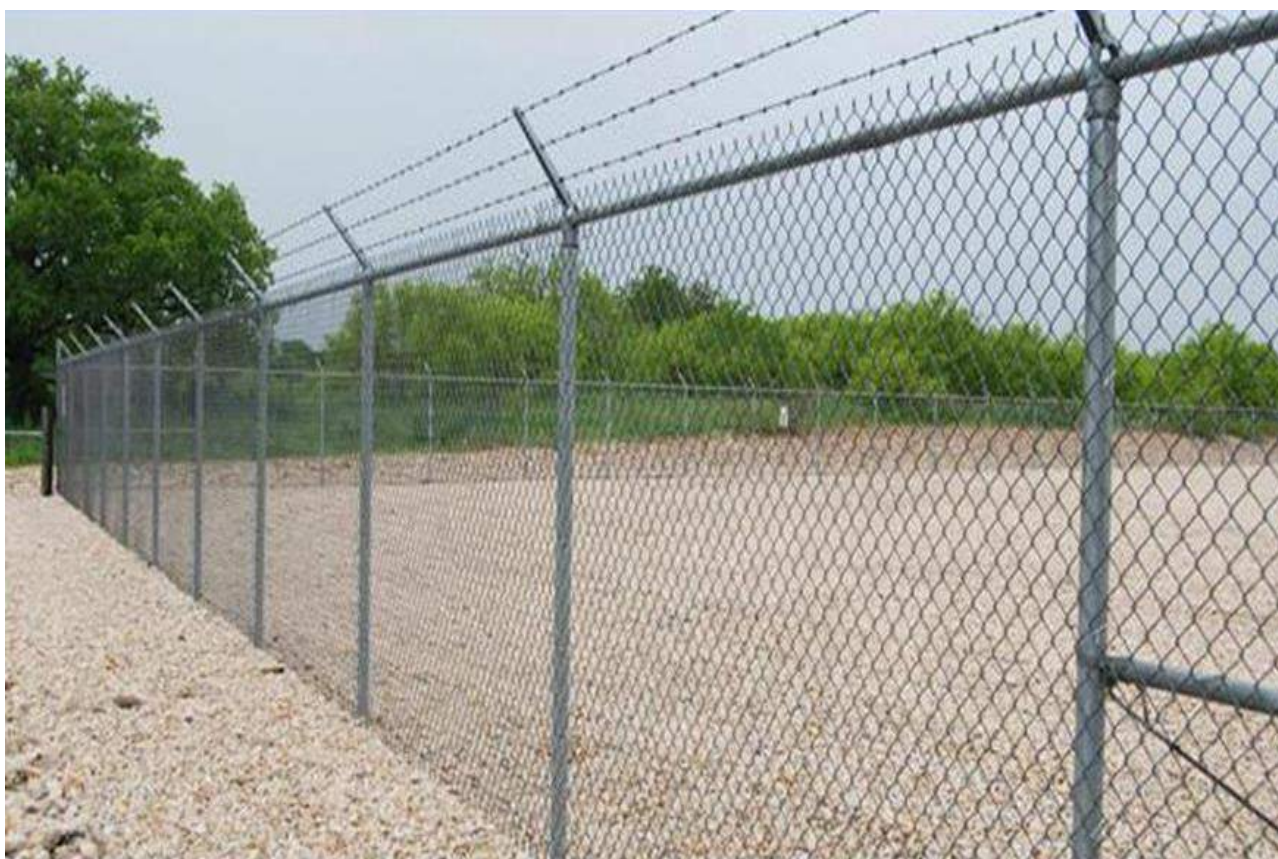
Figure 3-9: Example security fencing (chain link security fence)
