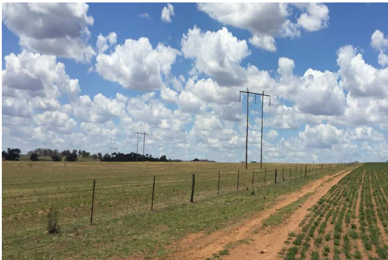
Figure 3-1: Existing electrical infrastructure in the area
