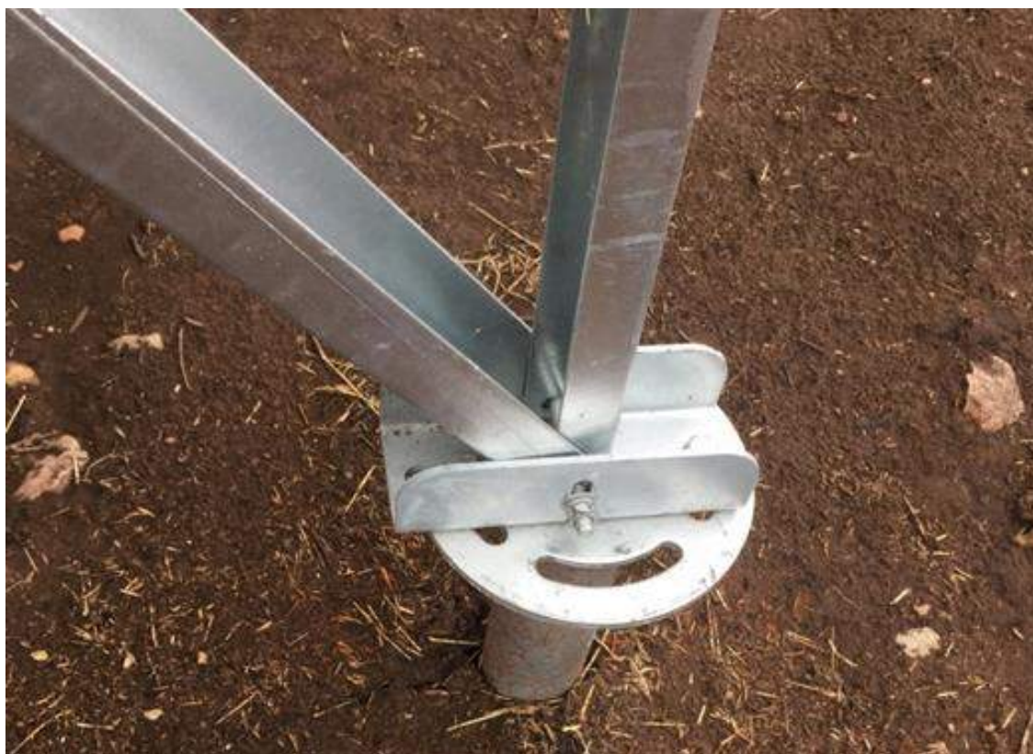
Figure 3-4: Example of ground mounting arrangements
