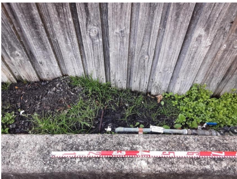
Photo 14 No exposure (0%) in the southern portion of 134 Beecroft Road, facing south-east (scale rod: 1 metre)
