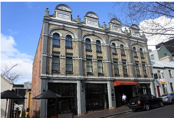
Picture 1 – Front Façade of the Harbour Rocks Hotel
