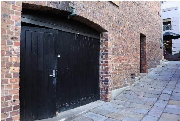
Picture 3 – Existing Northern Façade of the Building
