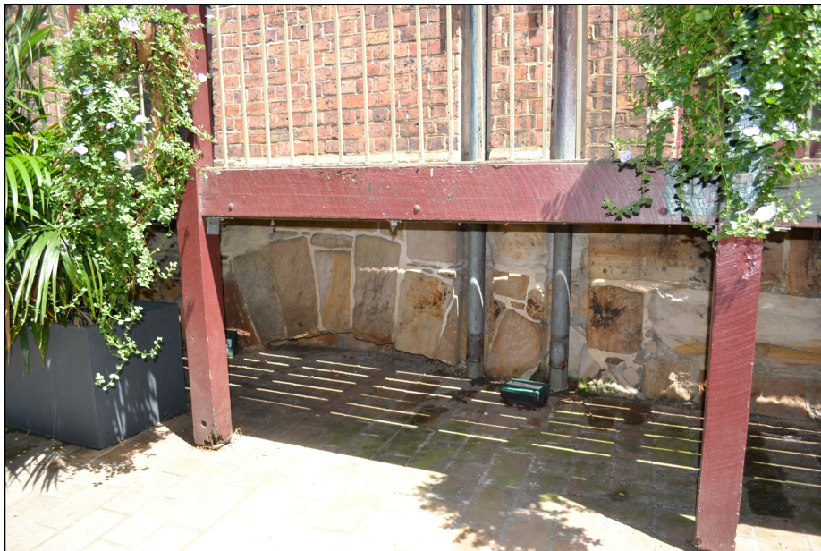
Photograph 4: Showing the rear of the Harbour Rocks Hotel along Nurses Walk. The top of an archway can be seen just above the current footpath surface indicating the building has been cut into the steeply sloping hillside of the study area.
