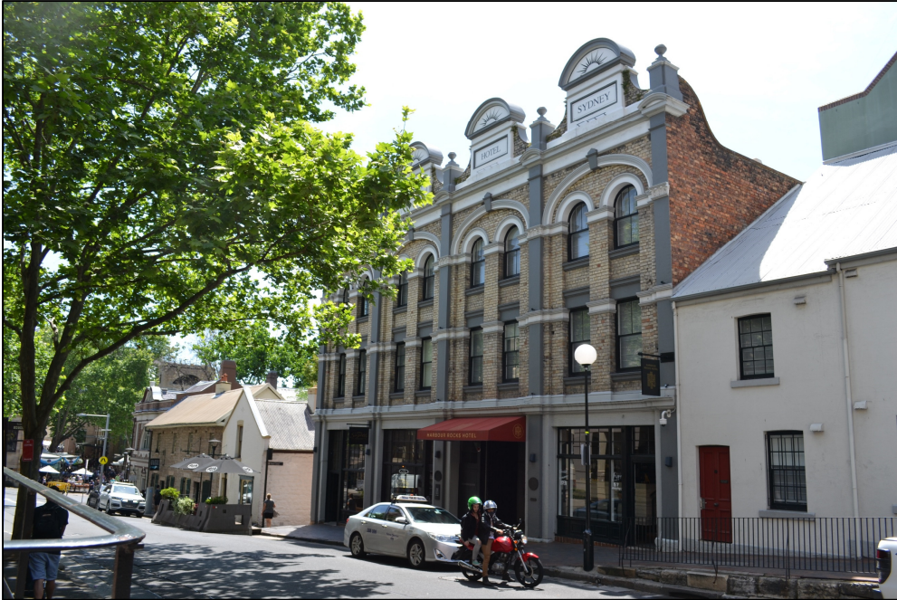
Photograph 1: Showing the Harrington Street frontage of Harbour Rocks Hotel.
