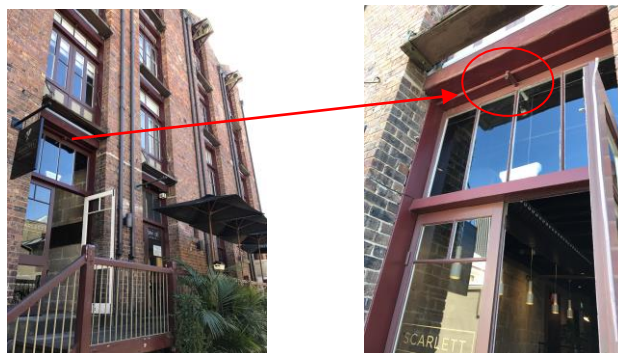
Figure 3: Existing protection to openings in the external wall (Nurses Walk)
