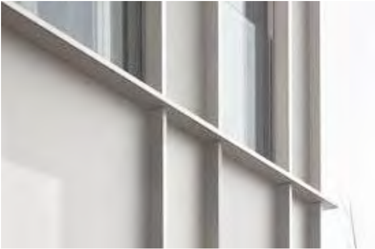
Matte off white metal window wall framing
