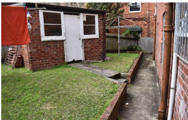
Figure 29 – Brick shed and paved surfaces within rear of 64 Lavender Street.
