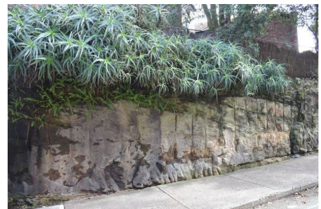
Figure 30 – View from 3 Middlemiss looking towards 5 Middlemiss.
