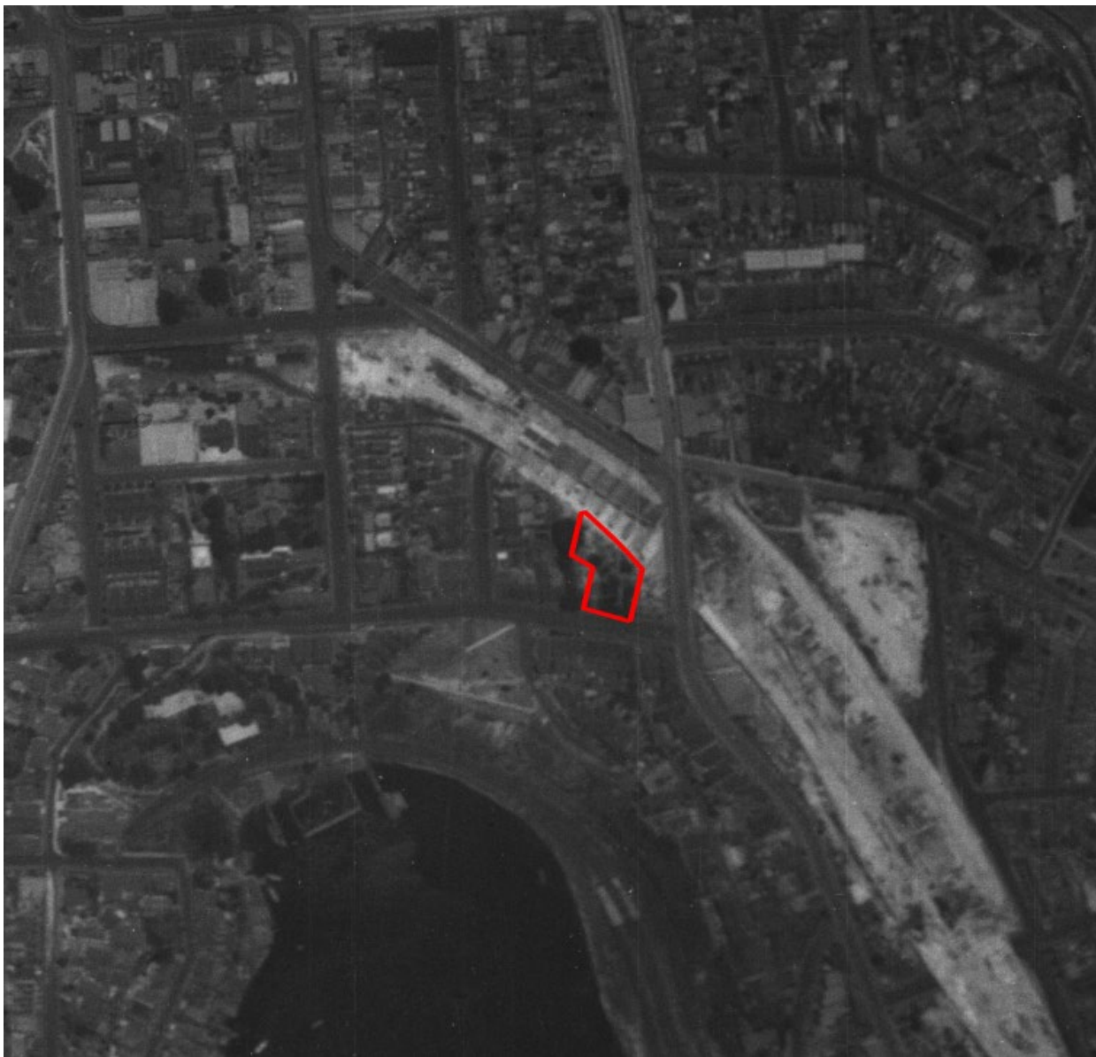
Figure 19- Aerial view of the subject site in 1930, the subject site is approximately indicated in red. Construction activity related to the Sydney Harbour Bridge is evident. No structures are present on the subject site.
