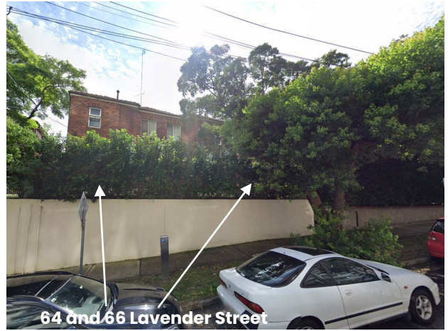
Figure 26 – View of front of 64 and 66 Lavender Street showing boundary wall, facing north-west.
