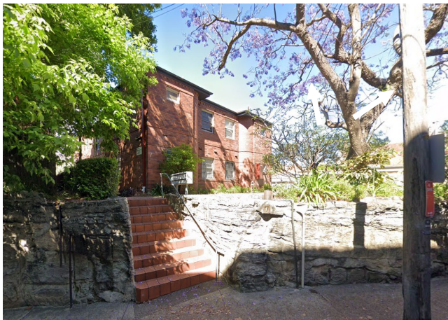
Figure 27 – View of 7 Middlemiss Street showing boundary wall, facing south-west.
