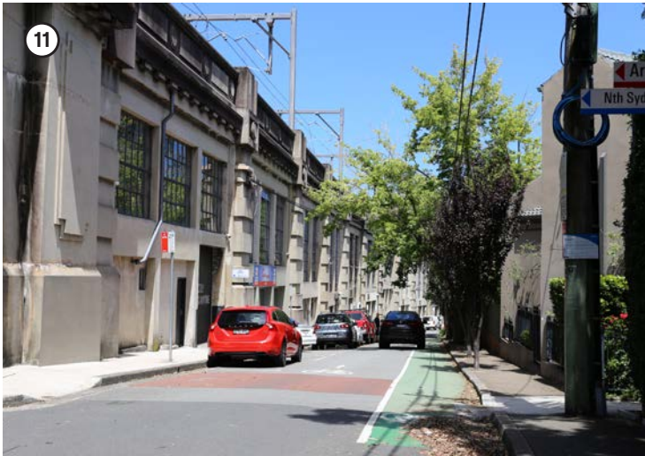
Sydney Harbour Viaduct and on-road cycleway on Middlemiss Street
