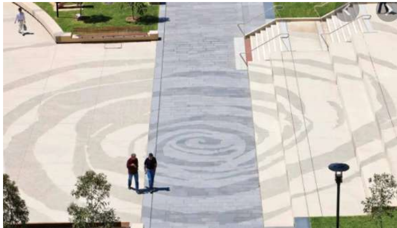
Wingarra-Murra, sandblasted paving design, University of Sydney
