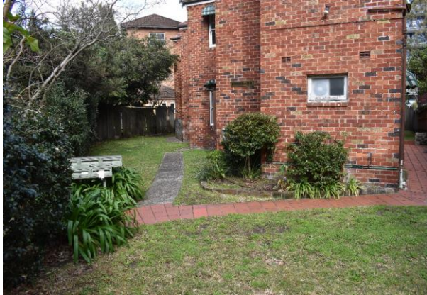
Figure 16: Grassed area complete with pathways and services in boundary of 3 Middlemiss Street
