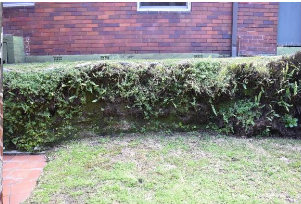
Figure 15: View from 3 Middlemiss looking towards 5 Middlemiss
