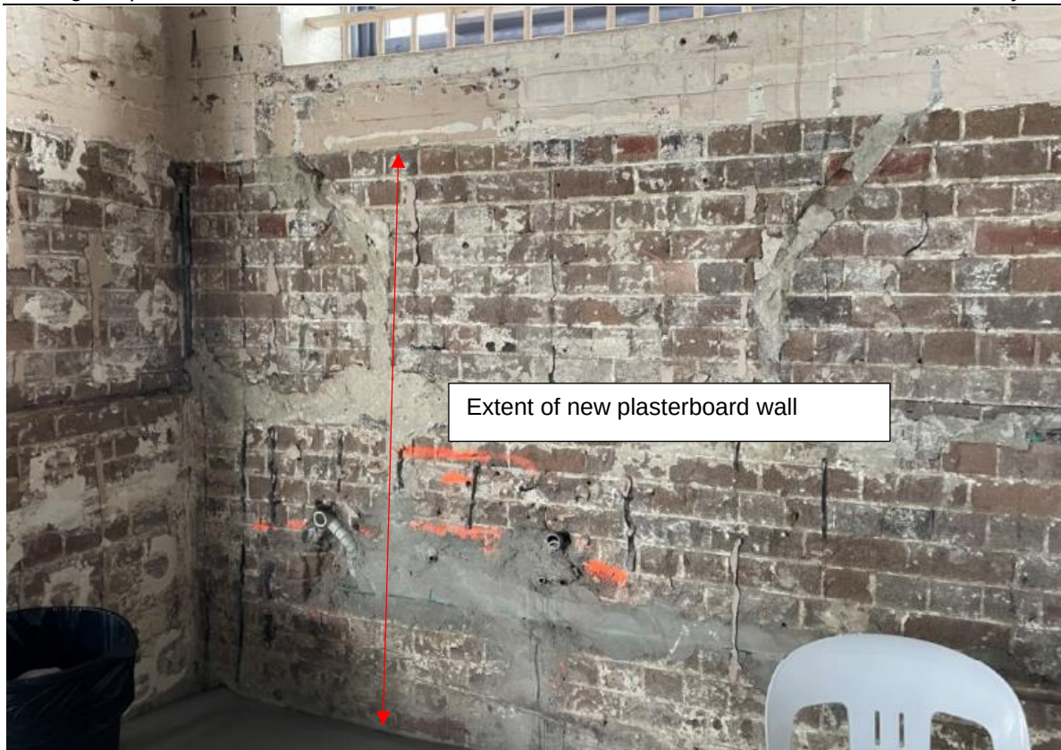
Figure 23: Previous chasing for services and poor cement mortar patching to southern brick wall.
