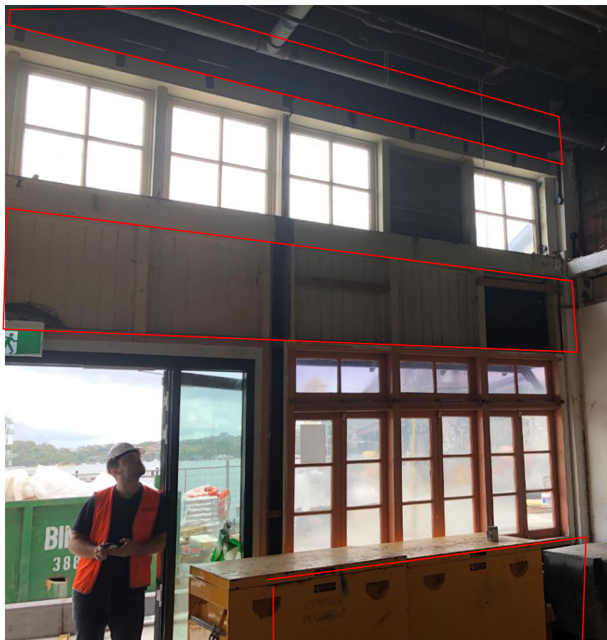
Figure 16: Commercial 2 taken in 2020. Current proposed upgrade includes lightweight wall to areas marked red.
