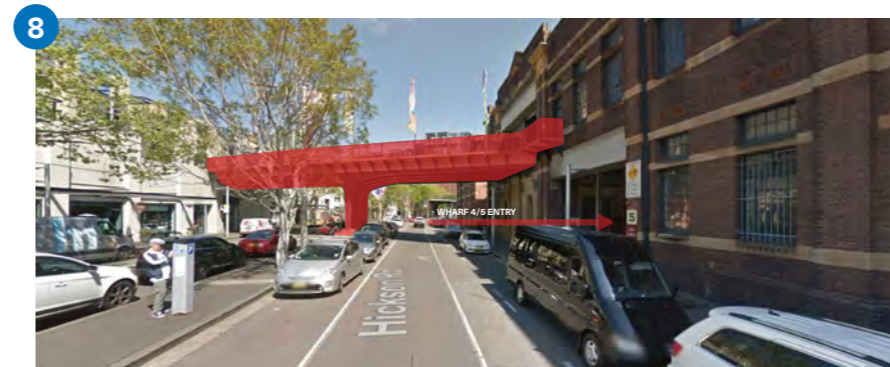
Gateway 8, Wharf 4/5 Viaduct Bridge (East Approach)
