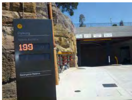
1 Car Park sign with digital counter at Barangaroo Reserve, Towns Place.
