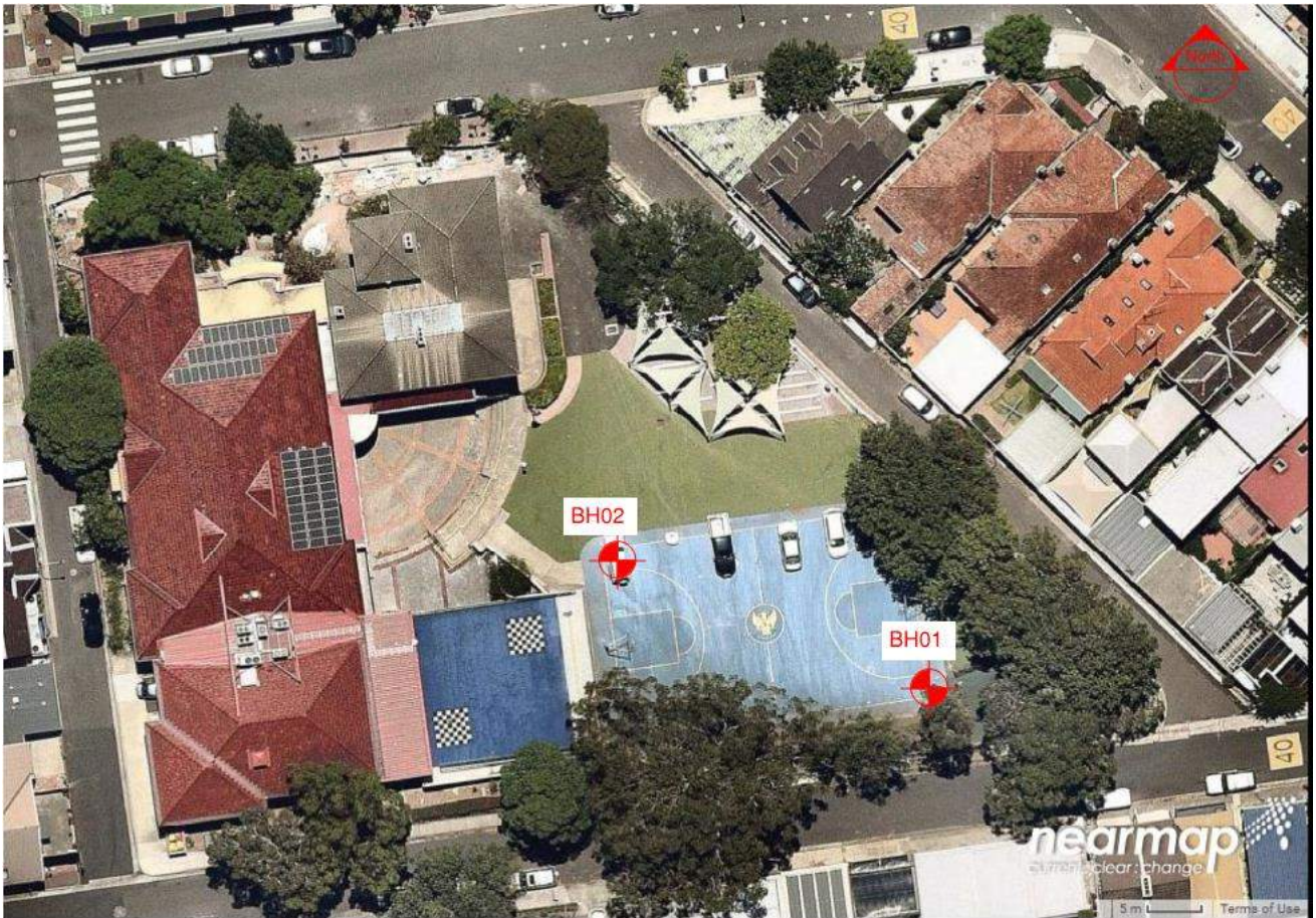
Figure 5 Aerial Image of the Junior School Site and Borehole Locations (Source Nearmap)
