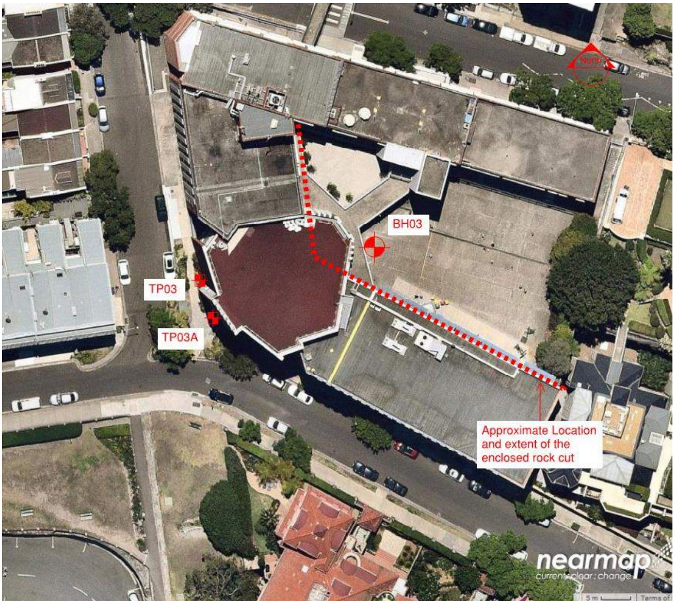
Figure 7 Main Campus Site and Exploratory Locations (Source Nearmap)
