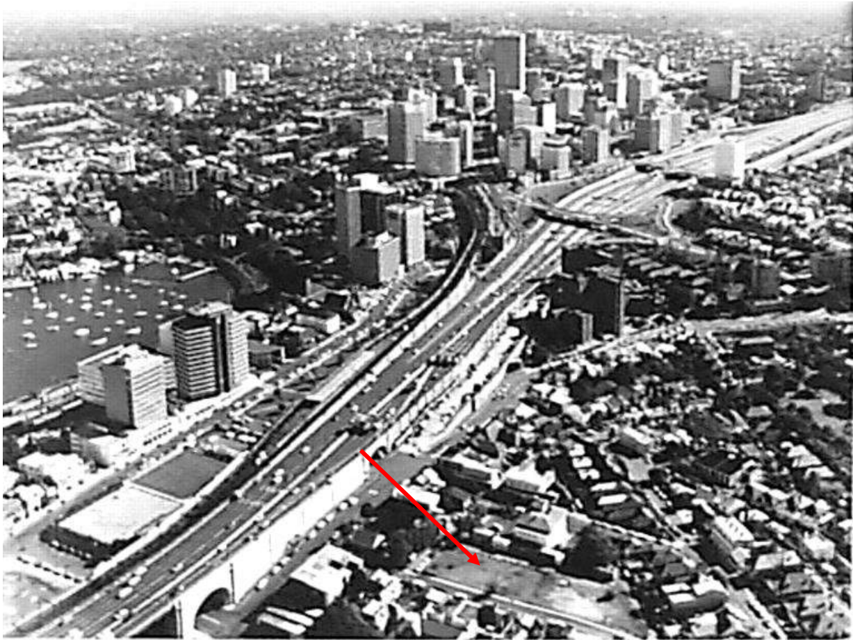
Figure 2.22: Aerial view of Milsons Point 1978. The block of houses fronting Bligh Street, behind Milsons Point Public School has been cleared (arrowed). Stanton Library LH REF PF807.
