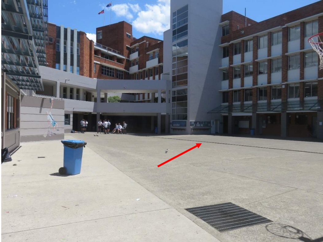
Figure 4.2: View looking southeast in concrete-paved courtyard playground area of Main Campus. Note grated service in foreground and shallow grated agricultural drain (arrowed) across playground area.
