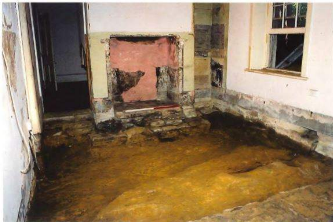
Figure 3.3: View of 63-65 Kirribilli Avenue, Kirribilli interior of Room 3 kitchen showing natural bedrock exposed below excavated deposit. Casey & Lowe 2000, Photo 10.
