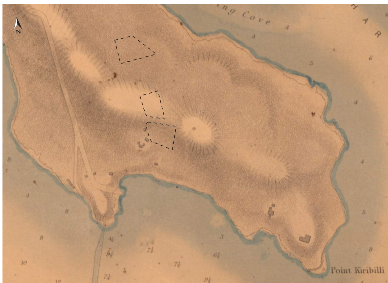
Figure 2.4: Detail from Mitchell's 1853 Trigonometrical Survey of Port Jackson showing approximate location of the three study area blocks in black outline. National Library http://nla.gov.au/nla.obj-231443454 .
