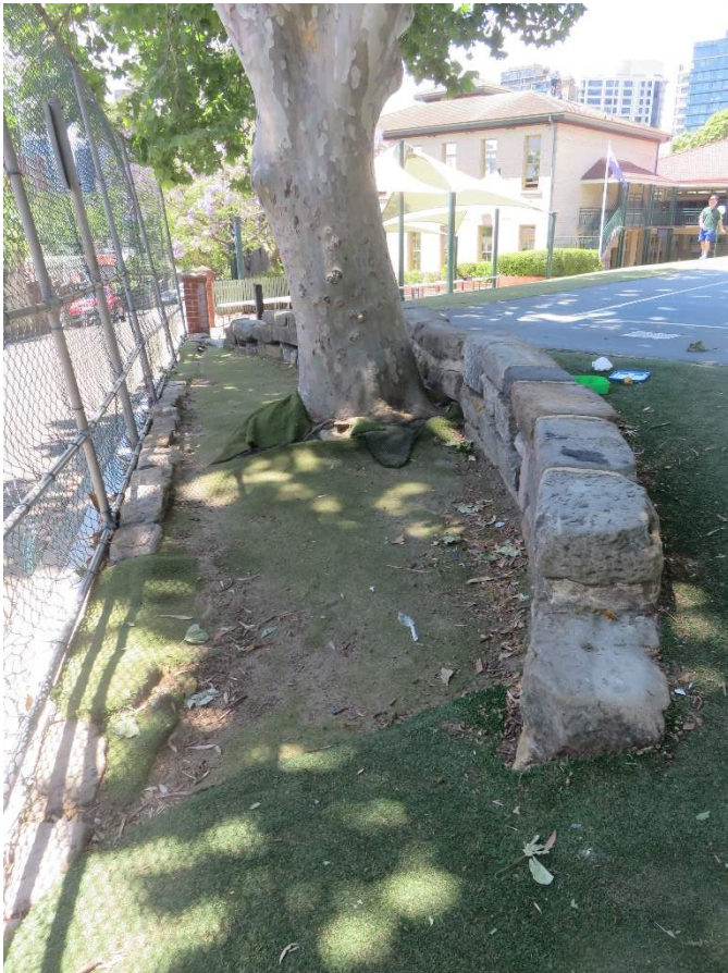
Figure 4.16: Looking west along north study area boundary toward original 1887 school building. Crescent Place on left. Salvaged sandstone blocks in two low lines form the study area boundary retaining 'wall' and a low curved wall behind trees. Some stones are above and others under the astroturf.
