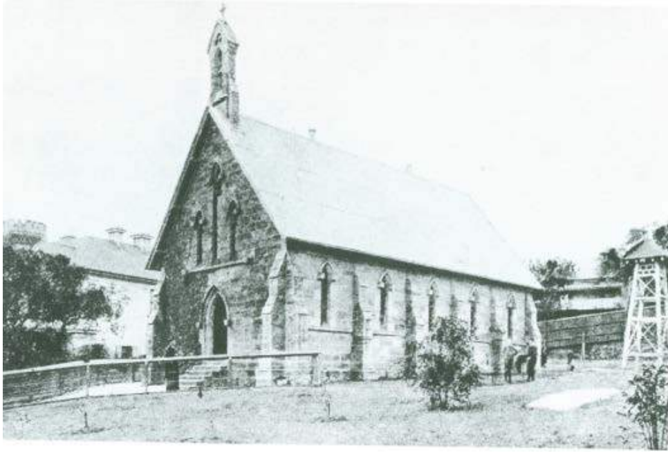
Figure 2.13: 1906 view of the Congregational Church looking northwest. 'Hillside' is visible at left. Strong 1997: 18.
