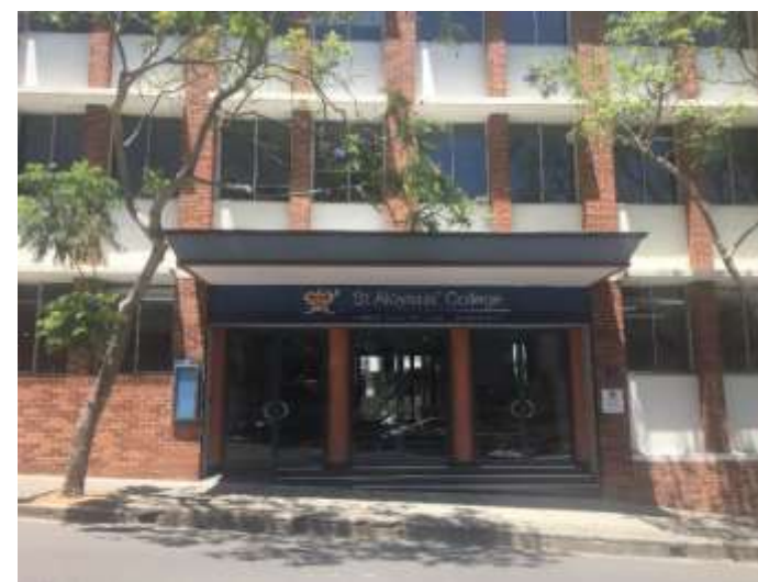
Figure 04 – Existing Principal Pedestrian Entry
