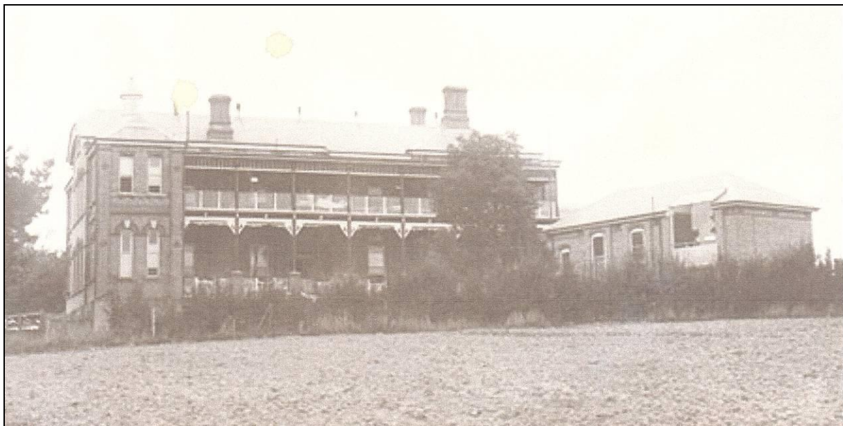
Figure 2.12 Image dated 1922 showing the rear of the 1919 operating room addition (at right). The image also clearly shows the open verandah and balcony added to the eastern facade of the eastern pavilion which was originally constructed with a “T” shaped footprint. (Source: Goulburn & District Historical Society Inc, State Records, 4346_a0202_a020000233)
