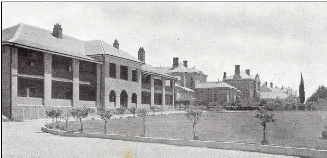
Figure 2.16 Springfield House and Hospital buildings c. 1930s. The northern addition to the eastern pavilion added in c. 1932 is visible (at left). The High School buildings are also in the background. (Source: Goulburn & District Historical Society Inc.)
