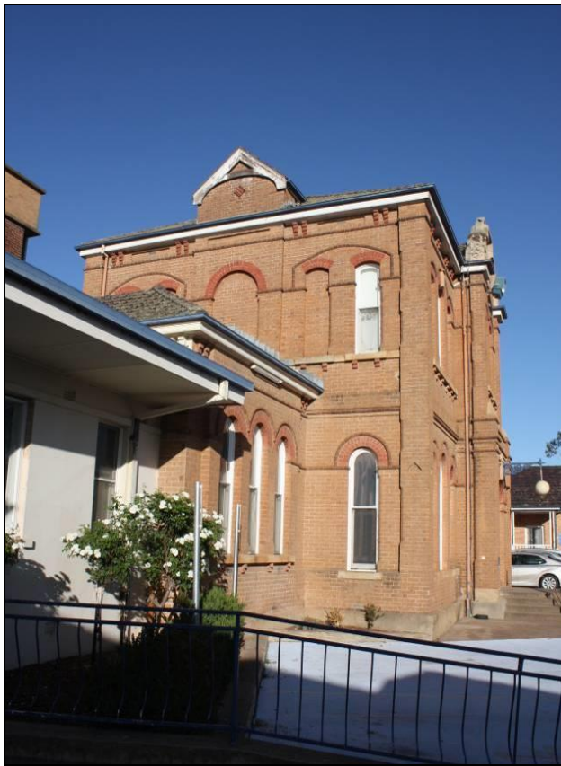
Figure 3.6 One and two storey connections and additions now surround the original pavilions.
