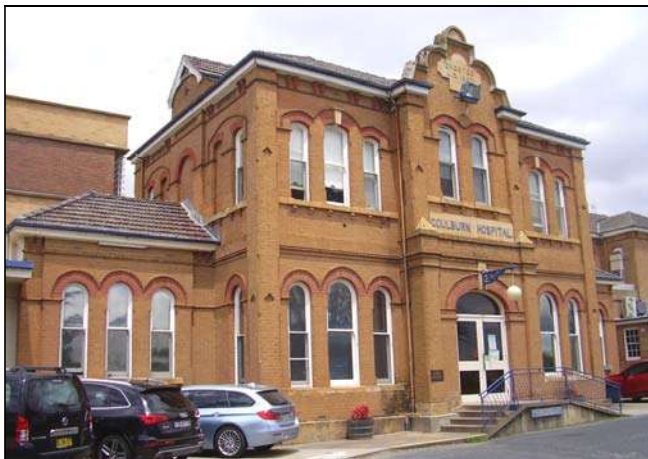
Figure 3.53 In addition to the single storey attached wings and walkways, the roof retains decorative gables. The original chimneys were removed in the c. 1970s when the slate roofing was removed and replaced with tiles.
