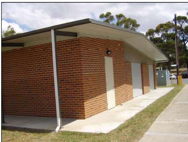
Figure 3.232 The Albert Street façade of the structure which has wide, extended eaves and concrete apron around the building.
