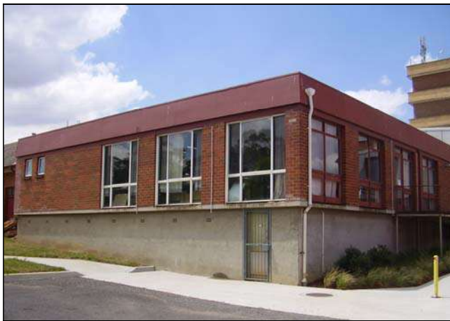
Figure 3.198 The eastern and southern façade of the 1970s addition to the building. A concrete ramp also extends along the north eastern façade.
