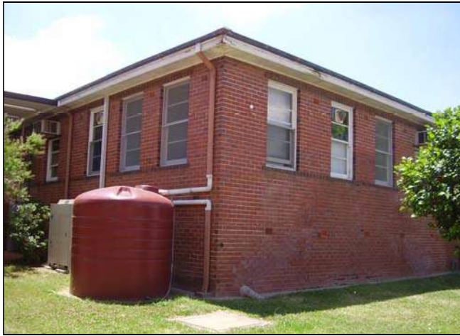
Figure 3.76 The south eastern facades of the former Children's Ward (now Admin and Medical Records) which was added to the eastern pavilion in the early 1940s. The Ward is as simple face brick structure with hipped and flat roof forms clad in tiles and metal sheeting and timber framed windows and doors.
