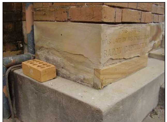
Figure 3.56 A concrete ramp and steps have been added to the original front entry. The foundation stone also remains at the base of the pilaster to the east of the entry. Some fretting and patch repairs are evident.
