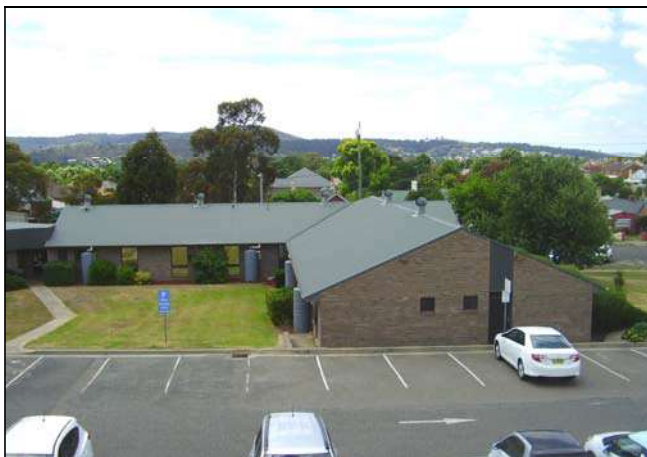
Figure 3.212 The rear of the southern wing of the building which appears to have been constructed after 2005.
