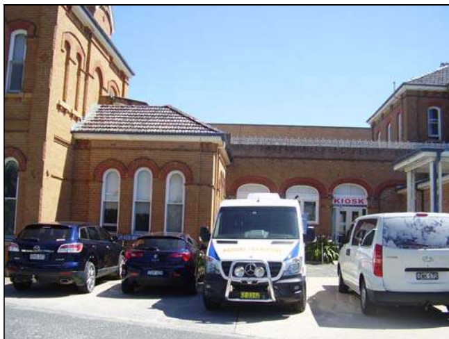
Figure 3.59 The western wing and covered walkway retain arched openings and associated details and cast iron lacework.
