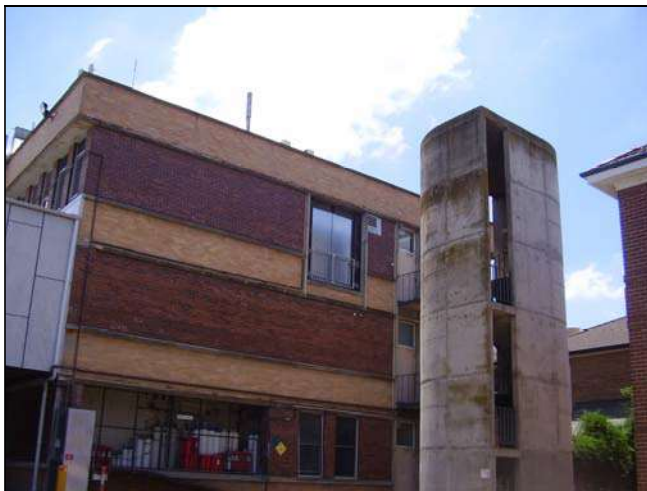
Figure 3.179 The eastern facade and concrete stair of the Theatre wing.
