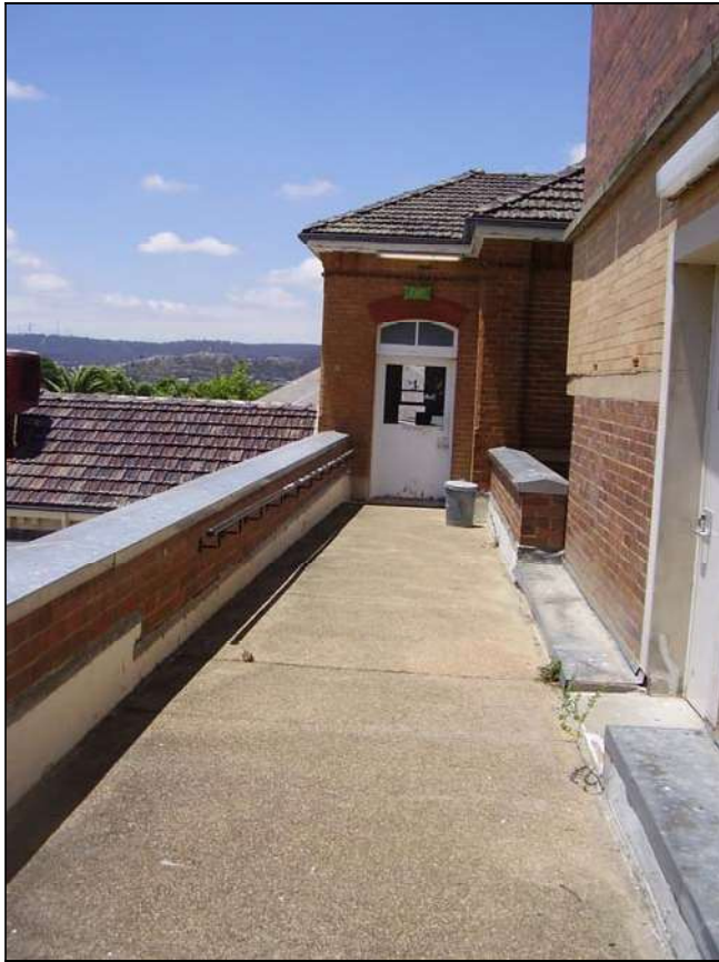
Figure 3.88 The connection and upper walkway between the eastern and central pavilions. The 1960s multi-storey building has been constructed directly to the original connection which has a concrete slab floor and retains the brick balustrade, however, the cast iron rails and detailing visible on the early photographs appears to have been removed.
