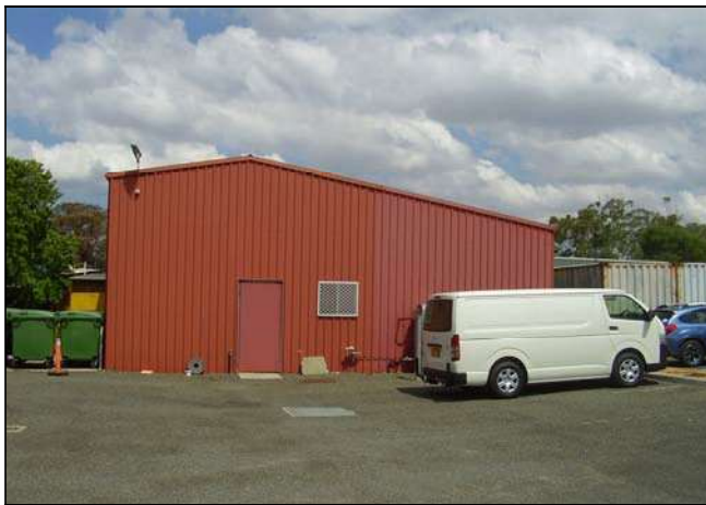
Figure 3.229 The Waste Management Building.
