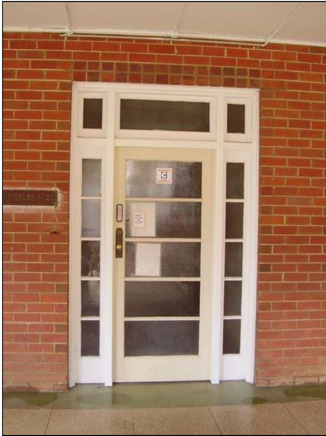
Figure 3.139 The entry door on the ground floor verandah.
