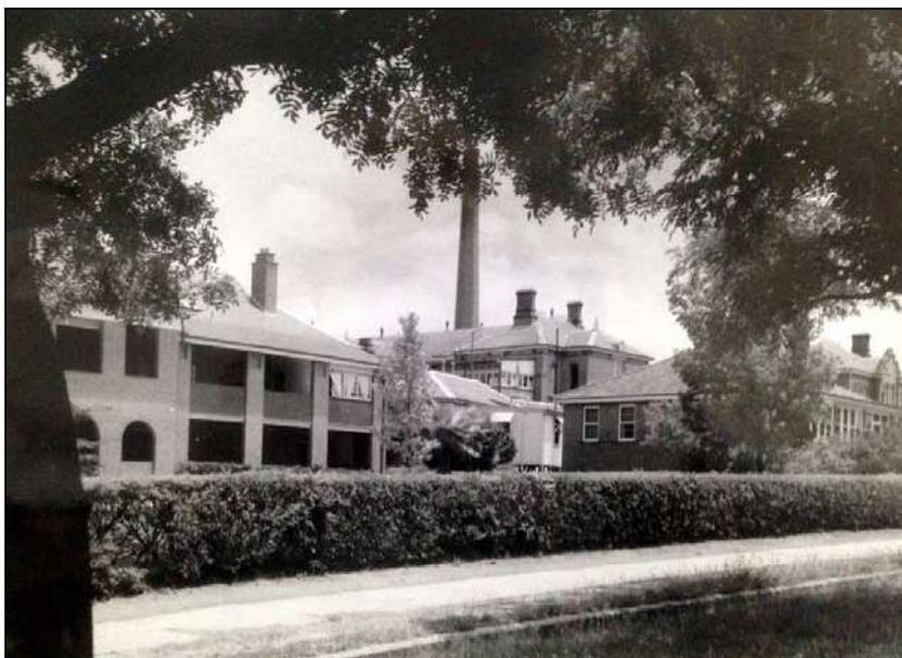
Figure 2.24 Photograph of the c. 1960 showing the Children's Ward constructed at the "front" of the western pavilion, also lightweight additions to the 1919 wing and infill of verandah and balcony spaces. Also note the large brick stack which has since been removed.
