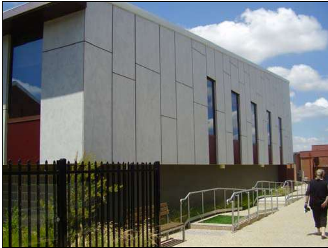
Figure 3.190 The south western façade.
