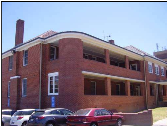
Figure 3.123 Lady Grose Home is a two storey face brick Inter-war period building with hipped and flat roof section clad in tiles and metal sheeting.
