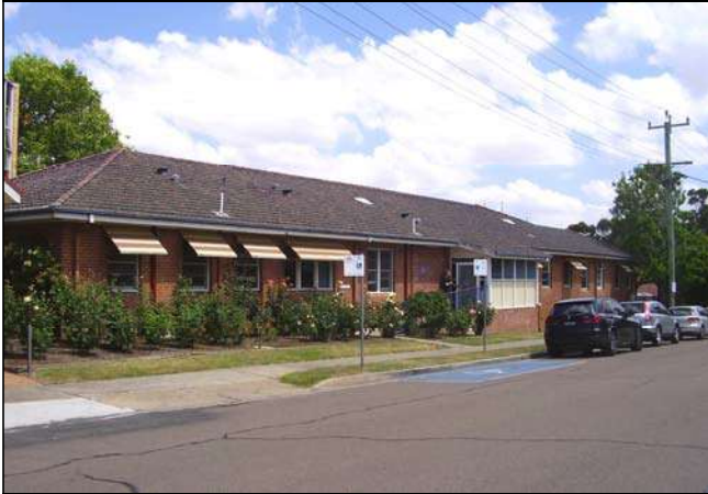
Figure 3.155 The Maternity wing is located close to the Albert Street frontage and is a simple storey face brick building with hipped roof clad in tiles.
