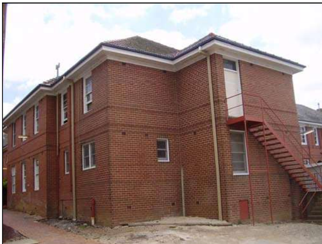
Figure 3.133 An addition three bedrooms, show bathroom and lavatory were added to the south western corner of the building in c. 1955. A steel stair is also located on the southern facade of the addition.
