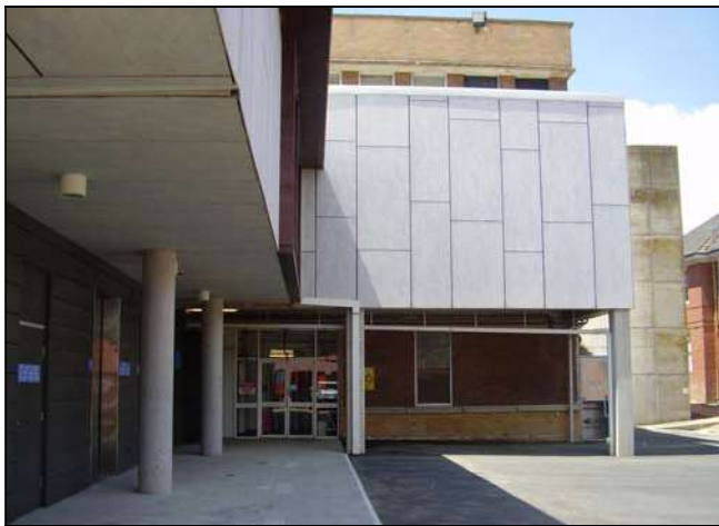
Figure 3.187 The service entry and loading dock area.
