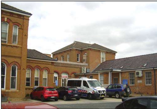
Figure 3.52 The western pavilions and various single storey wings and connecting elements.
