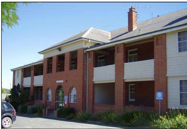
Figure 3.105 The front façade of Springfield House. The main roof changes pitch and extends over the first floor balcony spaces. The ground floor verandahs have solid brick balustrades to the openings and verandahs also have solid balustrades with timber shingled cladding with bellcast detail. Lightweight cladding and aluminium framed windows have been added to enclose the end bays.
