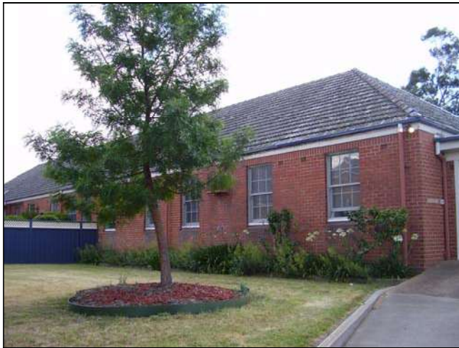
Figure 3.149 The West Wing is located in the north western corner of the site and is a single storey face brick structure with hipped roof clad in tiles and timber framed windows and doors.
