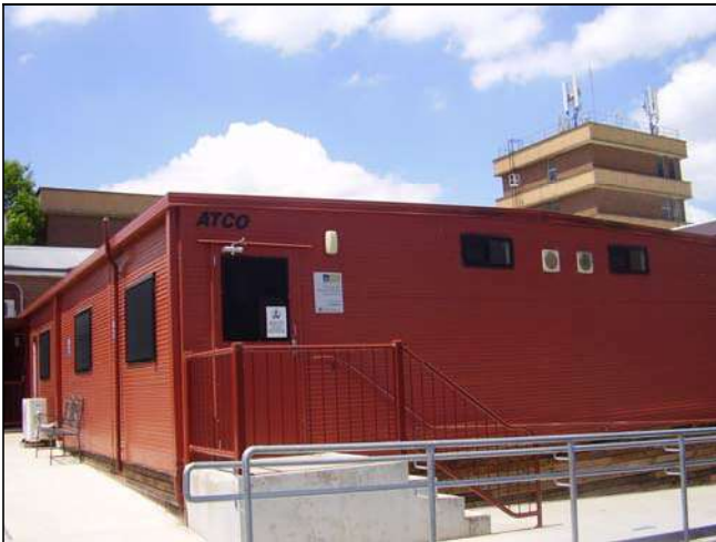
Figure 3.163 A demountable (Uni) building abuts the southern façade of the building.
