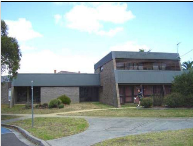
Figure 3.208 The building is a brick and steel structure with architectural form typical of the late 20 th century (c. 1980s).
