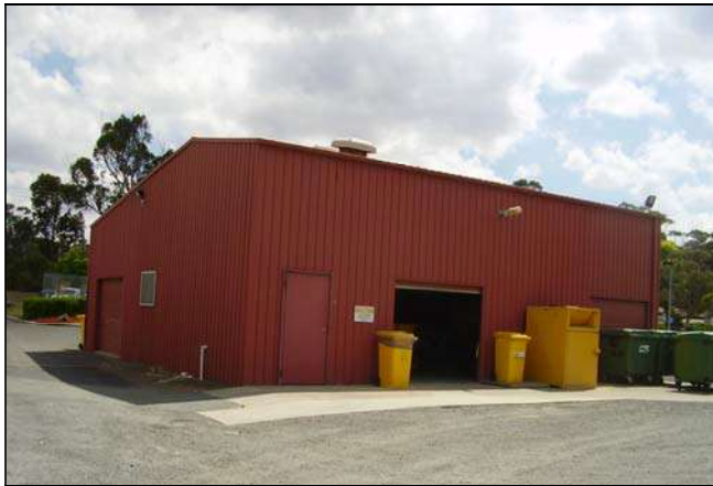
Figure 3.228 The Waste Management Building.
