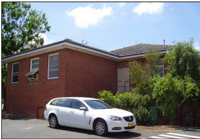
Figure 3.160 The southern façade of the building.
