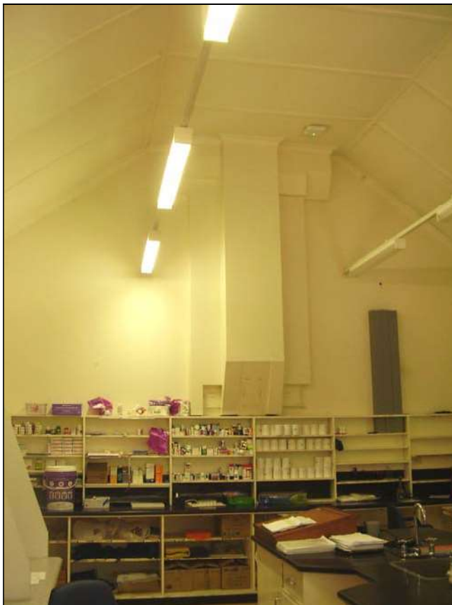
Figure 3.93 The Pharmacy area retains a mix of finishes including some early details including batted raked ceilings and later plasterboard and lighting.
