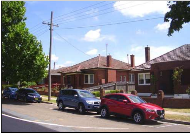
Figure 3.3 Goldsmith Street is largely characterised by single storey detached dwellings mostly dating from the late 19 th early to mid 20 th centuries.
