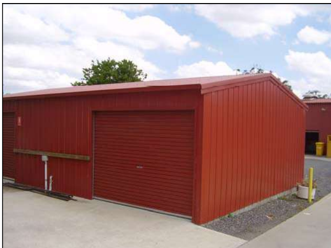
Figure 3.230 One of the other service buildings
