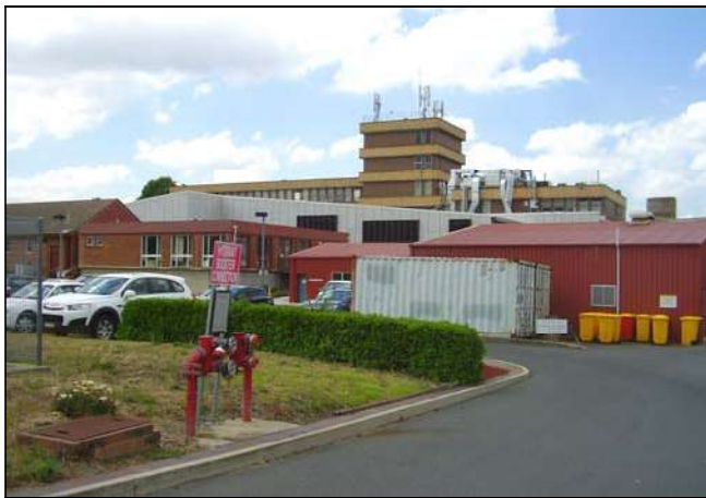
Figure 3.27 A driveways and car park appear to be relatively recent additions to the Clifford Street frontage.
