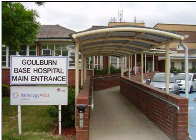
Figure 3.80 A covered concrete access ramp has been added to the western end of the building. The ramp also has a stair and extends from the Goldsmith Street frontage.
