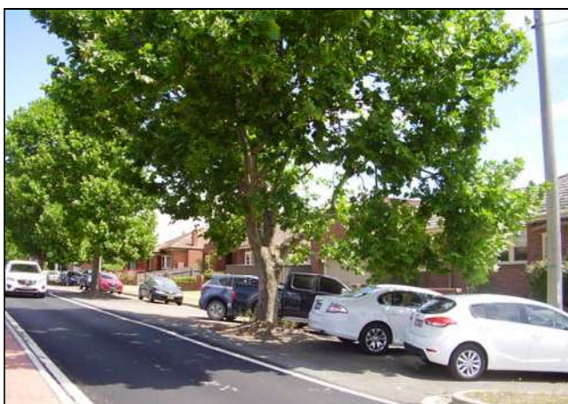
Figure 3.2 The built context is generally enhanced by wide verges and mature street trees.
