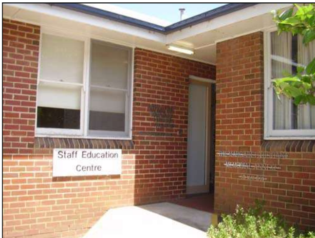
Figure 3.166 The main entry is located at the junction of the two wings of the building. The Zella Fife Memorial Lecture Theatre (1956) which extends in a north south orientation and the southern wing, the Margaret Tustian Memorial Annexe (1959).
