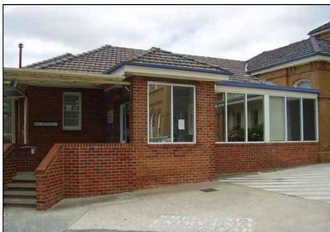
Figure 3.83 Brick and glass infill has been added to the junction between the north eastern single storey wing and former Children's Ward to form the current main entry.
