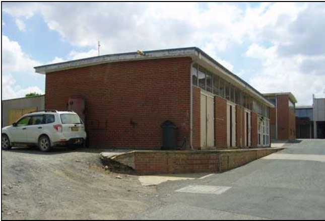
Figure 3.207 The eastern and northern façade of the building which “face” the central service road.
