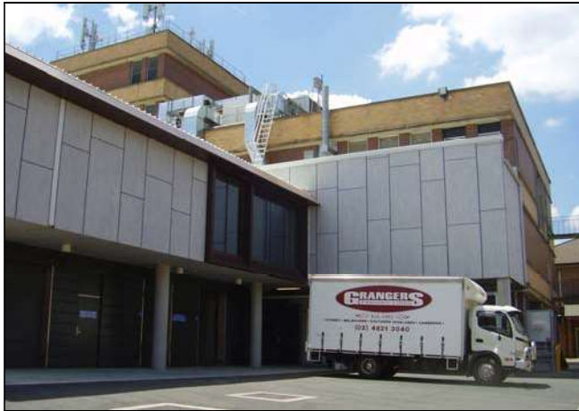
Figure 3.181 A two storey ward and rehab unit has recently (2013) been constructed to the southern facade of the building.
