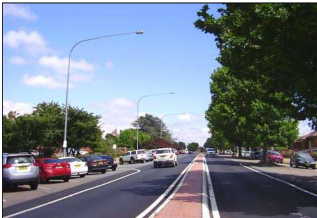
Figure 3.1 Goldsmith Street is a wide dual carriageway with parking on both sides of the street.
