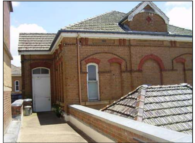
Figure 3.88 The connection and upper walkway between the eastern and central pavilions. The 1960s multi-storey building has been constructed directly to the original connection which has a concrete slab floor and retains the brick balustrade, however, the cast iron rails and detailing visible on the early photographs appears to have been removed.
