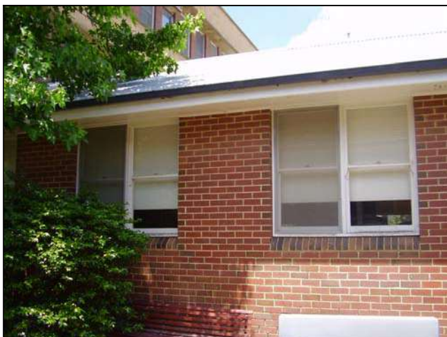
Figure 3.167 The north western facade.
