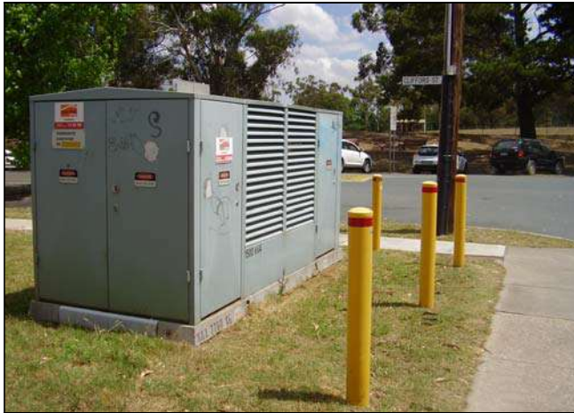
Figure 3.234 A substation is located close to the building and street corner.
