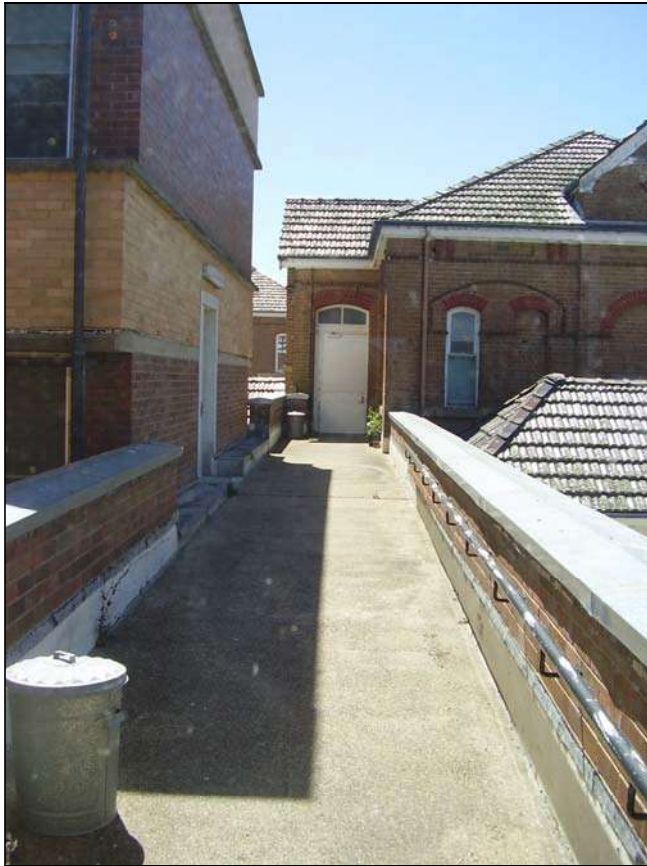
Figure 3.174 The elevated walkway and connection to the northern wing of the 1960s building.
