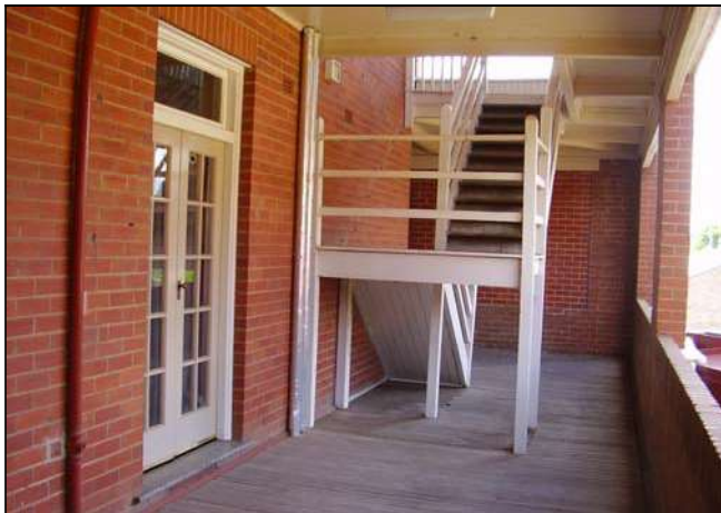
Figure 3.112 A timber stair located at the south eastern corner of the rear verandah provided external access to the upper balcony.
