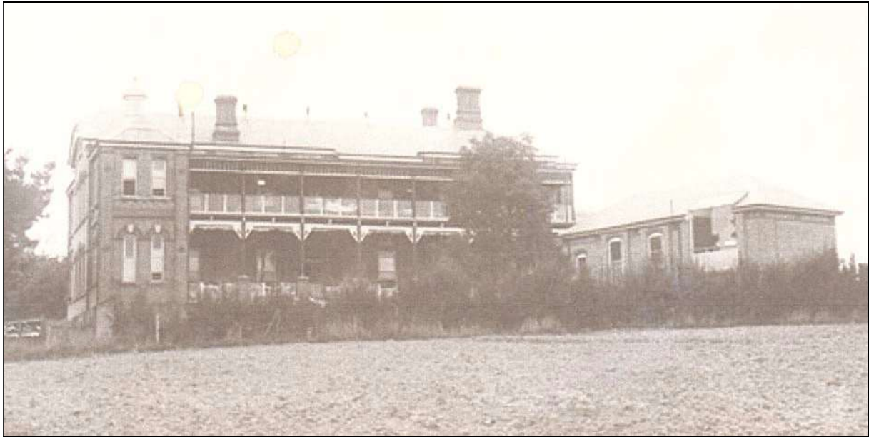
Figure 2.16 Image dated 1922 showing the rear of the 1919 operating room addition (at right). The image also clearly shows the open verandah and balcony added to the eastern facade of the eastern pavilion which was originally constructed with a “T” shaped footprint. (Source: Goulburn & District Historical Society Inc, State Records, 4346_a0202_a020000233)
