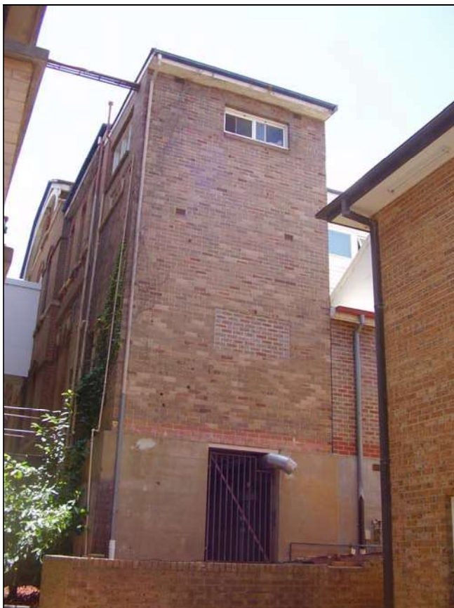
Figure 3.72 A brick addition has been added to the south eastern projection of the eastern pavilion.
