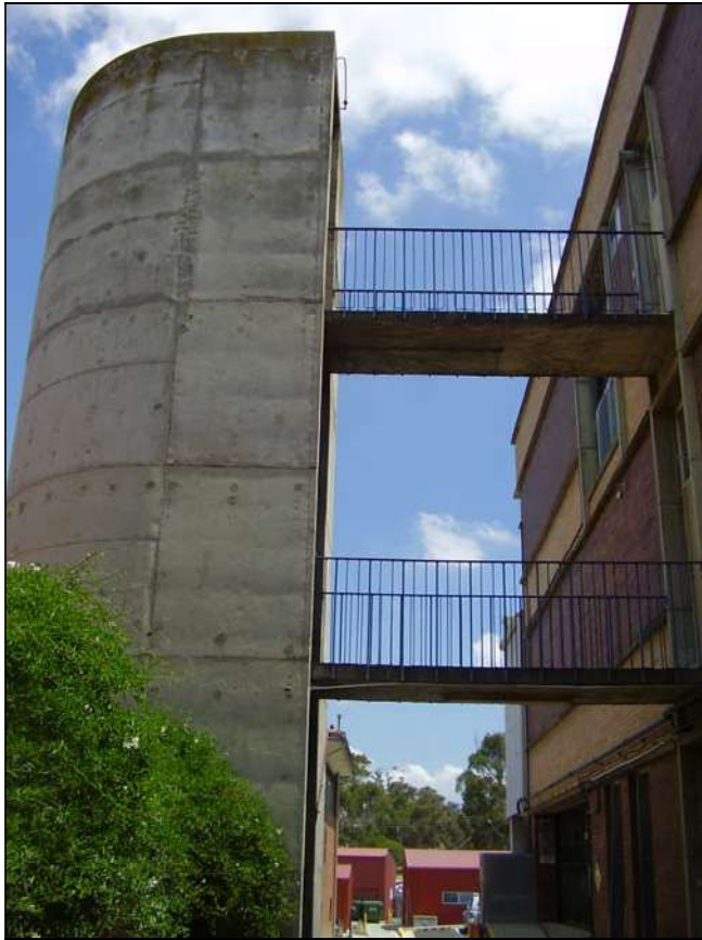
Figure 3.178 A concrete stair is attached to the eastern, Theatre wing of the building.
