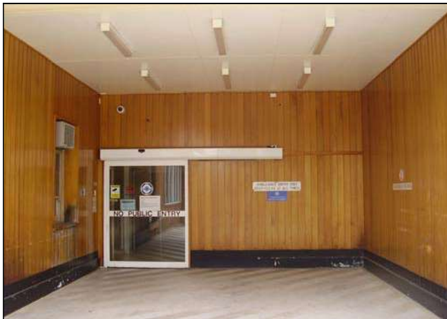
Figure 3.86 The ambulance bay which is simply finished.
