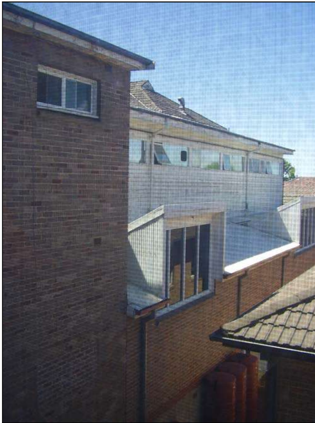
Figure 3.73 A two storey verandah and balcony were added to the eastern façade of the eastern pavilion in c. 1915. The ground floor verandah has been extended out with new brick walls, roof and skylight added. The upper balcony was infilled by the 1930s and has also been upgraded since.
