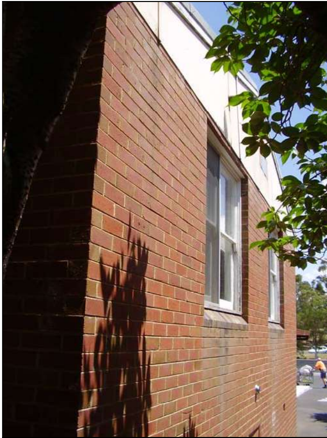
Figure 3.165 The south western façade of the southern wing which has a battened sheet finish to the gable end.
