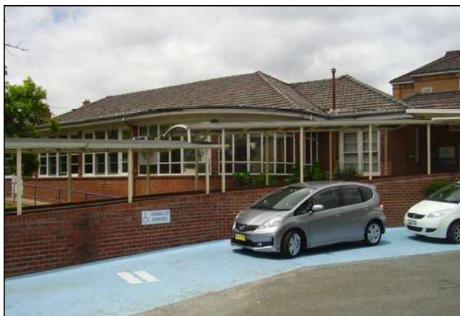
Figure 3.82 The former Children's Ward, now Admin and Medical Records and main entry to the Hospital.
