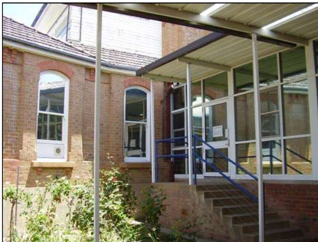
Figure 3.74 The construction of the 1919 operating theatre (splayed wing) also necessitated some alterations this section of the building and verandah and balcony additions. Brick and concrete steps, glazed wall and light weight cover have also since been added to the junction between the north eastern single storey wing and 1919 addition.
