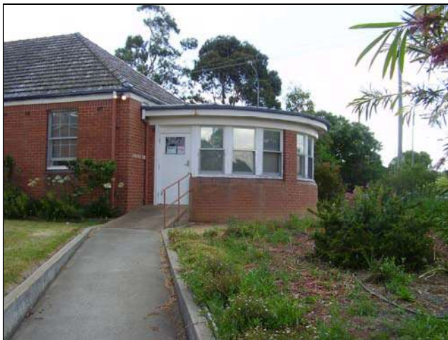
Figure 3.150 The northern end of the building features a curved end bay with flat roof over clad in metal sheeting and timber framed windows and doors. Constructed as a sitting room it is surrounded by planted garden and also overlooks Goldsmith Street.
