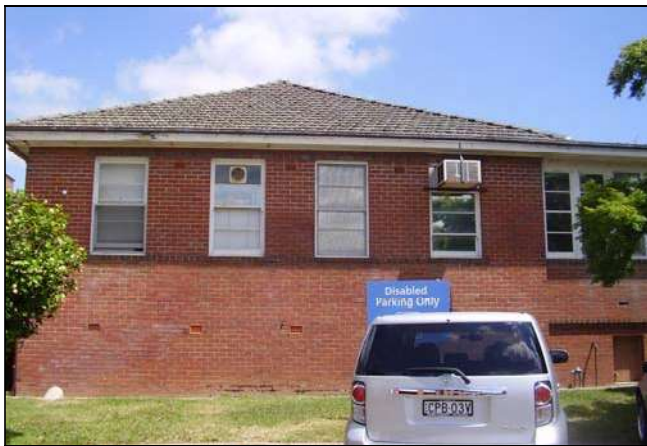
Figure 3.77 The eastern façade of the former Children's Ward (now Admin and Medical Records).
