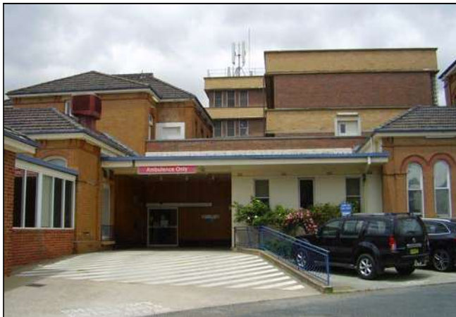
Figure 3.85 The ambulance bay is located adjacent to an infill addition added in the c. 1940s to provide a kiosk. The kiosk was relocated to its present position in the c. 1970s.
