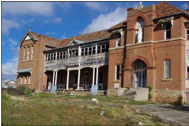
Figure 4.8 St John's Orphanage which was constructed in 1912. The facility also underwent some alterations and additions and closed in 1975. The building is now privately owned and has been affected by a fire.
