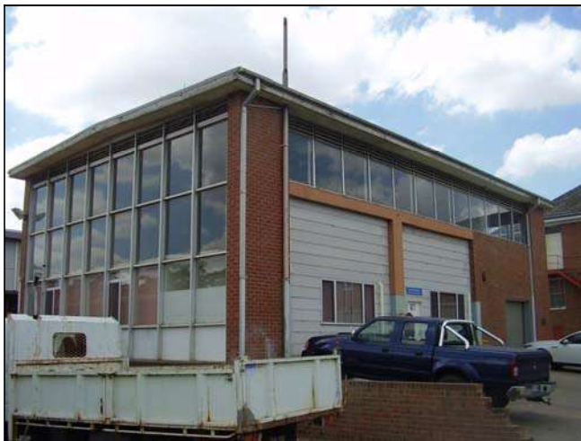
Figure 3.202 The southern façade of the building is fully glazed.
