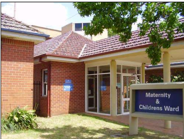
Figure 3.157 The canopy and attached wing are a later addition to the building and site. Other modifications include the aluminium framed doors and signage.
