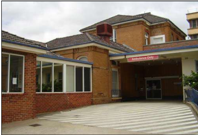
Figure 3.84 An ambulance bay with flat metal deck roof over and concrete ramp extending from the curved driveway has also been added to the front of the building.
