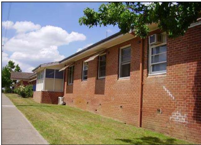
Figure 3.159 The south western façade.
