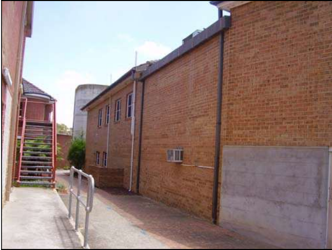
Figure 3.101 The 1989 addition is also constructed of face brick with flat and simple hipped roof clad in concrete tiles.
