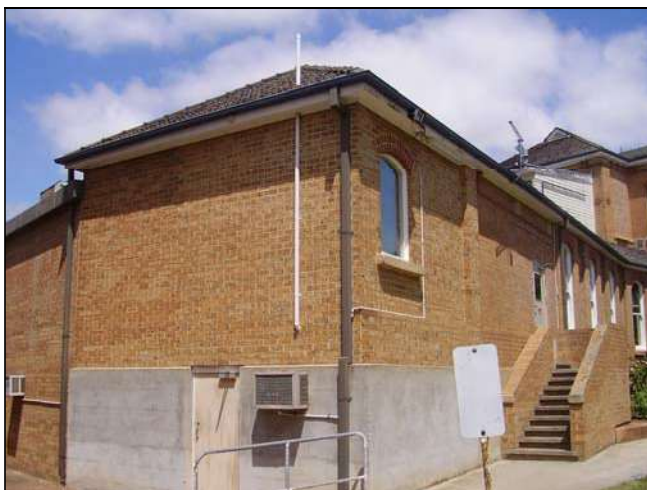
Figure 3.100 The wing was extended in c. 1989 with new Pathology section also added to its south. A simple concrete and brick stair also appears to have been added to the northern façade of the wing.
