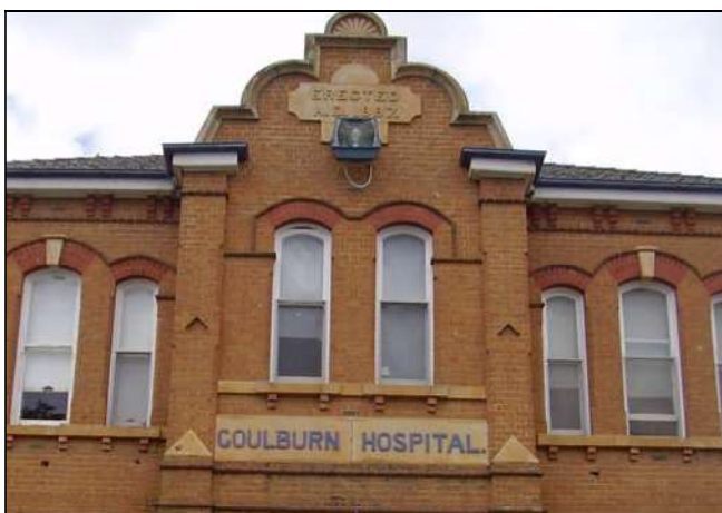
Figure 3.54 Detail of the central front bay and parapet which retains original stone capping and details.
