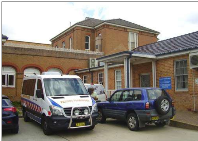
Figure 3.58 The two storey western pavilion and attached wings and connection also retain their overall form and details.
