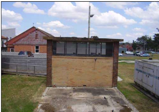
Figure 3.236 The former substation.
