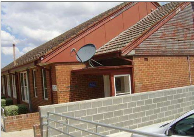
Figure 3.194 The entry to the Renal Unit and 1950s part of the building has a flat roof porch supported by a simple column.
