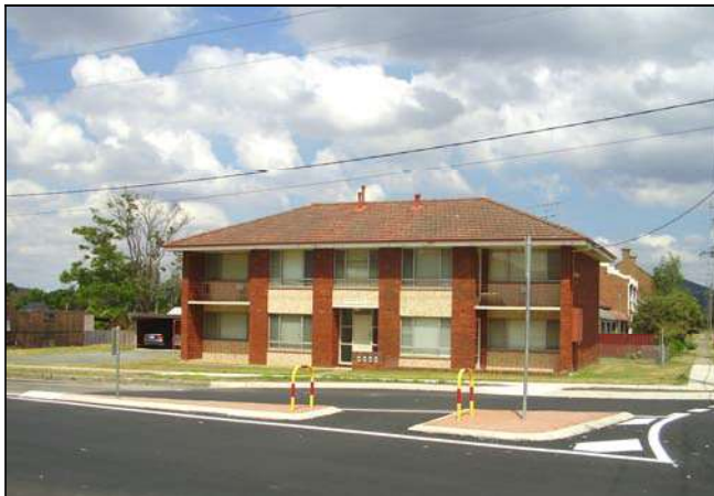
Figure 3.12 Some later, infill residential development is also located in the area.
