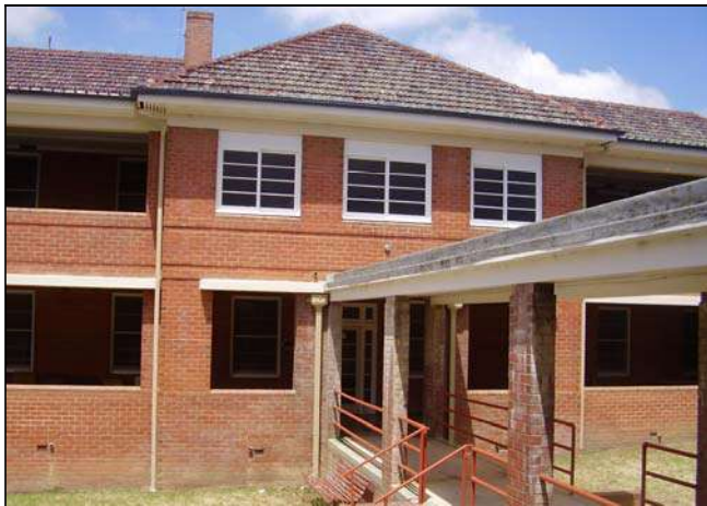
Figure 3.127 The main entry corresponds to the location of the covered walkway connecting the two Nurses’ Homes.
