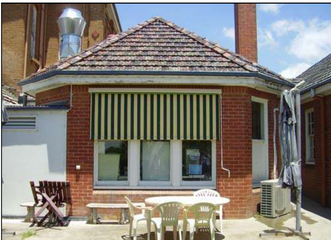
Figure 3.64 The existing kiosk was relocated to a small single storey addition that was constructed as a patient's sitting room in the 1930s. The structure is also face brick with splayed corners, hipped roof and large timber framed windows. A small courtyard bounded by a timber fence and planting surrounds the structure.
