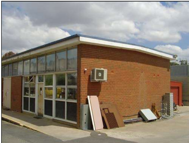
Figure 3.205 A concrete apron and sealed areas extends around the front and western side of the building.
