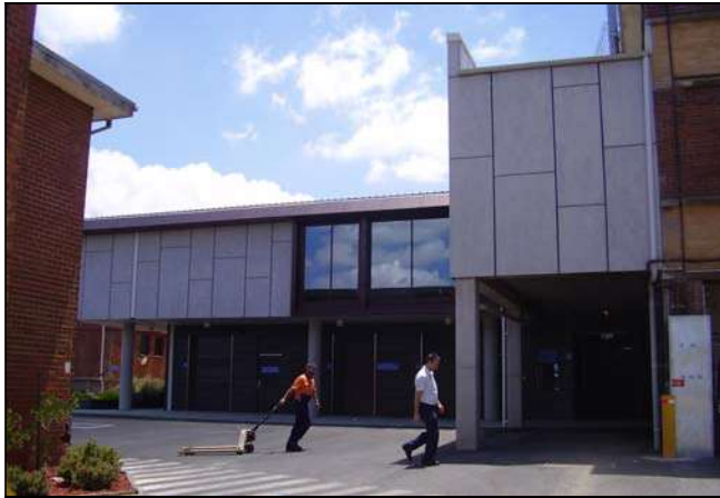
Figure 3.186 The eastern facade of the building which faces the service/ access road.
