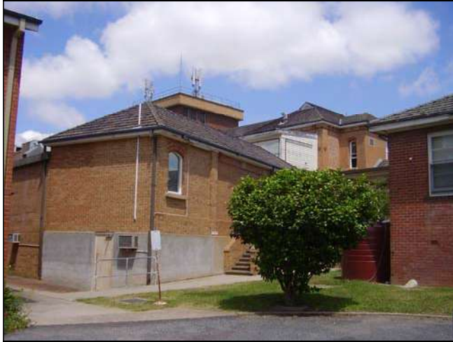
Figure 3.98 The 1919 wing located behind the former Children's Ward now Admin and Medical Records, between the eastern pavilion and Springfield House.
