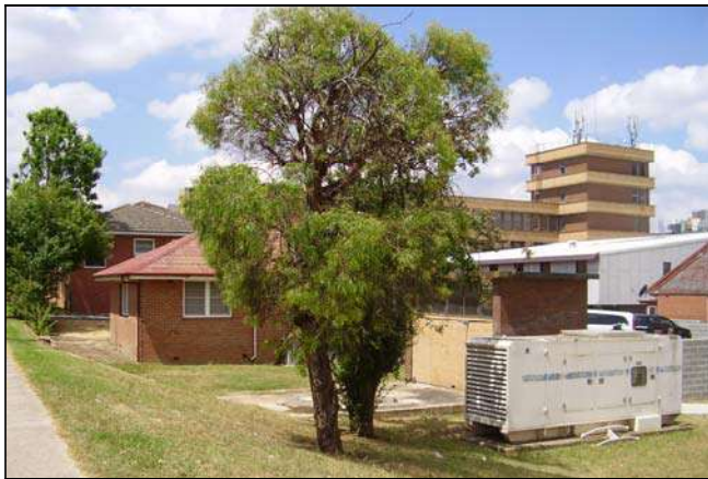
Figure 3.235 The former substation and other slabs and service elements located to the north of the Power and Generator Room and south of the Antenatal Clinic.
