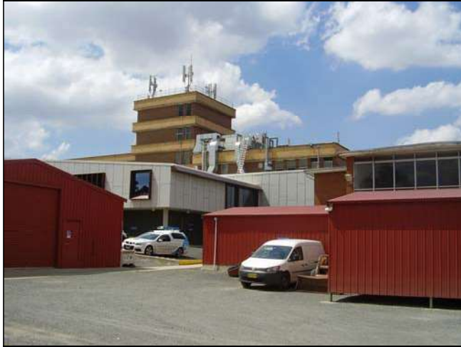
Figure 3.224 The Biomedical Engineering and Waste Management Building are part of a group of simple steel structures located to the south east of the main Hospital buildings.
