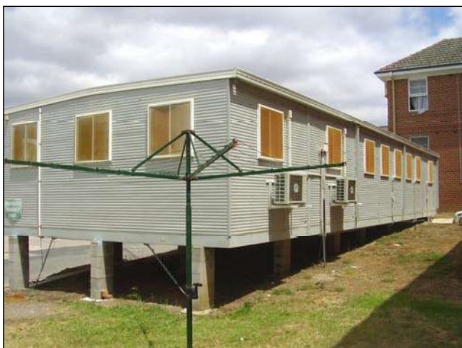
Figure 3.240 The north and eastern façades of the demountable which is mounted on concrete block piers.
