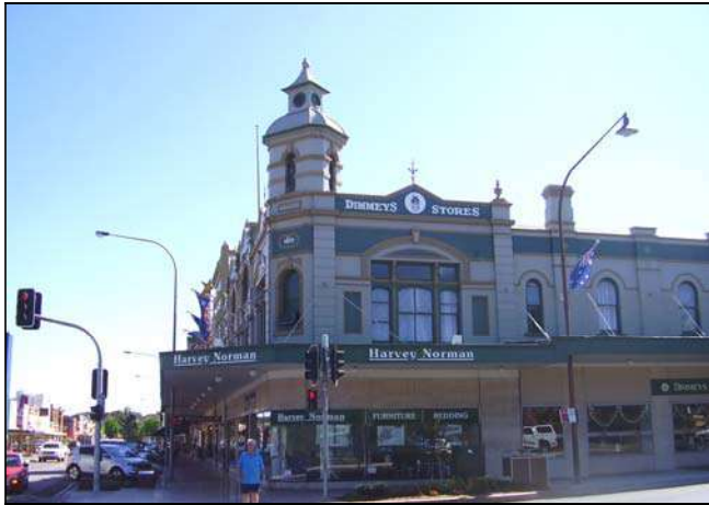
Figure 4.3 Dimmey's Store front and tower located on the corner of Auburn and Montague Streets designed by Manfred and constructed in 1887.
