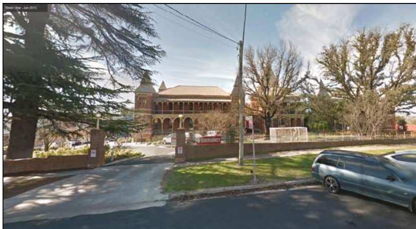
Figure 4.11 Bathurst Base Hospital.
