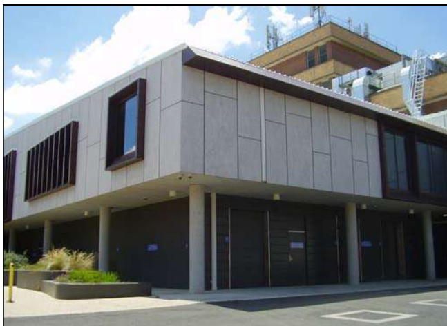
Figure 3.188 The south eastern corner of the building.
