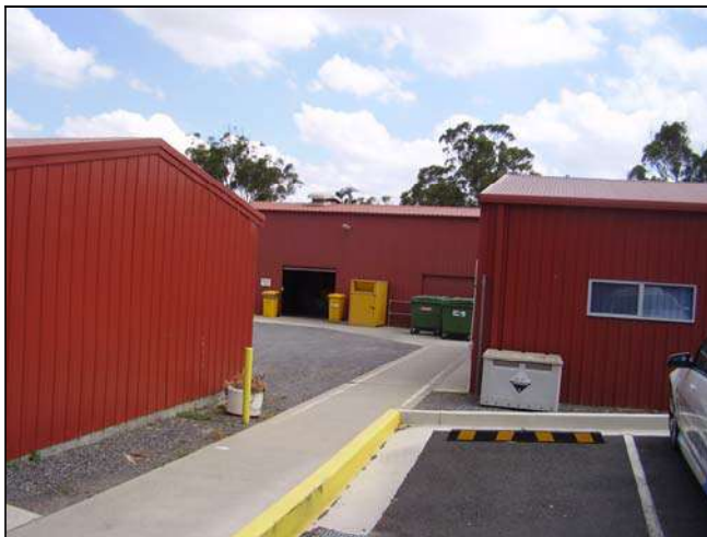
Figure 3.225 The group are accessed by two service roads and are surrounded by sealed area.
