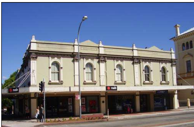
Figure 4.2 The Auburn Street façade of the Mechanics’ Institute on the corner of Montague and Auburn Streets.
