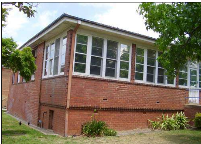
Figure 3.78 The front façade of the former Children's Ward (now Admin and Medical Records) retains typical details from 1940s.
