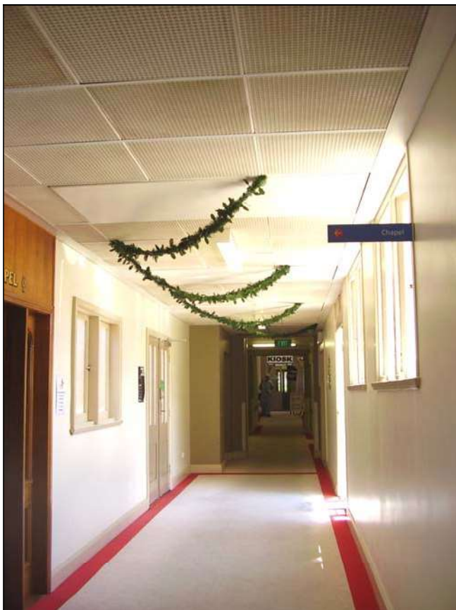
Figure 3.91 The ground floor corridor extending to the western pavilion has been modernised and has vinyl floor finish, minimal timber details and suspended tiled ceiling and modern lighting and services.
