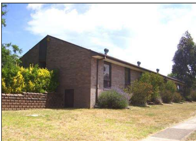
Figure 3.213 The southern wing faces and open setback along the Faithfull Street frontage.
