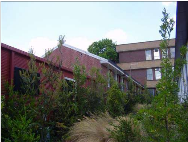
Figure 3.162 The building is a simple single storey face brick structure located in the western section of the site and to the west of the multi-storey 1960s building.
