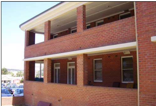
Figure 3.126 The The verandahs and balconies have solid brick balustrade and brick piers and are accessed by timber framed French doors.
