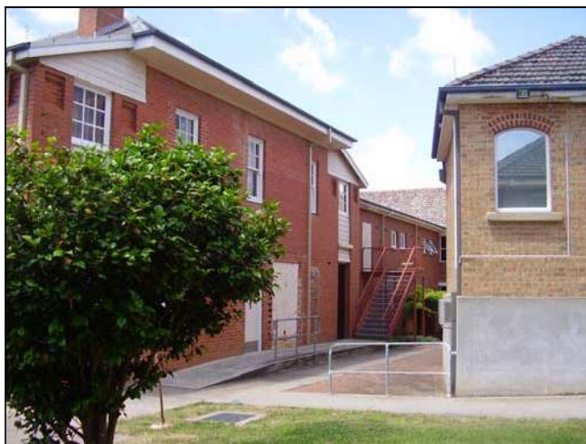
Figure 3.109 Springfield House is detached and setback from the main Hospital building and additions.
