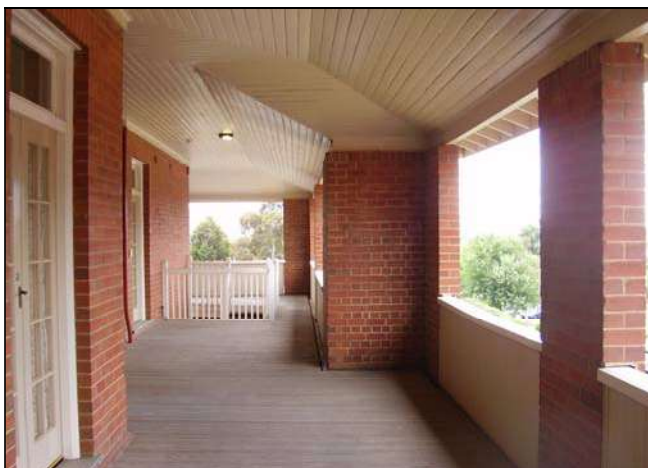
Figure 3.113 The southern balcony. The balconies also retain timber boarded ceiling/soffit.
