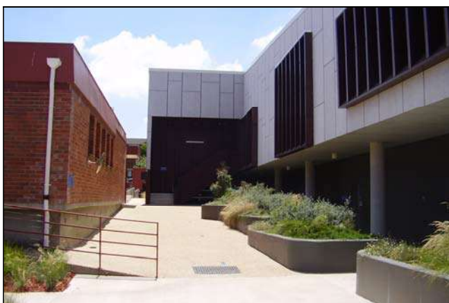
Figure 3.189 New paths and landscapes elements have been added around the building and particularly to the south.
