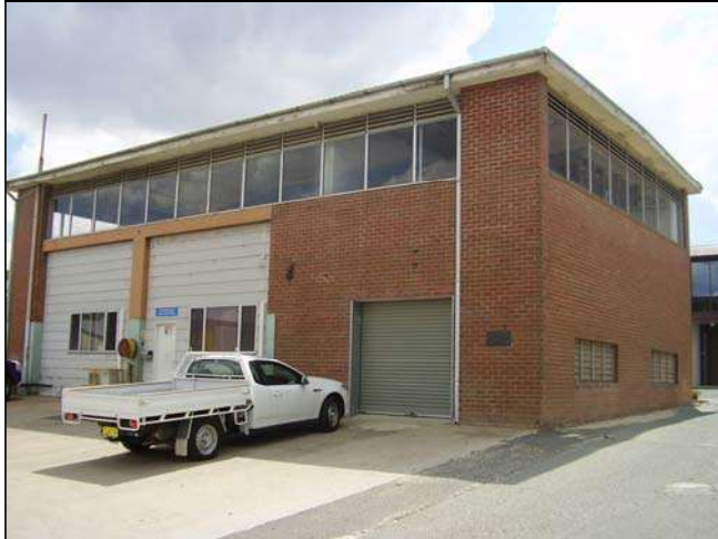
Figure 3.201 The “front” façade of the building faces east and has lightweight infill and a roller door opening at ground level. Aluminium framed windows and louvres extend along most of the upper facades.
