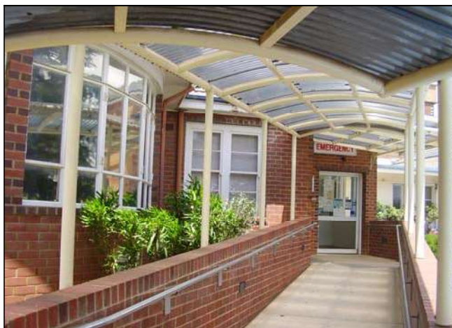
Figure 3.81 The former Children's Ward (now Admin and Medical Records) retains the curved corner detail ("solarium") and openings.
