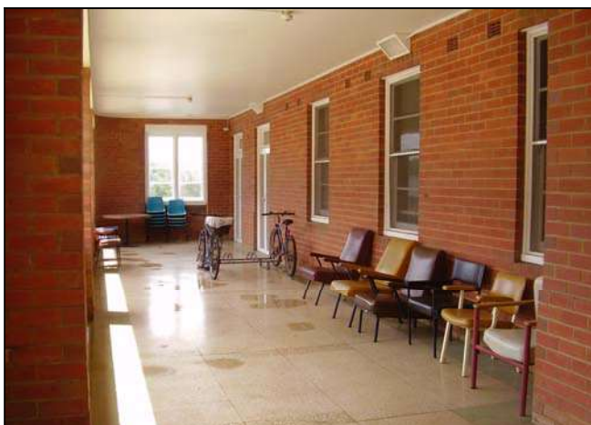
Figure 3.138 The ground floor verandah space which retains terrazzo floor finish, timber framed windows and doors.
