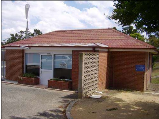
Figure 3.168 The Antenatal Clinic is a small face brick building located close to the Albert Street frontage. The building has hipped roof clad in pressed metal and metals sheeting with rolled joints.
