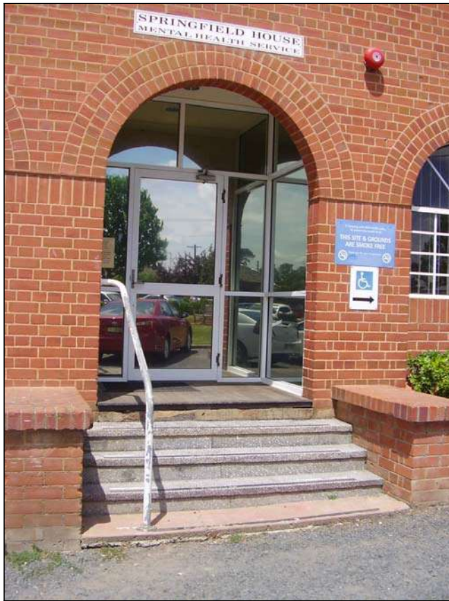
Figure 3.107 The main entry. Concrete and terrazzo steps extend up to the opening which retains the timber verandah flooring.
