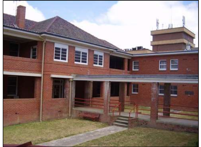
Figure 3.129 The walkway was also also constructed in 1938 and has terrazzo floor finish on concrete slab and brick base. Brick columns support the flat roof over.
