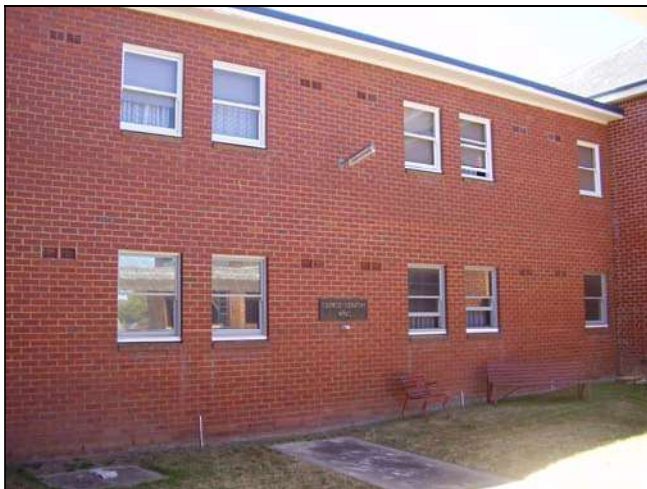
Figure 3.130 The Gerathy Wing is a simple brick structure with small timber framed windows and flat roof.
