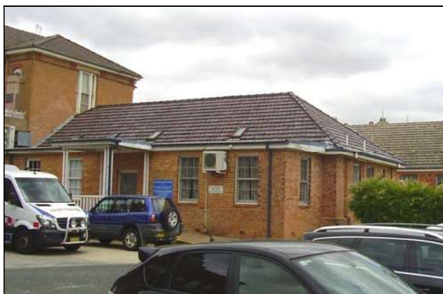
Figure 3.60 The single storey wing attached to the northern face of the western pavilion has a simple hipped and flat roof section clad in tiles and metal sheeting.
