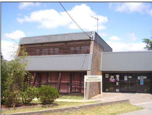
Figure 3.209 The main entry is located on the Goldsmith Street frontage, close to the corner of Faithfull Street.
