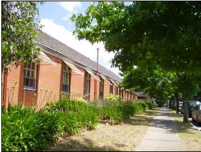
Figure 3.152 The Wet Wing is also constructed close to the Albert Street frontage. Simple bracketed awnings have been added to the west facing windows.
