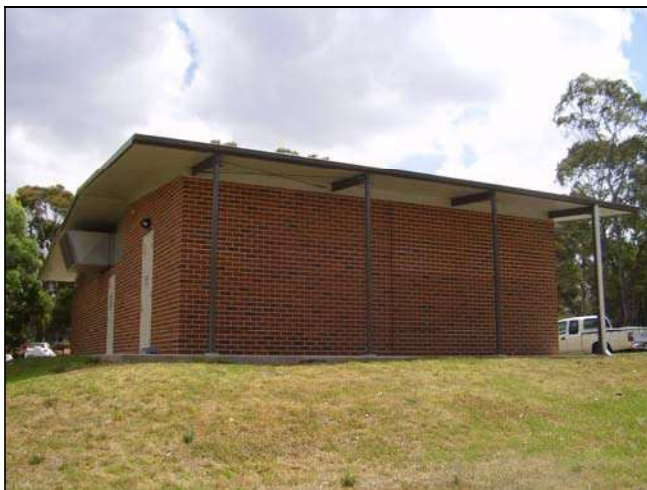
Figure 3.233 The northern and eastern façades of the building.
