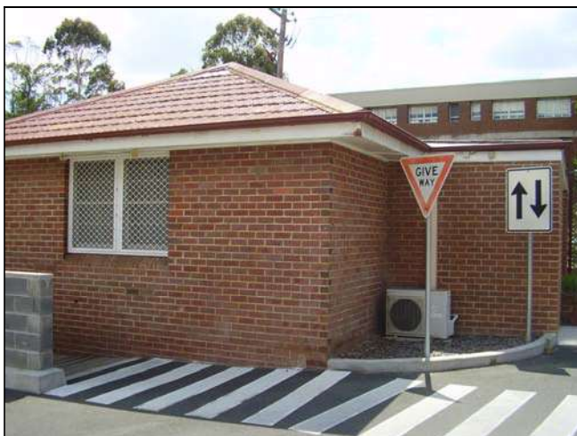
Figure 3.170 The eastern façade of the building which faces a recently formed car parking area.
