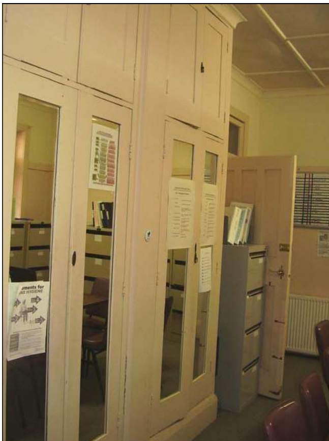
Figure 3.122 Some early built-in furniture also remains.
