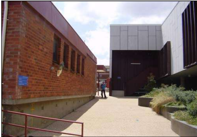
Figure 3.197 The northern façade of the 1970s addition to the building.
