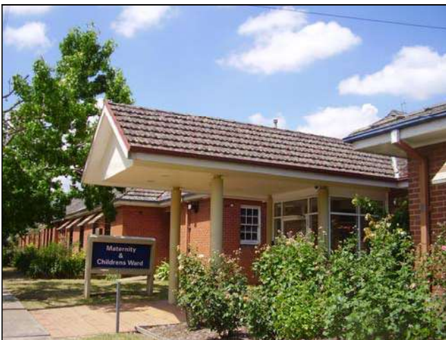
Figure 3.156 A gable roofed canopy extends from the northern end of the building to the Albert Street frontage.
