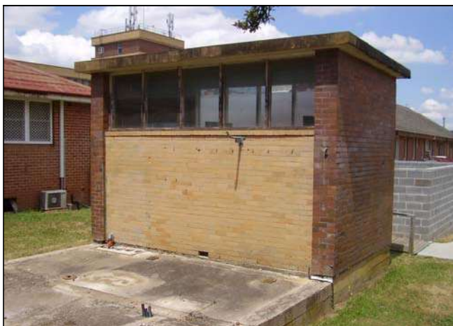
Figure 3.237 The former substation.
