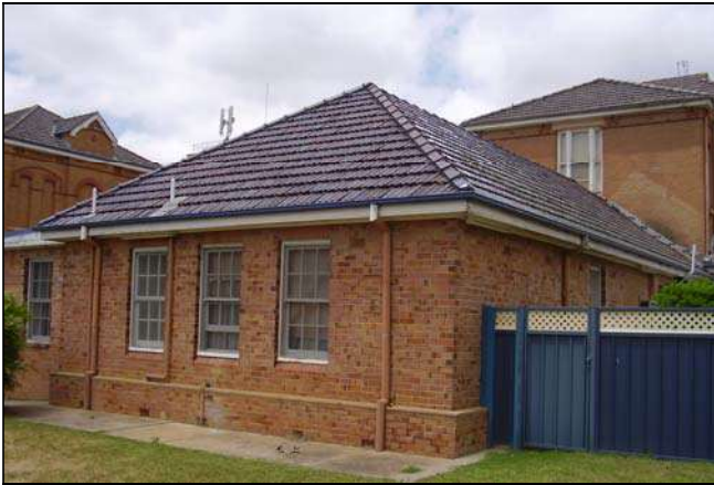
Figure 3.61 The north western wing which was extended and altered in the 1930s.
