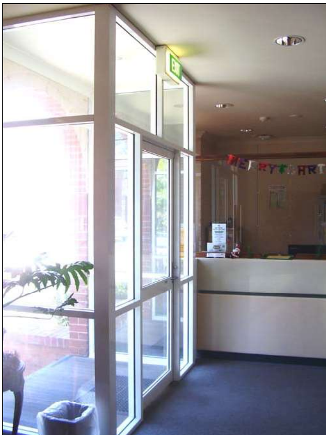
Figure 3.116 The building entry. Part of the ground floor verandah has been enclosed and refinished to provide a reception/ lobby area. The building has been converted for use by the Mental health Service with offices and rooms located on the ground floor.
