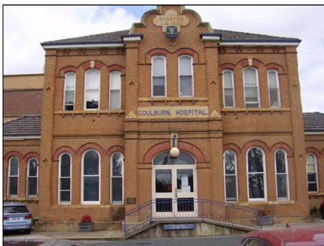
Figure 3.50 The front façade of the central pavilion is symmetrical about a parapeted projecting bay. The parapet is stone capped and has a stone with "Erected AD 1887" in relief lettering. The façade also has timber framed double hung windows with rounded and flat arch and later timber framed glazed door with arched toplight over and infill between.
