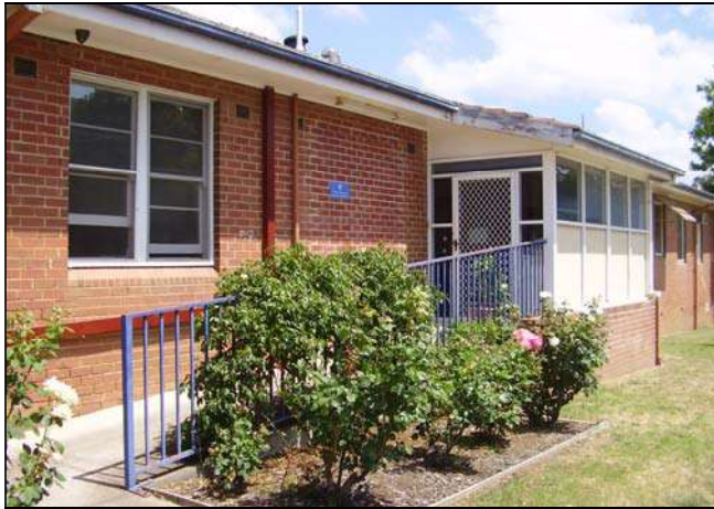
Figure 3.158 The western facade also has another entry and concrete ramp.
