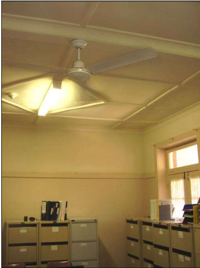
Figure 3.121 The building retains some early battened ceilings and timber windows and doors.
