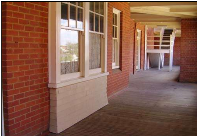
Figure 3.111 The southern ground floor verandah has timber floors and retains details such as a bay window, timber framed double hung windows and multi-paned French doors with terrazzo thresholds.
