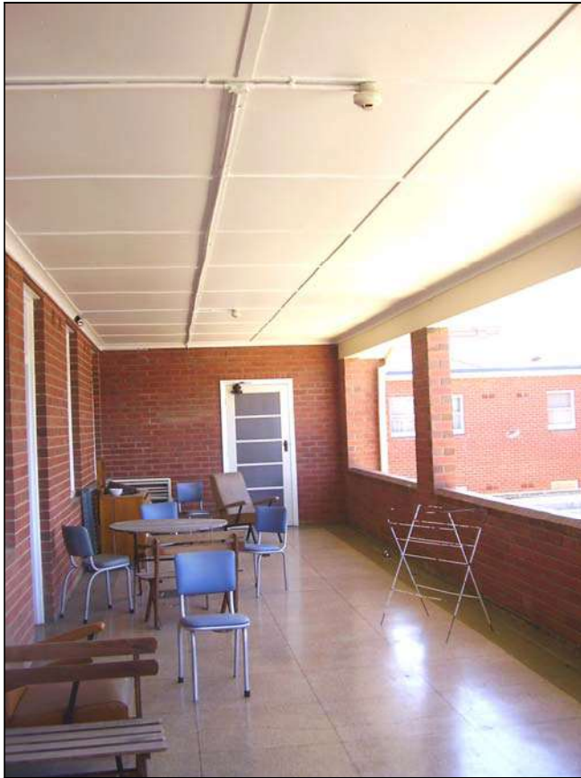
Figure 3.147 The first floor balcony which also has terrazzo floor finish, solid brick balustrade and batted ceiling.
