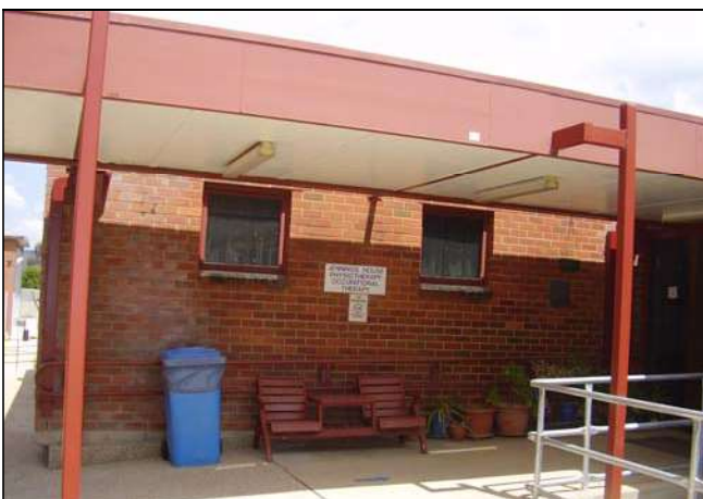
Figure 3.196 The eastern wing was added in the 1970s and accommodates Physio and Occupational Therapy. The entry also has a flat roofed canopy supported on simple steel posts.
