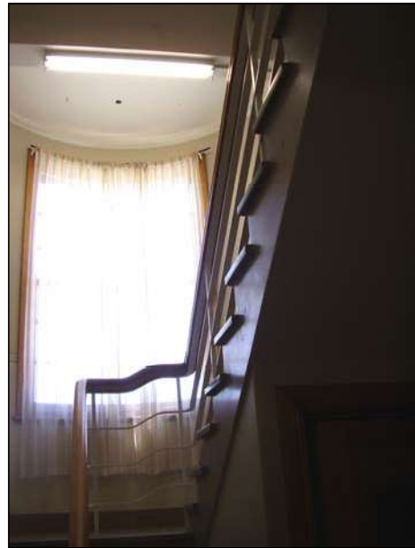
Figure 3.143 The stair has terrazzo finish and retains the original steel balustrade and curved stair window at the mid floor landing.
