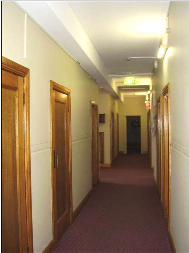
Figure 3.141 The ground floor corridor which has simple rendered walls with profiled dado detail and concrete slab ceiling over.
