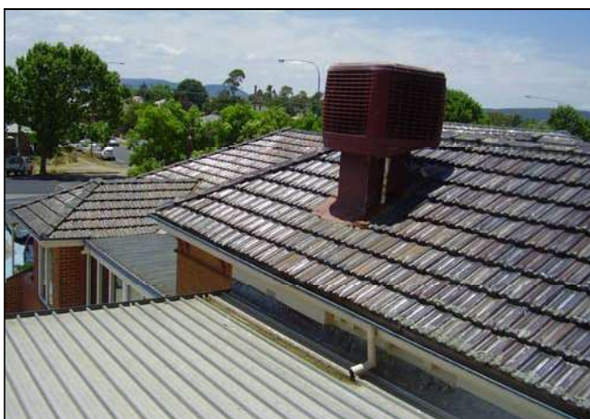
Figure 3.87 The various additions and infill are visible when looking at the roof over this section of the building.
