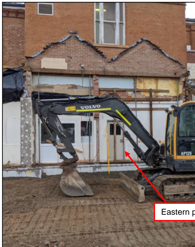
Figure 4.2 The area following the demolition which has revealed rendered and modified walls and parapet above the main corridor and bounding the first floor open walkway. The north eastern corner of the single storey section of the main pavilion has also been fully exposed. The earlier gabled roof form of the eastern pavilion is also apparent (at left).
