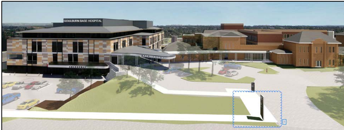
Figure 4 | Proposed hospital external treatments (Source: Modification 2 Application)
