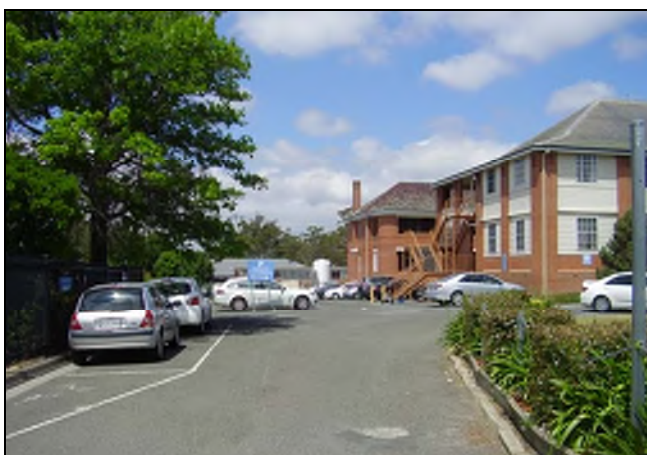
Figure 3.42 The secondary driveway accesses the staff car parking area located to the east of the Springfield House and Lady Grose House.
