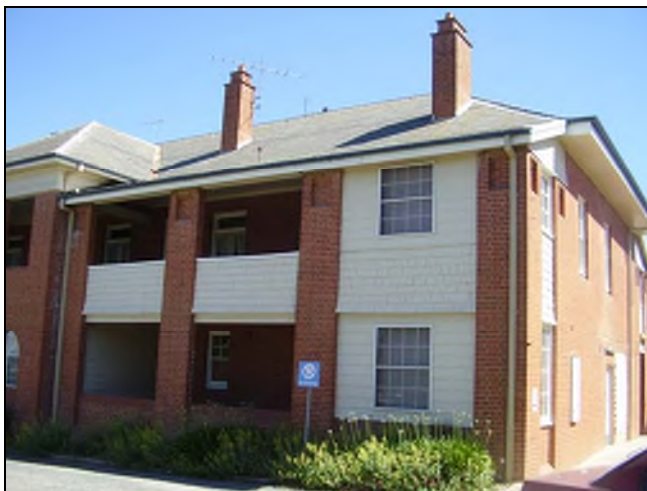
Figure 3.108 The north western corner and facades of the building. Note the lightweight infill to the end bays.
