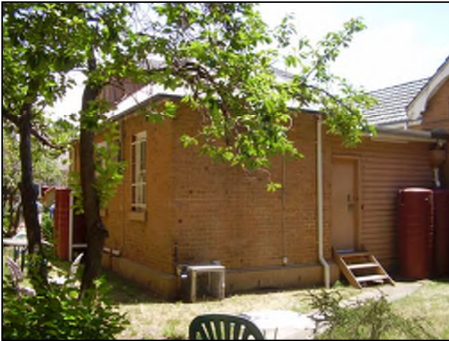
Figure 3.68 Additions dating from c. 1924 and 1960s at the western side of the original kitchen wing (now the Pharmacy).
