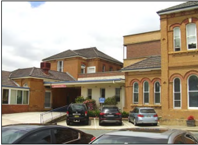
Figure 3.51 The eastern, two storey pavilion is similarly detailed with hipped and gabled hipped roof clad in tiles with bracketed detailing to the eaves. The original two storey walkways that connected the three pavilions remain discernible despite and various additions and infill between.
