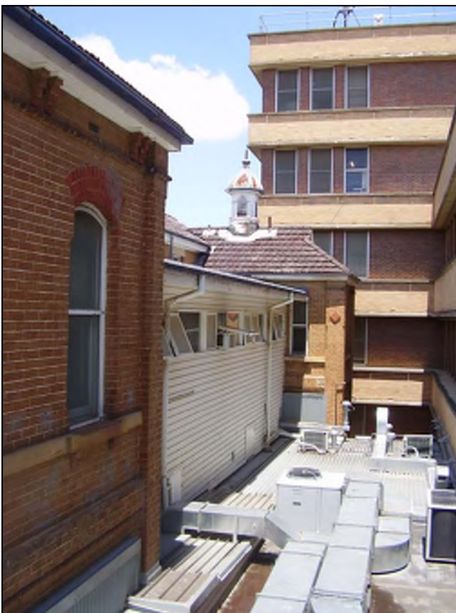
Figure 3.69 The multi-storey building constructed in the 1960s has been constructed to and adjoins the eastern pavilion.
