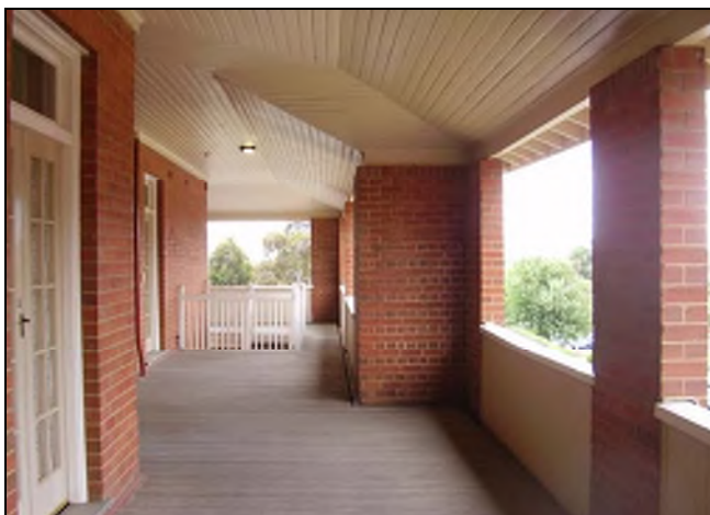
Figure 3.113 The southern balcony. The balconies also retain timber boarded ceiling/soffit.
