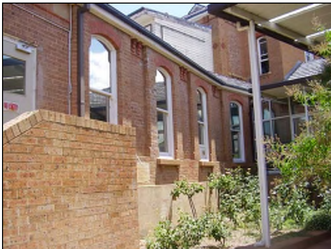
Figure 3.99 The wing is attached to the north eastern corner of the eastern pavilion. The north western façade features similar details to the original building including timber framed double hung windows with flat arched heads, contrasting brick and stone details, brick corbelling/ brackets at the eaves and also retains a stone foundation stone.
