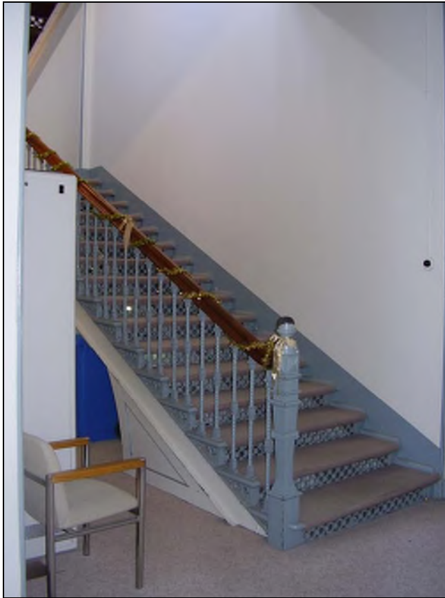
Figure 3.90 Each of three two storey pavilions retains a cast iron stair. The treads have been carpeted, however, the iron balustrade and timber handrails are in intact.
