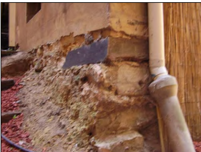
Figure 3.70 The rubble footings of the original building are partially exposed at the south western corner of the eastern pavilion.
