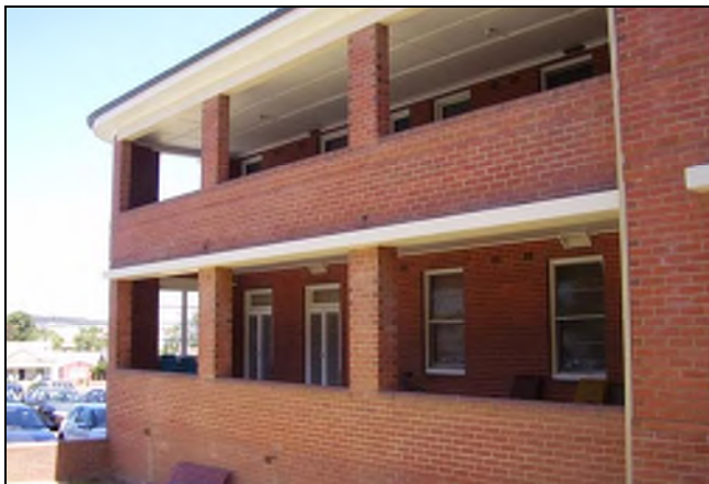
Figure 3.126 The The verandahs and balconies have solid brick balustrade and brick piers and are accessed by timber framed French doors.
