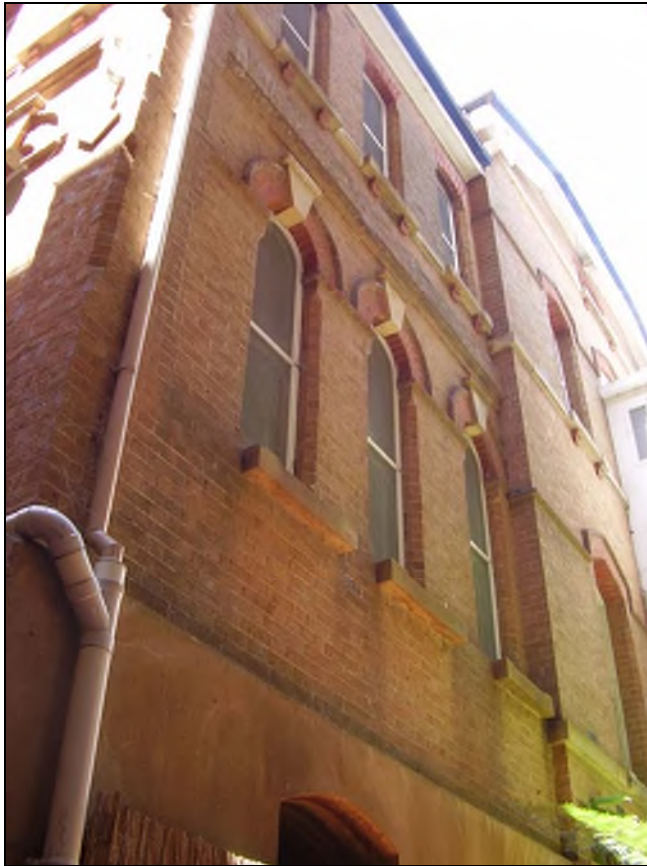
Figure 3.71 The southern façade of the eastern pavilion which remains highly intact externally. A lightweight bridge has also been added to connect to the 1960s addition.
