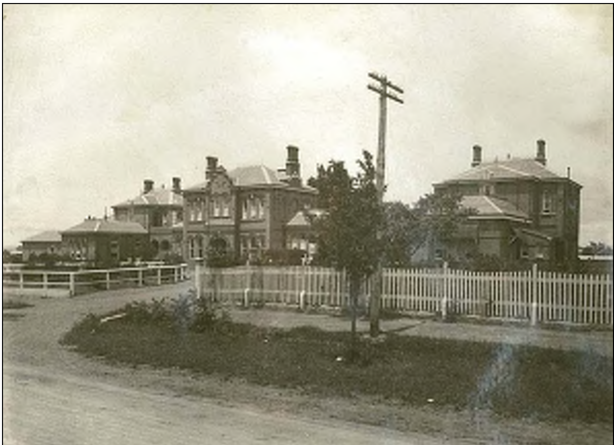
Figure 2.17 Undated photograph assumed to date 1920s-1930s showing the building and 1919 addition (at left). The verandah additions are also just visible. Also note the circular driveway and alteration of the front fence. (Source: Trove, State Records 4346_a020_a0200002)
