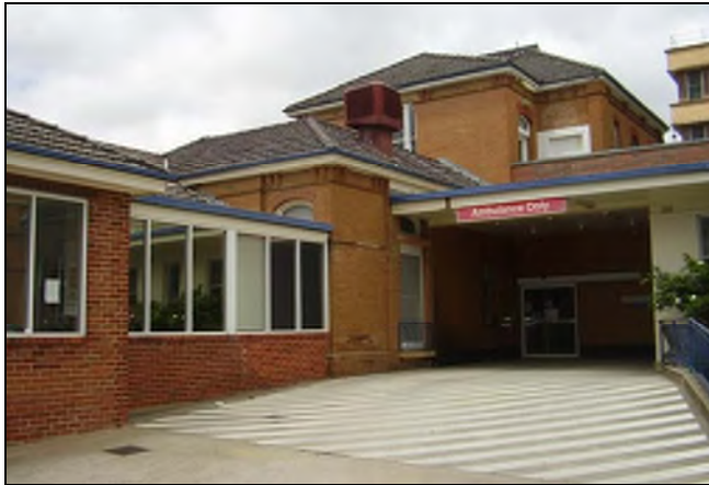
Figure 3.84 An ambulance bay with flat metal deck roof over and concrete ramp extending from the curved driveway has also been added to the front of the building.
