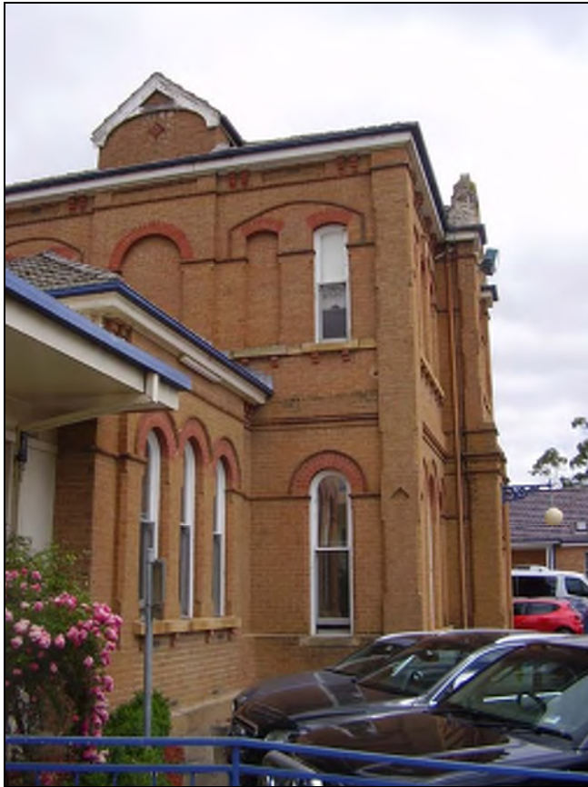
Figure 3.55 In addition to the single storey attached wings and walkways, the roof retains decorative gables. The chimneys were removed in the c. 1970s when the roof cladding was replaced.
