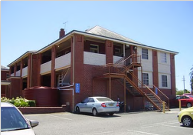
Figure 3.114 The south eastern corner and eastern façade of the building. Services have generally been added to the facades. An external fire stair has also been added to the eastern façade. A staff car parking area is also located to the east of the building.
