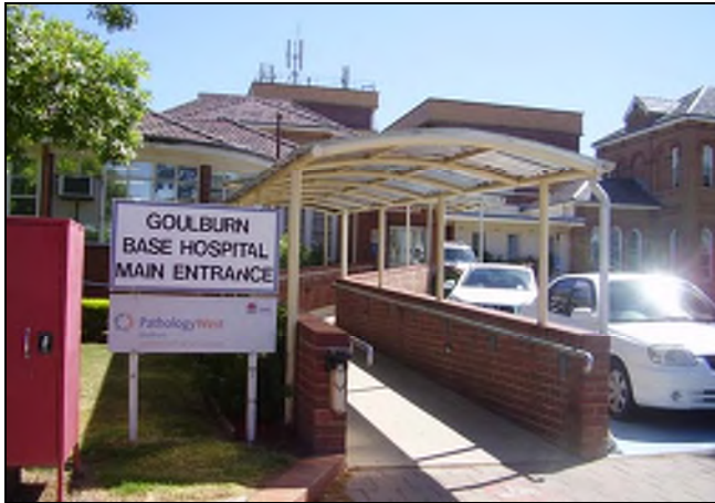
Figure 3.18 A covered concrete access ramp and steps have also been added to the main entry.
