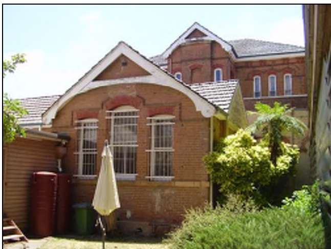
Figure 3.67 The rear of the central pavilion and part of the original kitchen wing.
