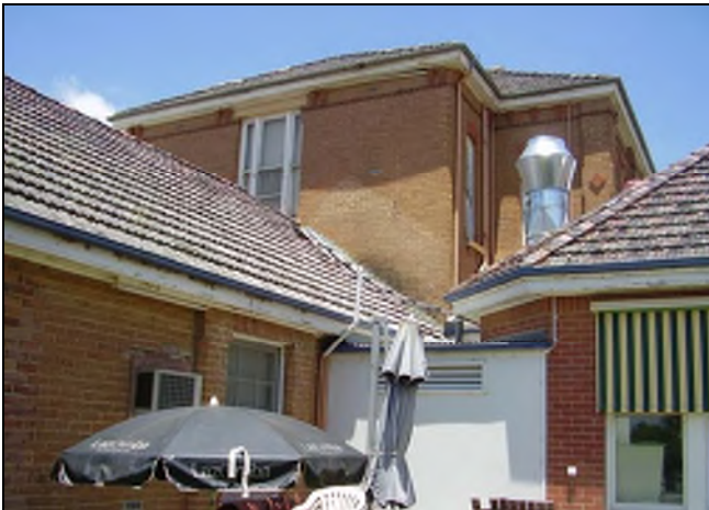
Figure 3.63 The northern façade of the two storey western pavilion also retains evidence of the original roof form over the original north western single storey wing.
