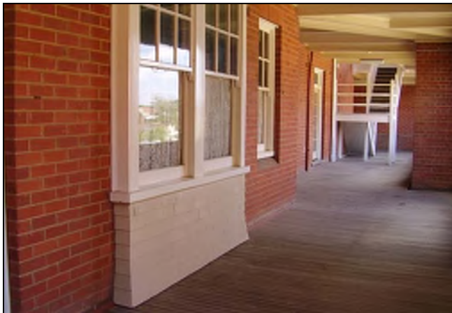
Figure 3.111 The southern ground floor verandah has timber floors and retains details such as a bay window, timber framed double hung windows and multi-paned French doors with terrazzo thresholds.
