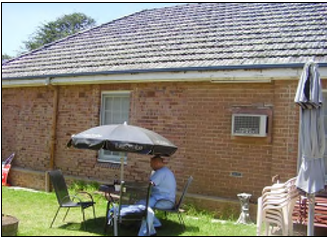
Figure 3.62 The extent of the original north western wing and later addition is clear on the western façade where the differing brickwork and junction is clear.
