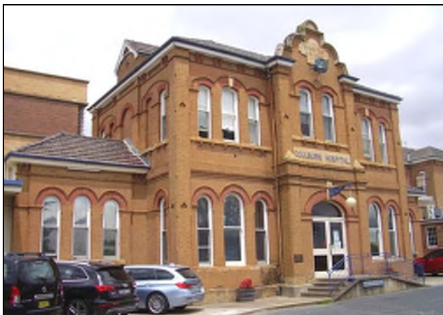
Figure 3.53 In addition to the single storey attached wings and walkways, the roof retains decorative gables. The original chimneys were removed in the c. 1970s when the slate roofing was removed and replaced with tiles.
