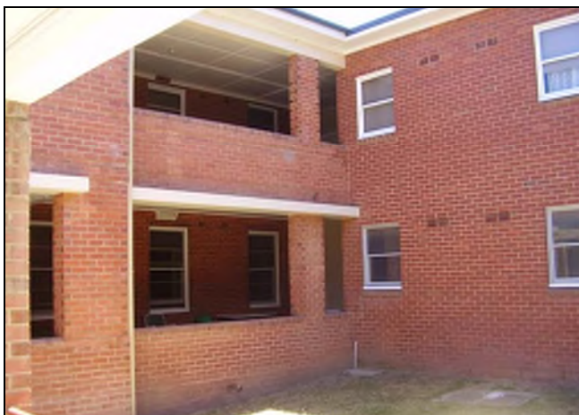
Figure 3.128 The Gerathy Wing has been constructed to the north western corner of the building.
