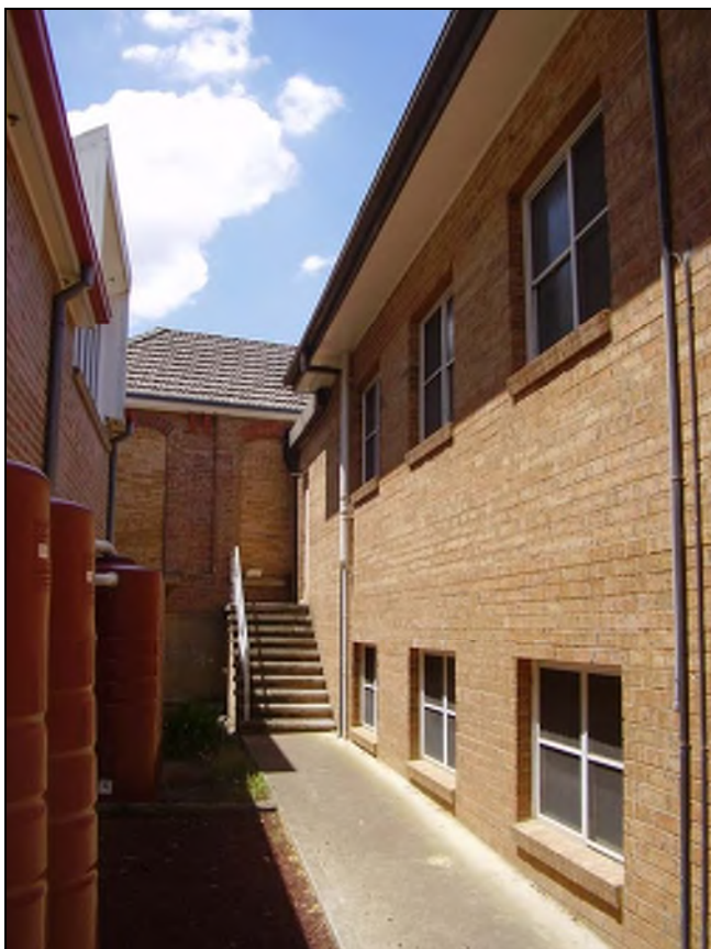
Figure 3.103 The western façade of the 1989 addition which also has aluminium framed windows with simple brick sills. Part of the southern facade of the 1919 wing remains, however, openings appear to have been infilled with bricks.
