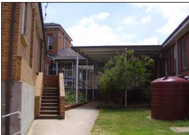
Figure 3.75 The courtyard area formed by the various additions to the northern end of the eastern pavilion including the former Children's Ward (now Admin and Medical Records).
