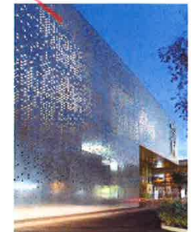
PERFORATED ALUMINUM PANEL AT FIRE STAIRS LOWER GROUND + LEVEL 3, & ROOFTOP PLANTROOM AREAS
