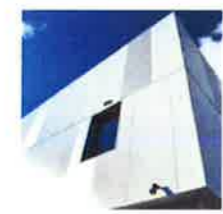
CFC CFC PANEL TO UPPER LEVELS
