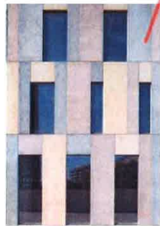
CFC PANELS ON UPPER LEVELS
