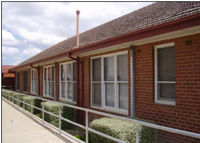
Figure 3.195 The 1950s, western portion of the building retains timber framed windows. Note the landscaping, path and railing recently added to the front of the building.
