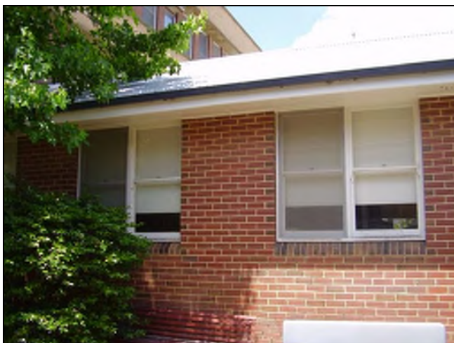
Figure 3.167 The north western facade.
