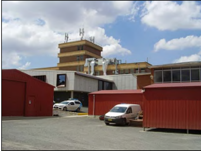
Figure 3.224 The Biomedical Engineering and Waste Management Building are part of a group of simple steel structures located to the south east of the main Hospital buildings.
