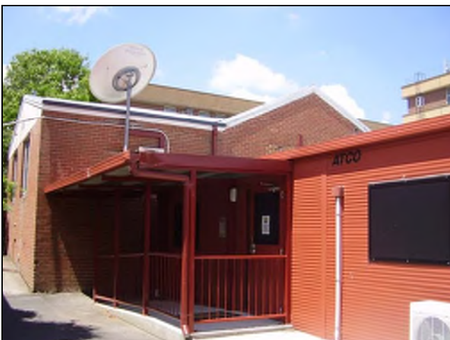
Figure 3.164 A demountable (Uni) building abuts the southern façade of the building.
