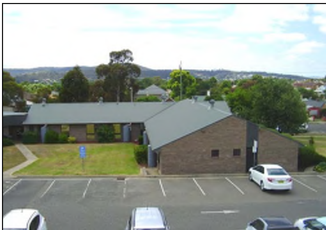
Figure 3.212 The rear of the southern wing of the building which appears to have been constructed after 2005.
