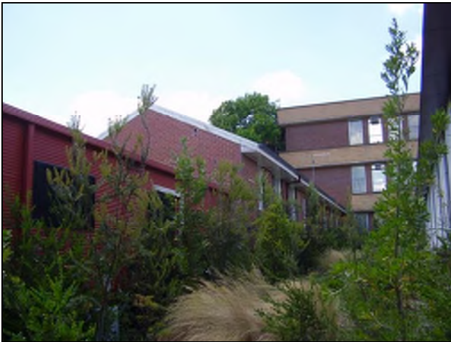
Figure 3.162 The building is a simple single storey face brick structure located in the western section of the site and to the west of the multi-storey 1960s building.
