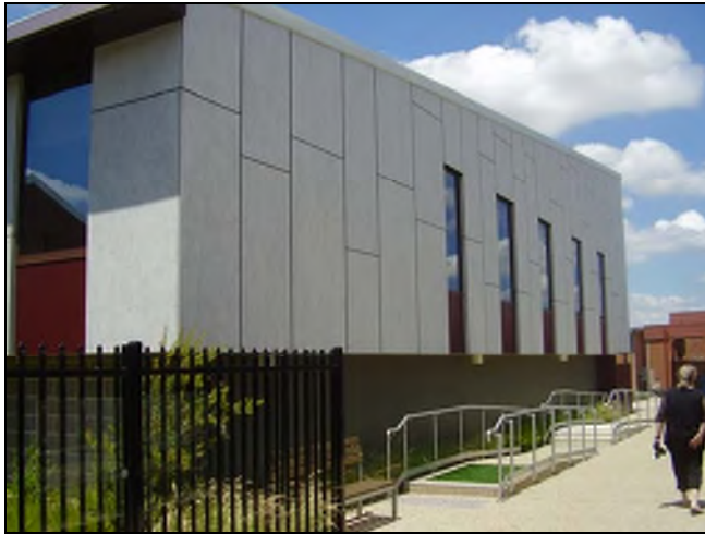
Figure 3.190 The south western façade.
