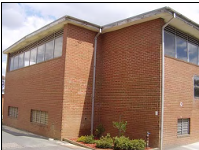
Figure 3.203 The “rear” of the building.
