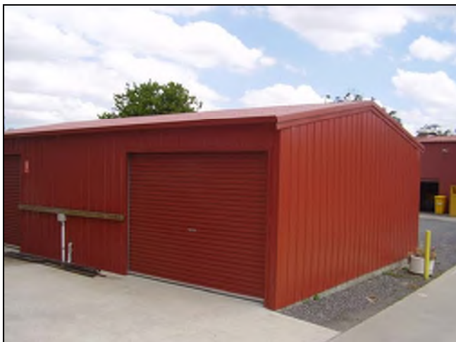
Figure 3.230 One of the other service buildings
