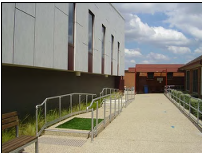
Figure 3.191 The paving and landscape elements, including rehab fixtures located to the south of the building.
