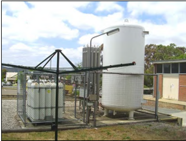
Figure 3.238 One of the other service buildings
