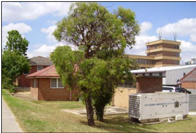
Figure 3.235 The former substation and other slabs and service elements located to the north of the Power and Generator Room and south of the Antenatal Clinic.
