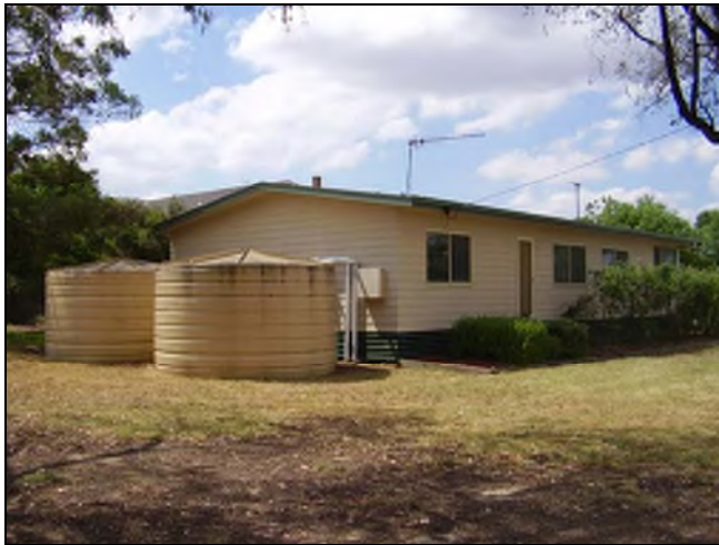
Figure 3.214 The Early Childhood Centre is a simple lightweight building located close to the Faithfull Street frontage.
