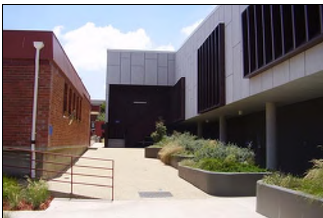
Figure 3.189 New paths and landscapes elements have been added around the building and particularly to the south.
