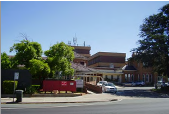
Figure 3.171 The 1960s building is a highly visible addition to the Hospital with the three and five storey building visible from Goldsmith Street and main entry to the site.
