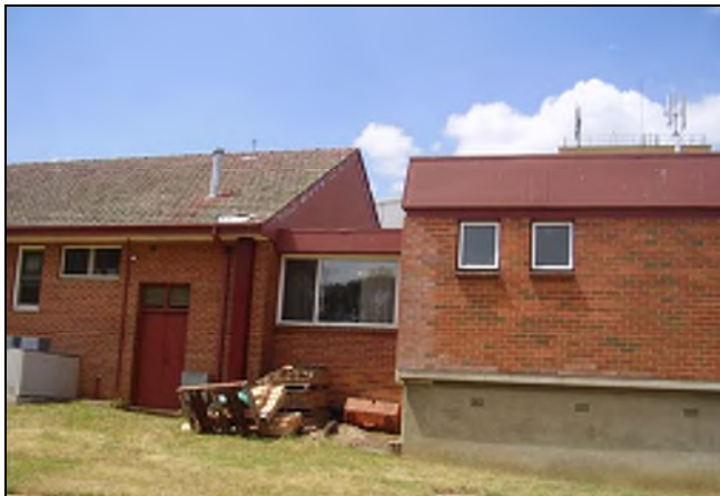
Figure 3.199 The connection between the two wings of the building.
