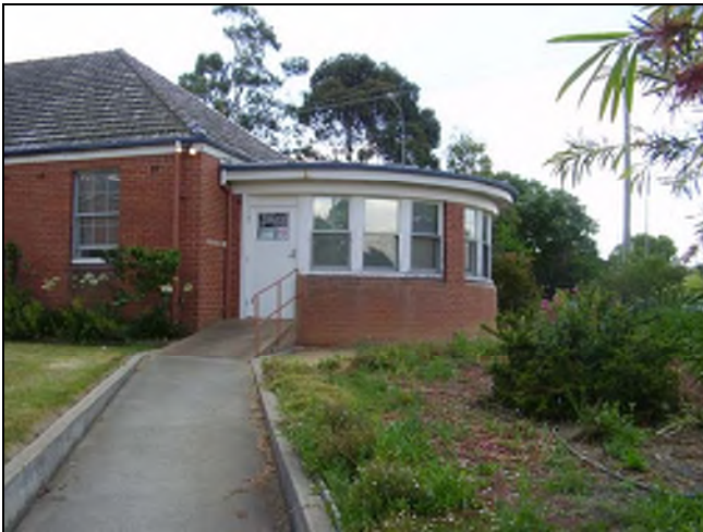
Figure 3.150 The northern end of the building features a curved end bay with flat roof over clad in metal sheeting and timber framed windows and doors. Constructed as a sitting room it is surrounded by planted garden and also overlooks Goldsmith Street.
