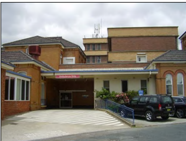
Figure 3.173 The 1960s building from the front circular driveway.
