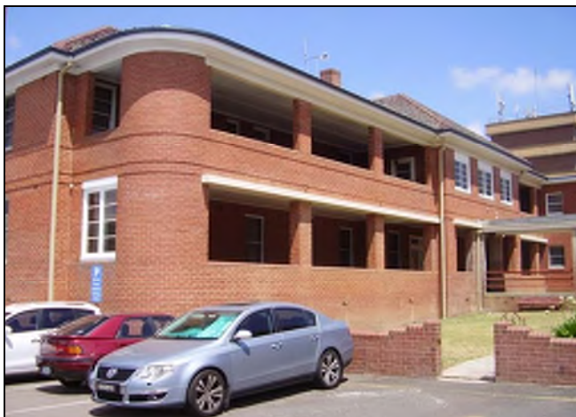
Figure 3.137 The access to the building from the staff car parking area.
