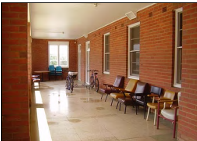
Figure 3.138 The ground floor verandah space which retains terrazzo floor finish, timber framed windows and doors.
