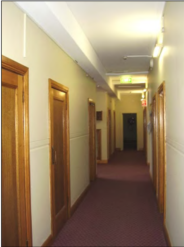
Figure 3.141 The ground floor corridor which has simple rendered walls with profiled dado detail and concrete slab ceiling over.
