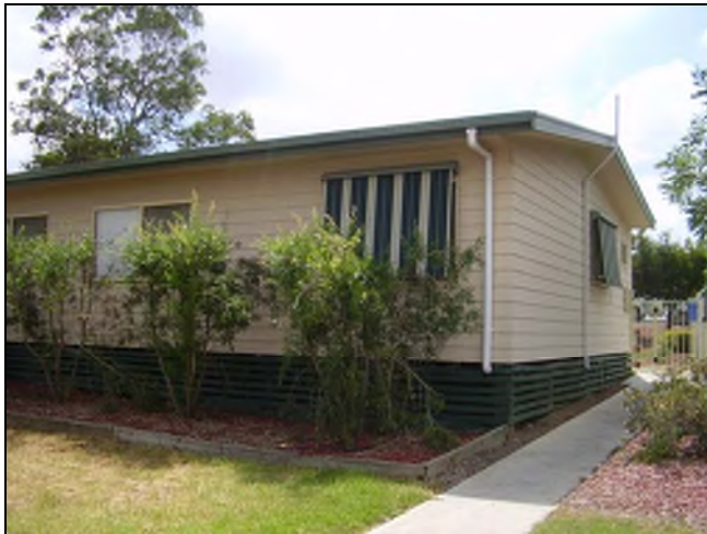
Figure 3.215 The northern end of the building.
