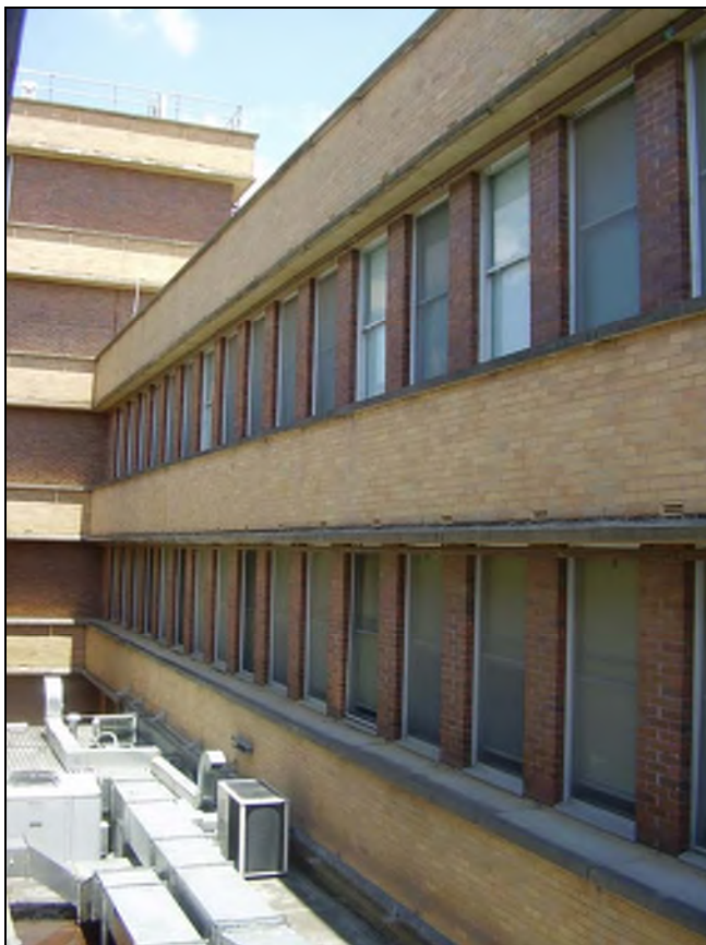
Figure 3.175 The north eastern façade of the building.
