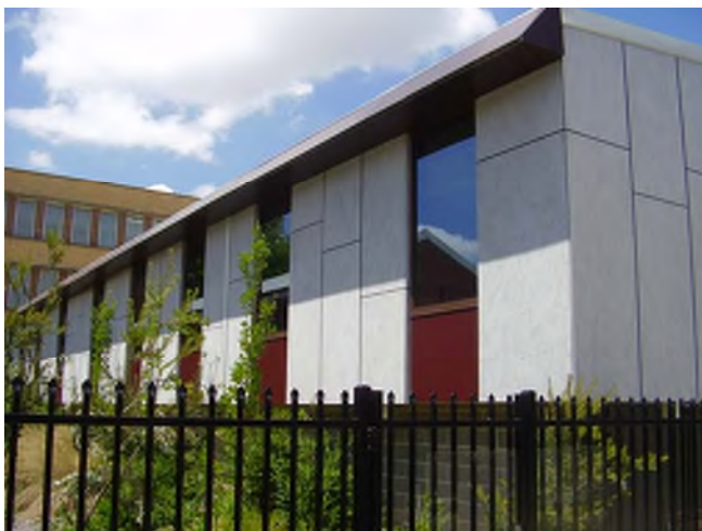
Figure 3.192 The western façade of the building.
