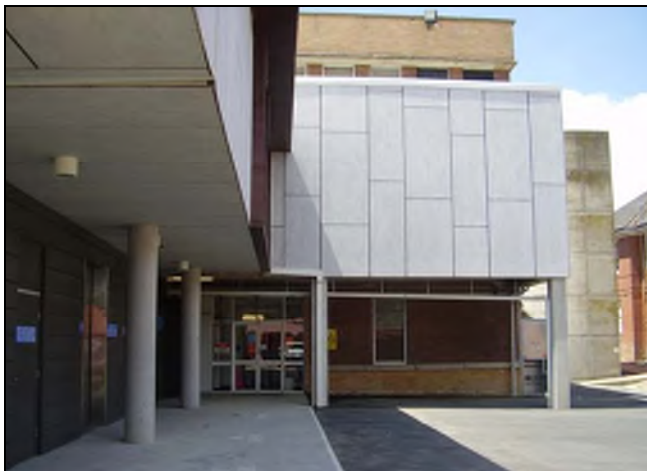
Figure 3.187 The service entry and loading dock area.
