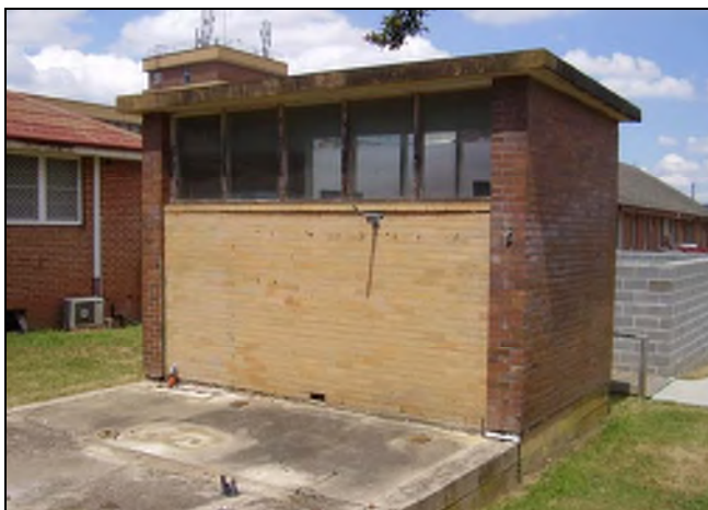
Figure 3.237 The former substation.
