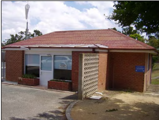
Figure 3.168 The Antenatal Clinic is a small face brick building located close to the Albert Street frontage. The building has hipped roof clad in pressed metal and metals sheeting with rolled joints.
