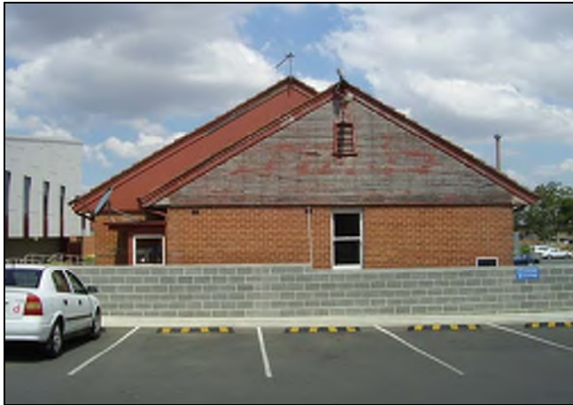
Figure 3.193 The western façade of the building which retains the original double gable timber boarding and vent and sheeted finish to the gable ends.
