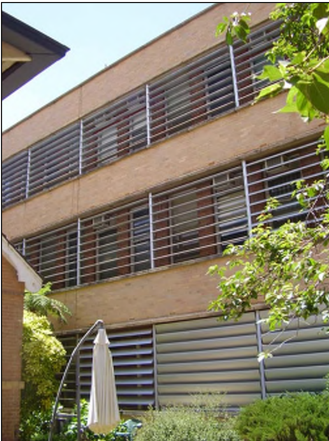
Figure 3.182 Sun-shading louvres have been added to the western façade of the northern, Emergency wing which faces an open courtyard space also bounded by the 3 storey main block, remainder of the original kitchen wing and rear of the western pavilion.
