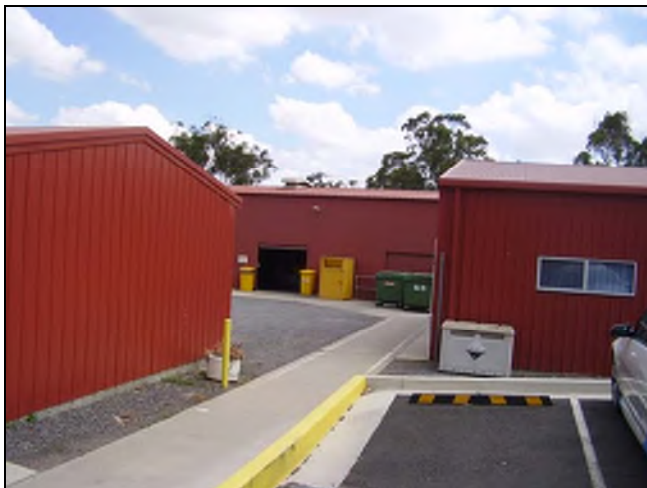
Figure 3.225 The group are accessed by two service roads and are surrounded by sealed area.
