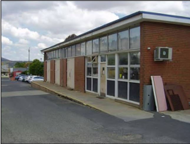
Figure 3.204 The northern façade of the building with has brick and both aluminium and steel framed glazed windows.
