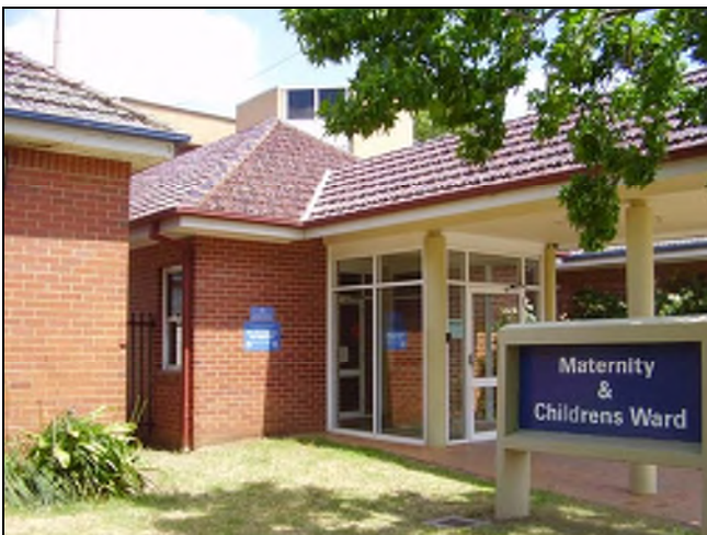
Figure 3.157 The canopy and attached wing are a later addition to the building and site. Other modifications include the aluminium framed doors and signage.
