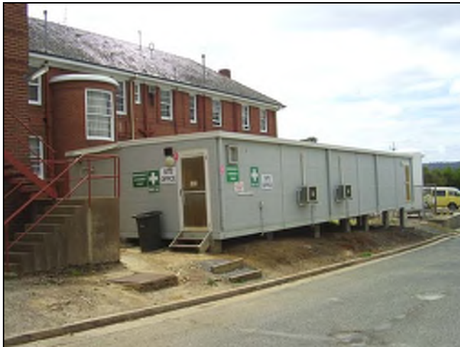
Figure 3.239 Demountable located to the south of Lady Grose House and north of the main service road extending from Faithfull Street.
