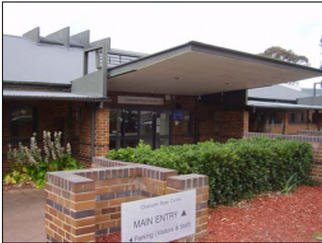
Figure 3.217 The entry facing Clifford Street.
