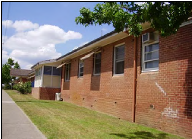
Figure 3.159 The south western façade.
