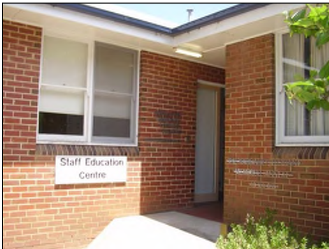
Figure 3.166 The main entry is located at the junction of the two wings of the building. The Zella Fife Memorial Lecture Theatre (1956) which extends in a north south orientation and the southern wing, the Margaret Tustian Memorial Annexe (1959).
