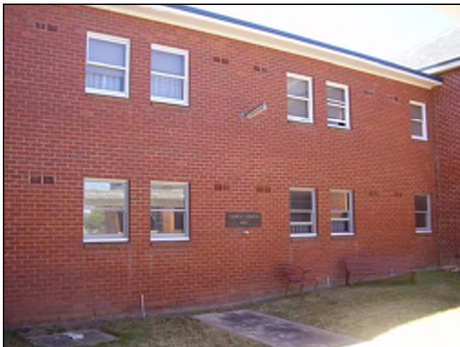
Figure 3.130 The Gerathy Wing is a simple brick structure with small timber framed windows and flat roof.
