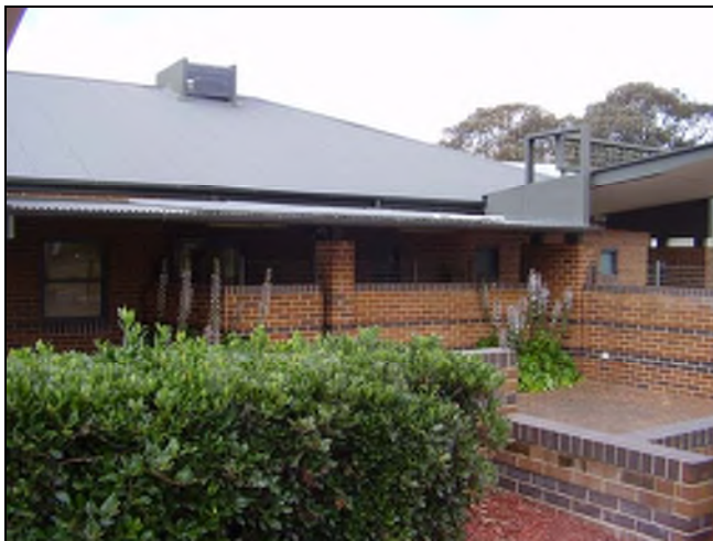
Figure 3.218 The building comprises a number of wings constructed in two stages.
