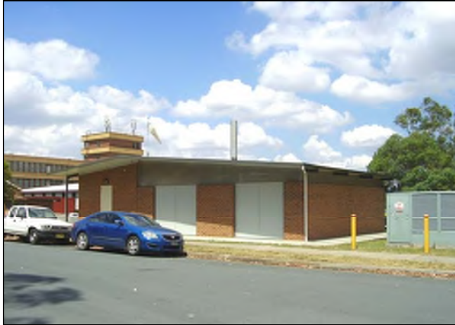
Figure 3.231 The recently constructed Power and Generator Room located near the corner of Albert and Clifford Streets.
