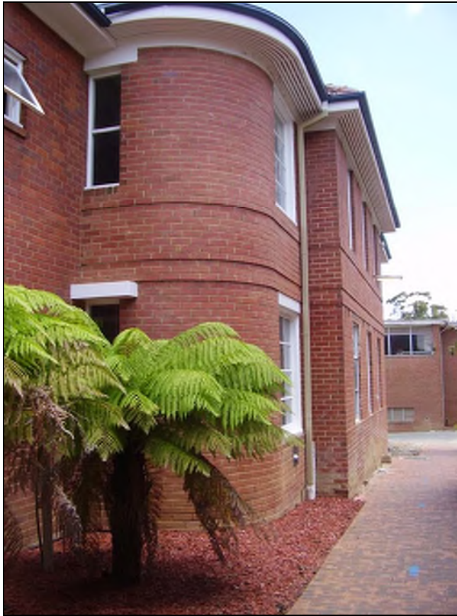
Figure 3.132 The curved corner detail and brick detailing and finishes such as the battened eaves remain. Some landscaping and paving has been added around the building and some changes such as alteration of openings are also visible.
