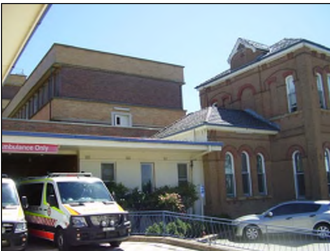
Figure 3.172 The northern (Emergency ) wing is constructed to the main building with door opening onto the open, elevated walkway between the central and eastern pavilions of the main Hospital building.
