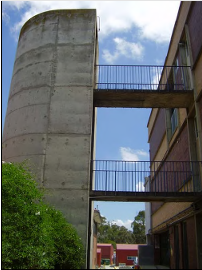
Figure 3.178 A concrete stair is attached to the eastern, Theatre wing of the building.
