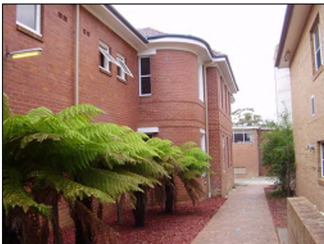
Figure 3.131 The western façade of the Gerathy Wing and Lady Grose Home.
