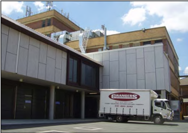
Figure 3.181 A two storey ward and rehab unit has recently (2013) been constructed to the southern facade of the building.
