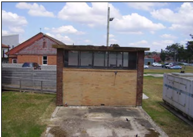
Figure 3.236 The former substation.
