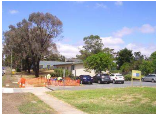
Figure 25: Some trees and buildings mark the Faithfull Street frontage which also has a driveway which accesses staff parking area and service buildings in the mid section of the site. (Source: PMA)
