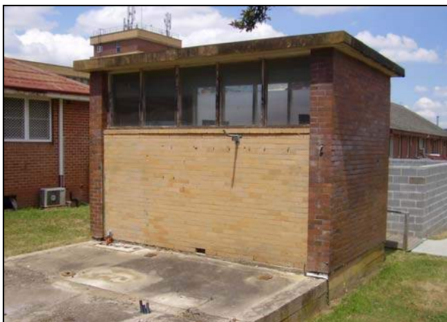
Figure 3.237 The former substation.
