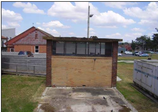
Figure 3.236 The former substation.
