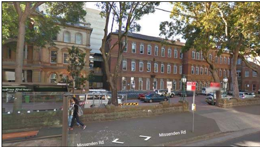
Figure 4.10 One of the other service buildings
