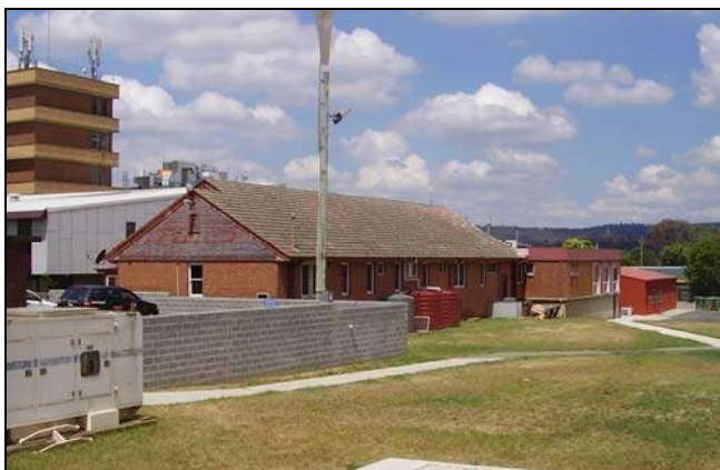
Figure 3.200 The rear, southern façade of the building faces the helipad.
