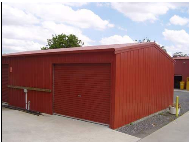
Figure 3.230 One of the other service buildings
