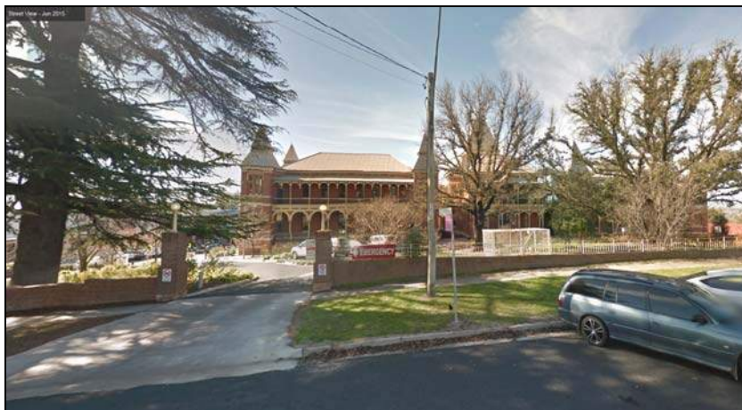
Figure 4.11 Bathurst Base Hospital.
