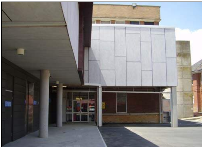
Figure 3.187 The service entry and loading dock area.
