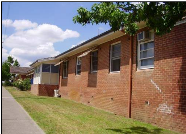
Figure 3.159 The south western façade.
