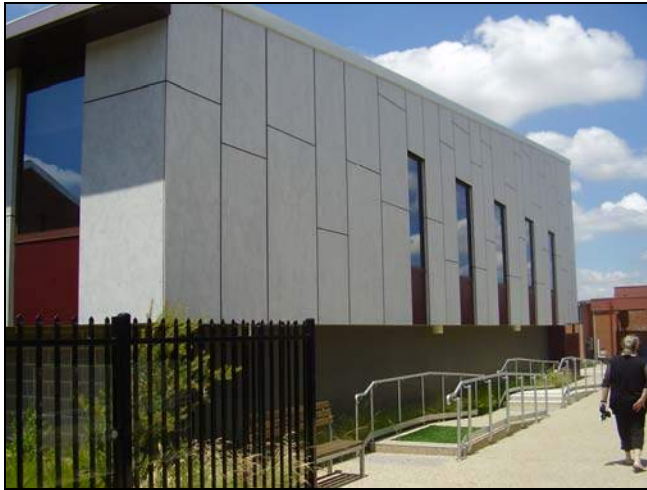
Figure 3.190 The south western façade.
