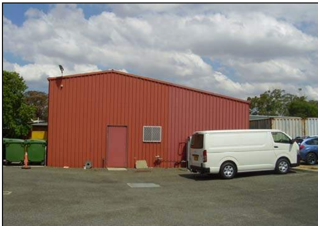
Figure 3.229 The Waste Management Building.
