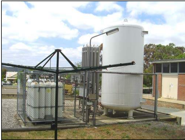
Figure 3.238 One of the other service buildings
