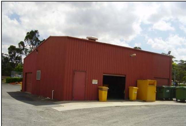
Figure 3.228 The Waste Management Building.
