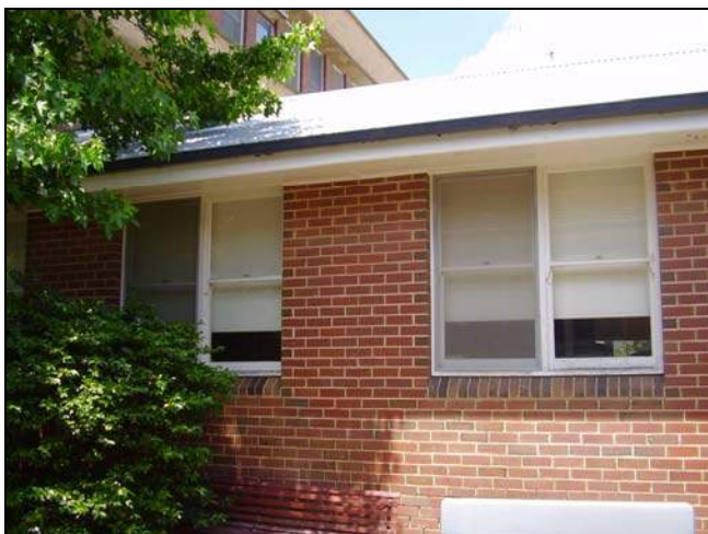
Figure 3.167 The north western facade.
