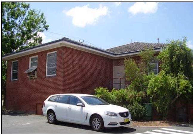
Figure 3.160 The southern façade of the building.
