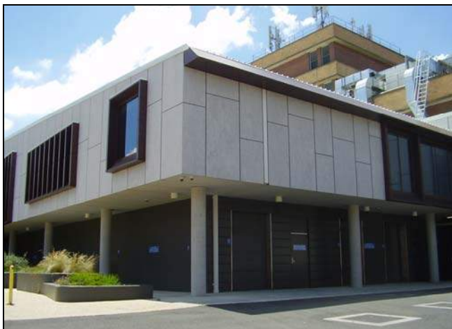
Figure 3.188 The south eastern corner of the building.
