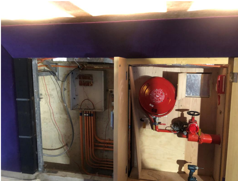
View of partially removed carpet clad wall, showing fire hose reel, electrical services, and uplighting of beams
