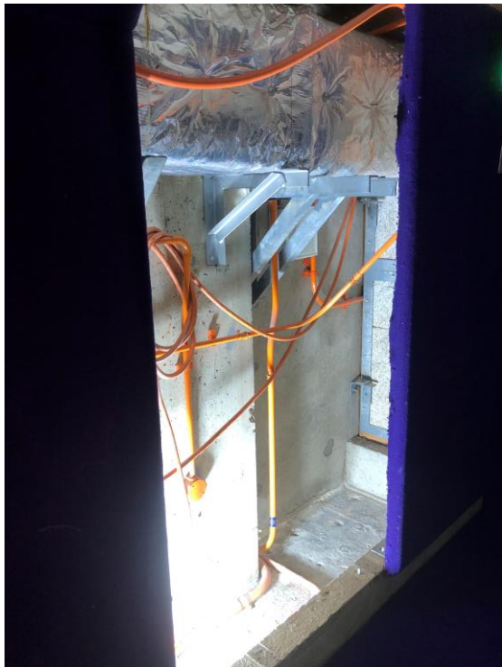
View behind carpet clad wall, showing a/c duct, electrical services and floor level lower beyond plinth
