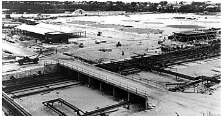
Figure 17: Construction of the Caltex Oil Refinery (1954)
