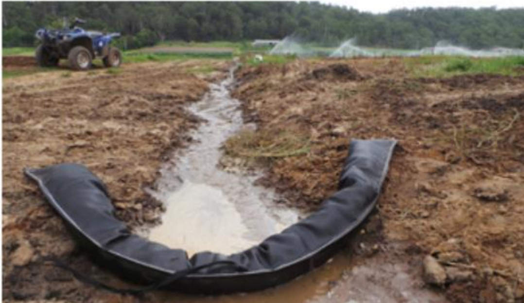
Figure 10 Star Water Filter Sausages (Safe Sox) used to filter metals and other pollutants
