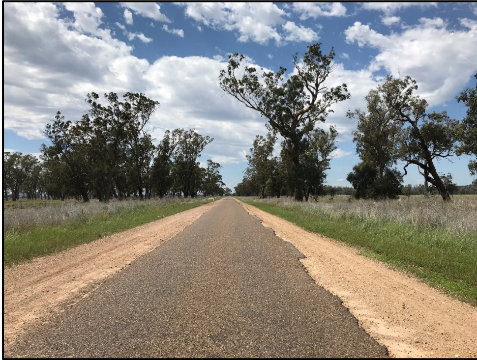
Photo 5 – Typical cross section of Old Blue Vale Road
