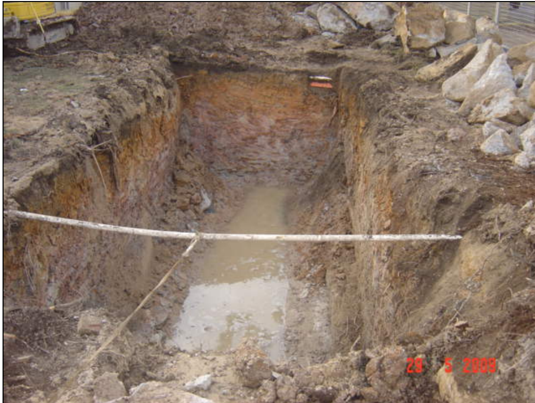
Photograph 5: UST Excavation- facing east
