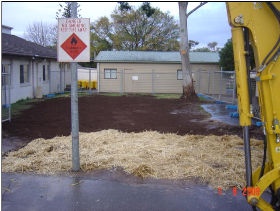
Photograph 7: Completed UST Removal and Validation Site – facing east
