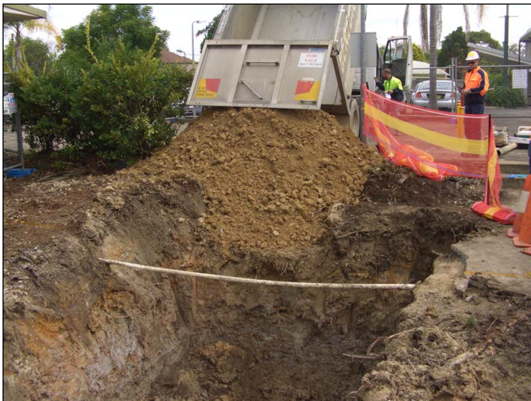
Photograph 6: Reinstatement of Excavation with Imported VENM – facing west
