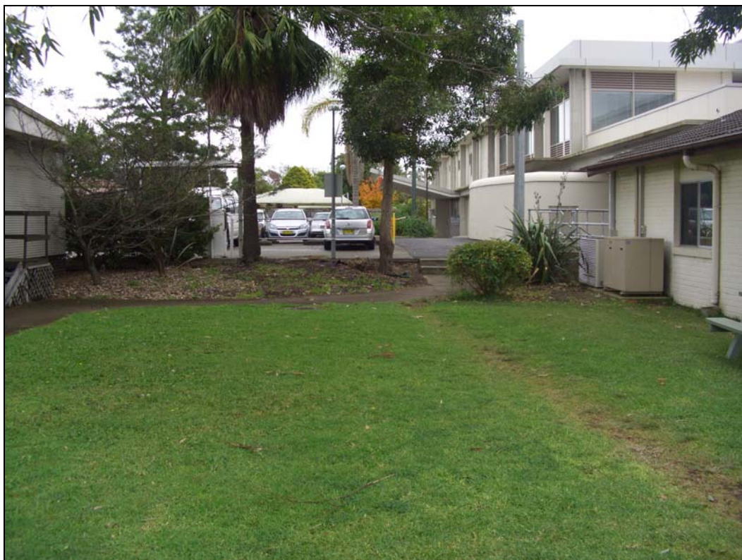
Photograph 2: Area of UST – facing west
