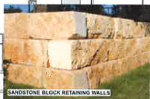
SANDSTONE BLOCK RETAINING WALLS
