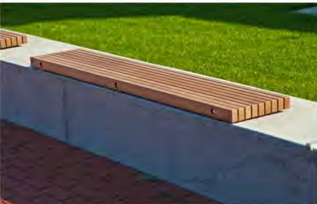
MODWOOD DECKING TO TOP OF MASONRY BLOCK WALL AS BEACH SEATS
