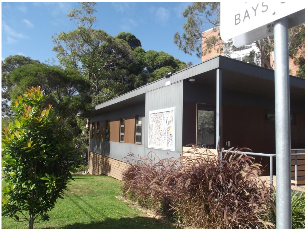
Figure 70: Building 53 EPIS on Lowe Road
