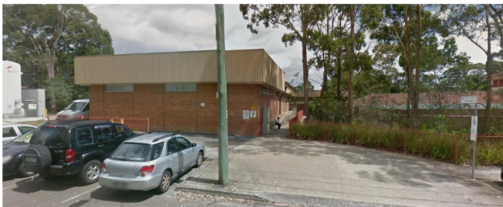
Figure 91: Gate 7 circa 2013 prior to the demolition of Building 4. Google Streetview
