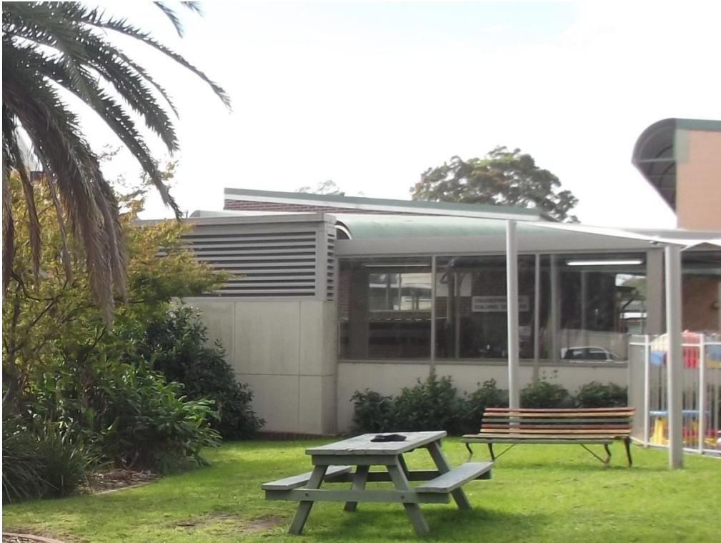
Figure 62: Building 47 just visible on the far side of the covered walkway. Number 47 sign in centre of image.
