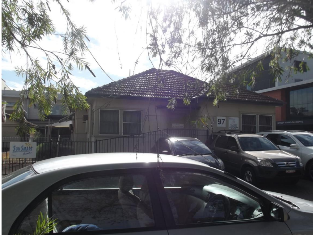
Figure 78: Building 97 from Burdett Street.
