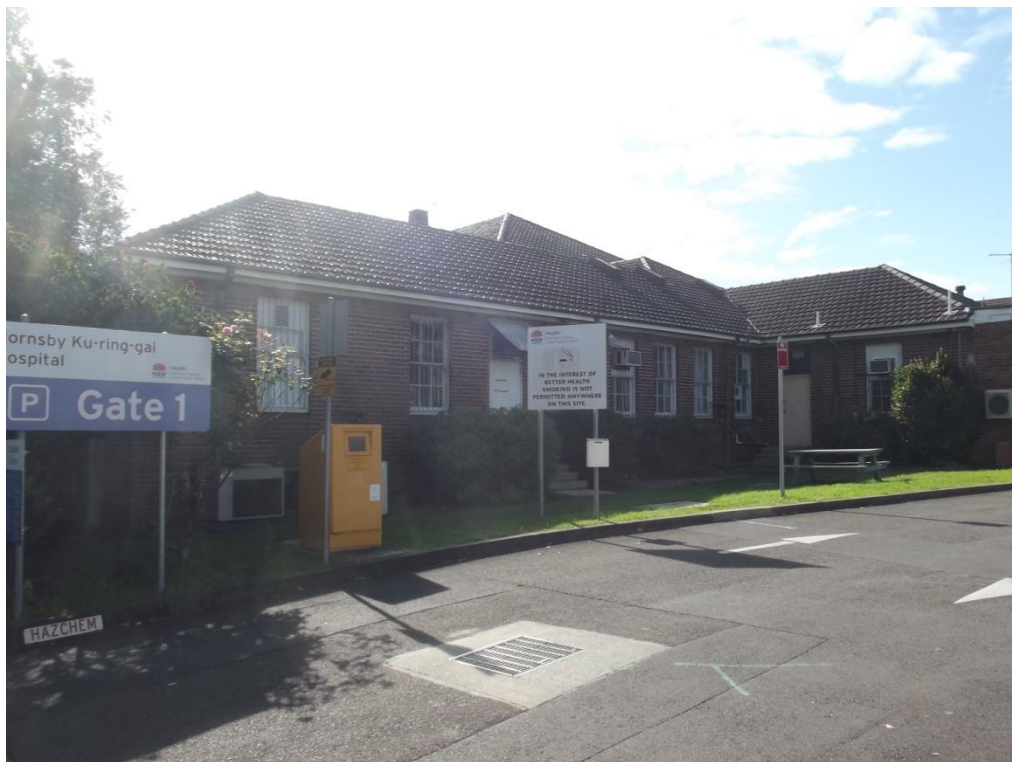
Figure 79: Gate 1 from Palmerston Road. Building 1 directly beyond. External doors to building 1 are purely service doors.
