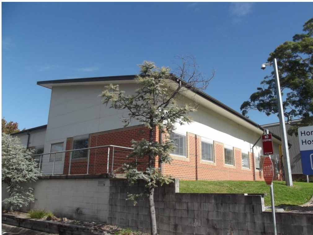
Figure 66: Building 51 taken from the Gate 5 location on Lowe Road.
