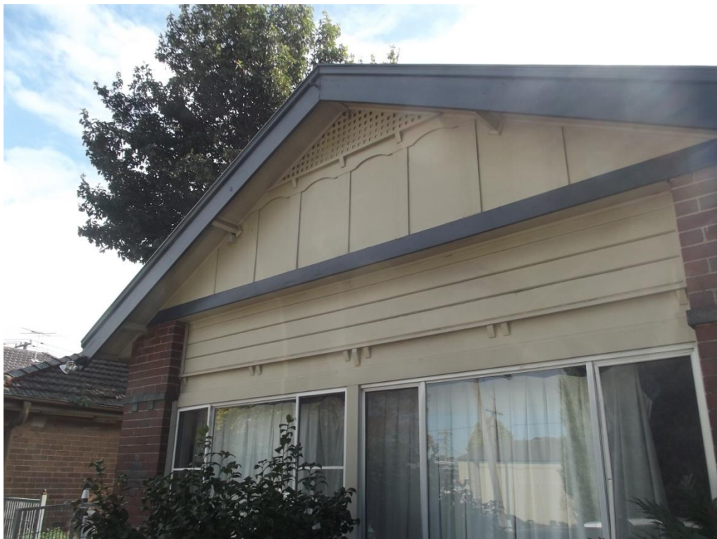
Figure 75: Detail of decorated gable. Also note brickwork details in darker and corbelled bricks to the verandah pillars.
