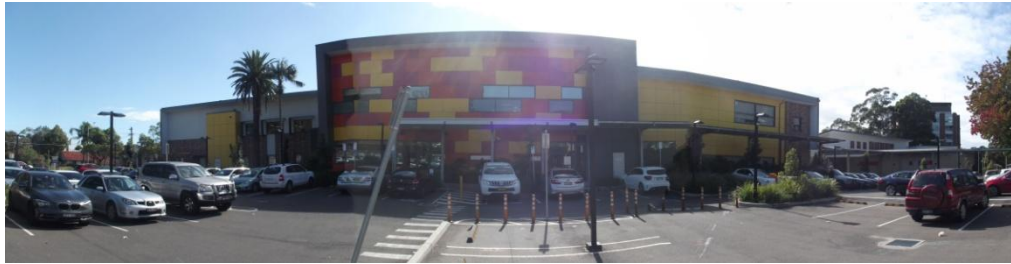
Figure 67: Panorama image of South side of Mental Health Centre looking North across car park.
