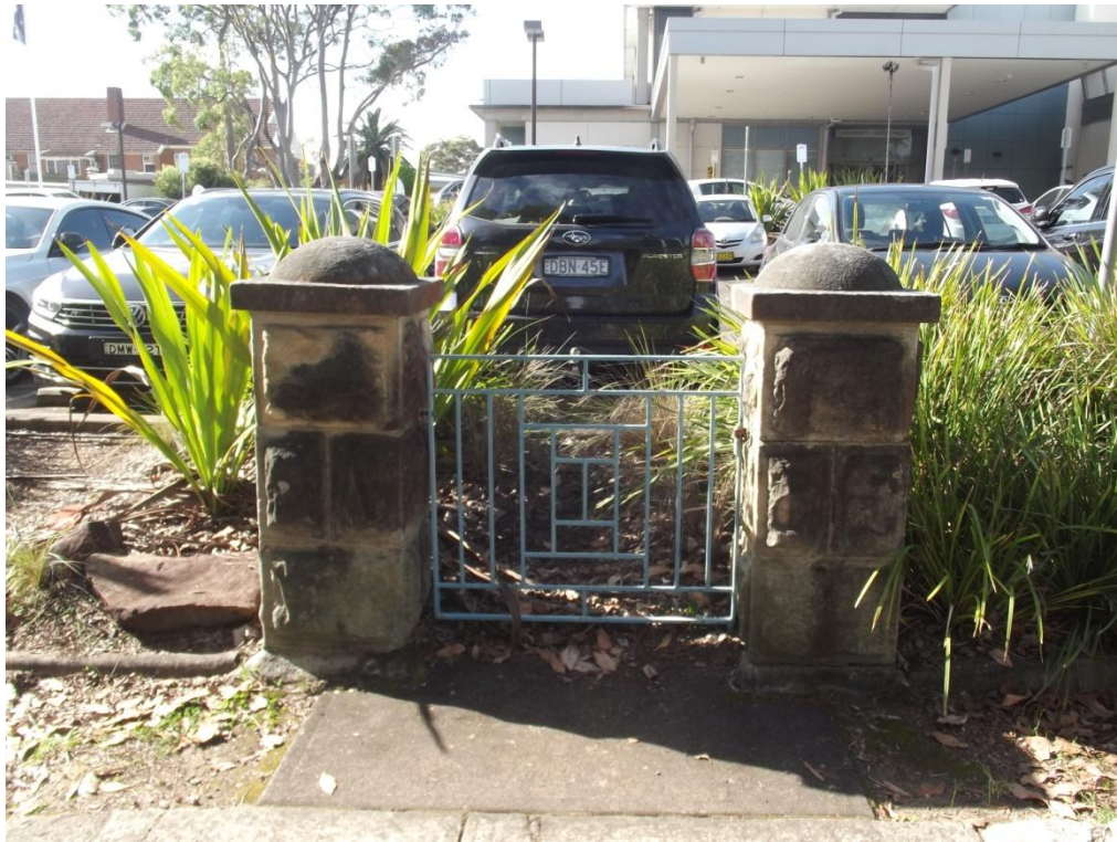
Figure 81: Gateposts and wrought iron gate south of Gate 1
