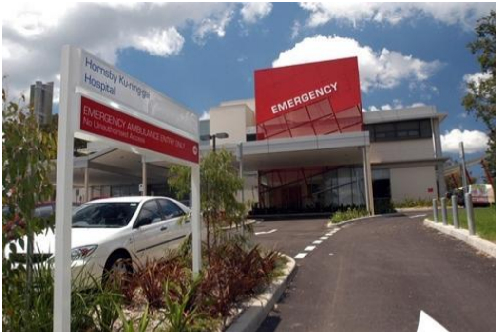
Figure 63: HOPE Building viewed from Palmerston Road showing main entrance.
