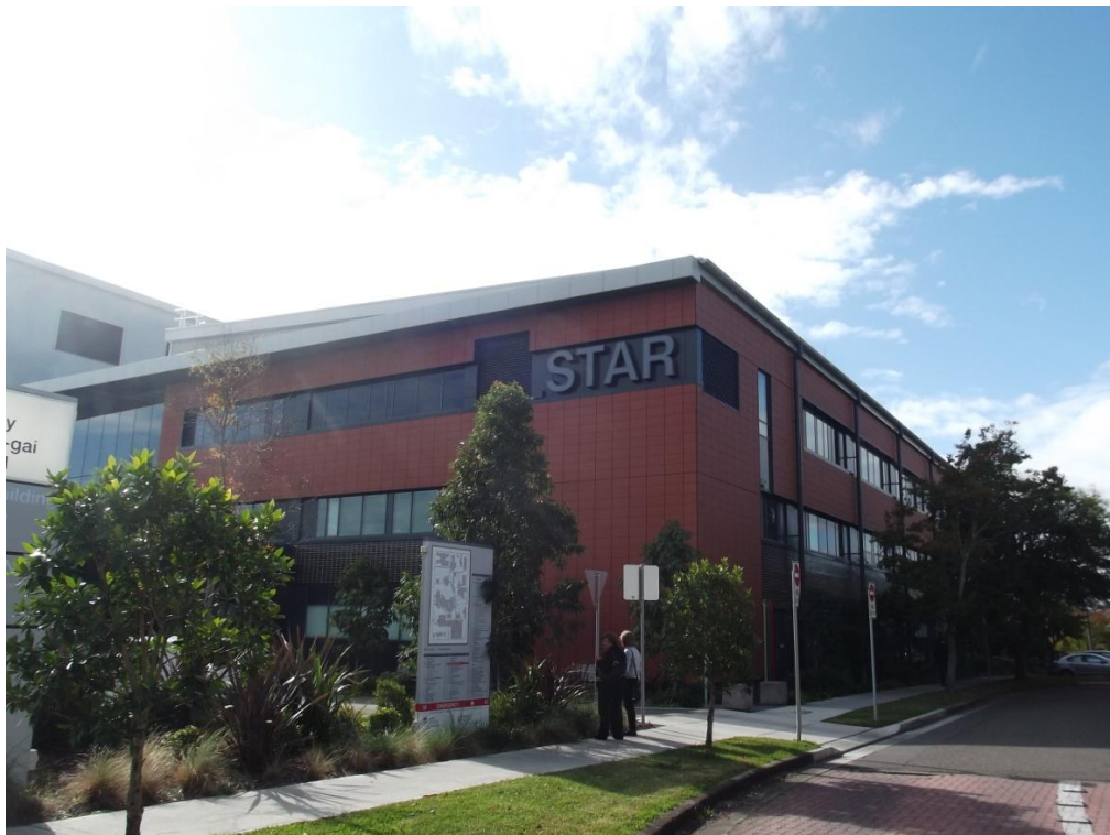
Figure 72: The STAR building from Burdett Street
