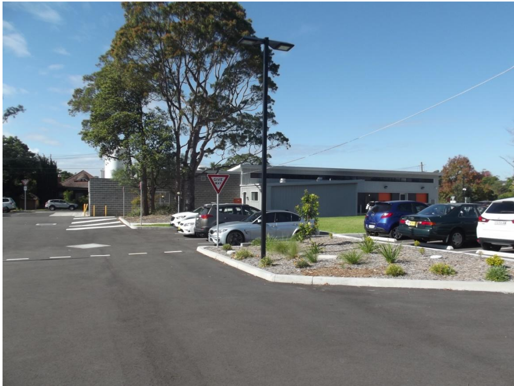
Figure 71: Building 54 looking east toward Derby Road
