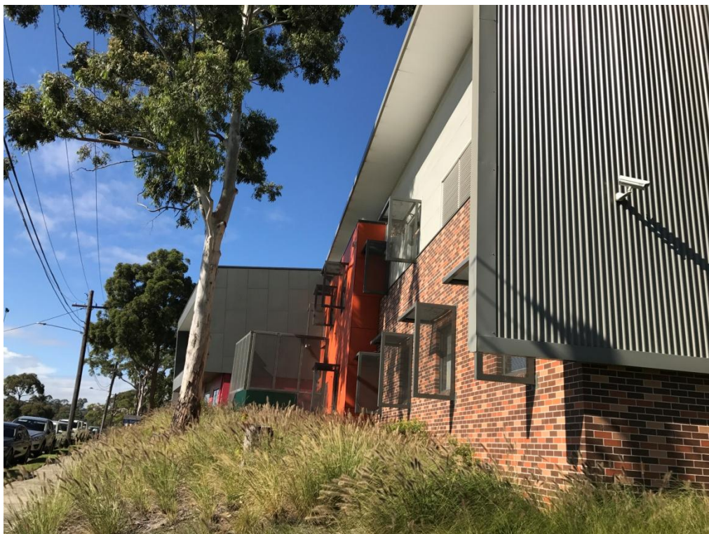
Figure 68: Mental Health Centre, looking East along Lowe Road. Viewing balcony is the grey form on the upper floor beyond the tree in the image.
