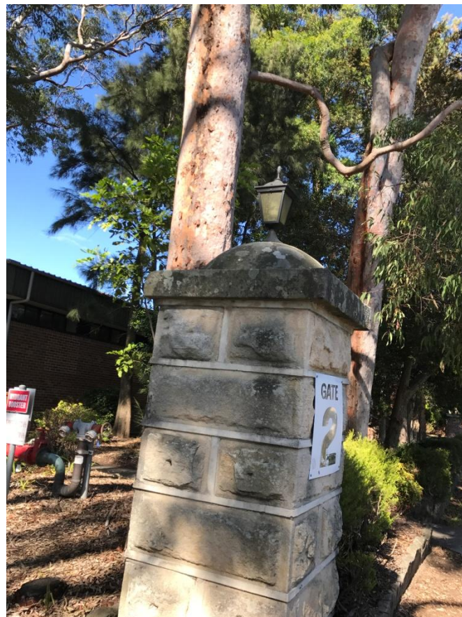
Figure 84: Gate 2 detail, note lamp fitting at the apex which probably dates from the late 1940s when it is compared with Gate 3
