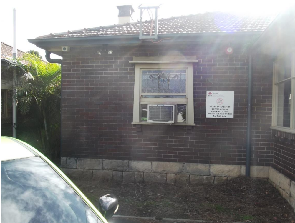
Figure 77: Detail of decorative window frame, glazing and stone foundations.
