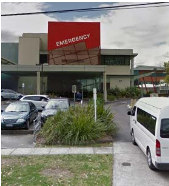
Figure 38 Existing Emergency Signage
