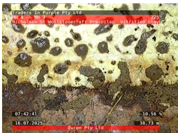
11, 00:09:02, 38.73 Point repair, localised lining--less than the complete inspection length, length: 600mm from 12 o'clock to 12 o'clock, Finish #
