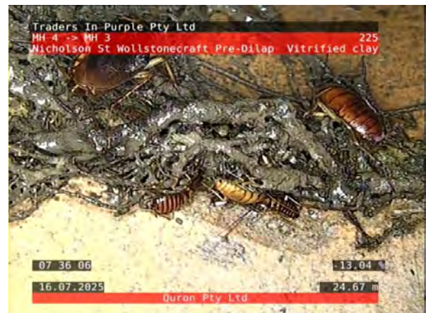
4, 00:04:54, 24.67 Fine roots--a relatively small number of flexible minor roots, at joint, Obstruction: 5-20% from 2 o'clock to 5 o'clock
