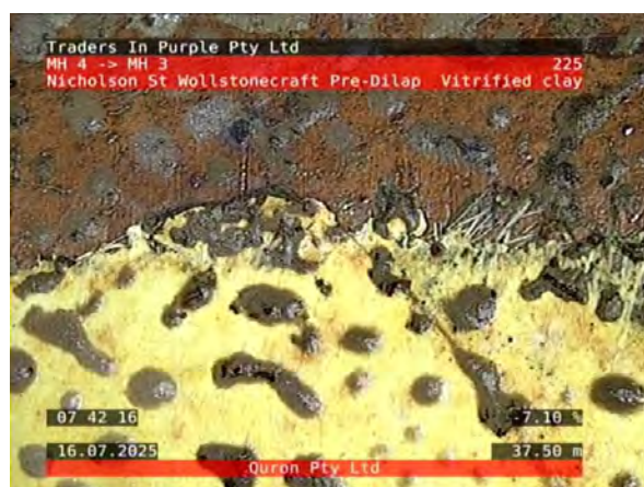
10, 00:08:44, 37.50 Point repair, localised lining--less than the complete inspection length, length: 600mm from 12 o'clock to 12 o'clock, Start #
