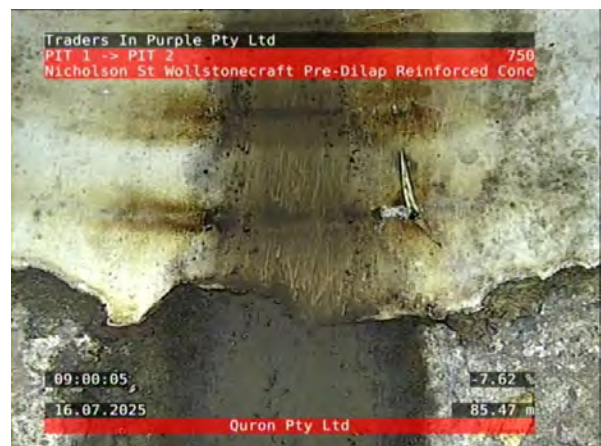
18, 00:14:52, 85.47 Change of conduit material. New material, Poly Vinyl Chloride (o, u or m)
