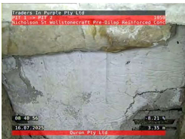
1, 00:00:40, 3.35 Change of cross section, new shape U shape, height: 750mm, width: 600mm
