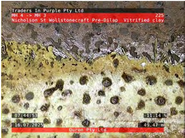
13, 00:10:51, 49.47 Point repair, localised lining--less than the complete inspection length, length: 1000mm from 12 o'clock to 12 o'clock, Start #
