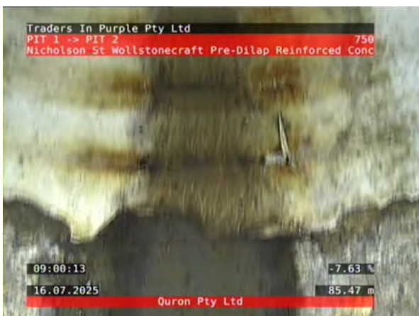
17, 00:14:48, 85.47 Change of cross section, new shape circular, height: 750mm, width: 750mm
