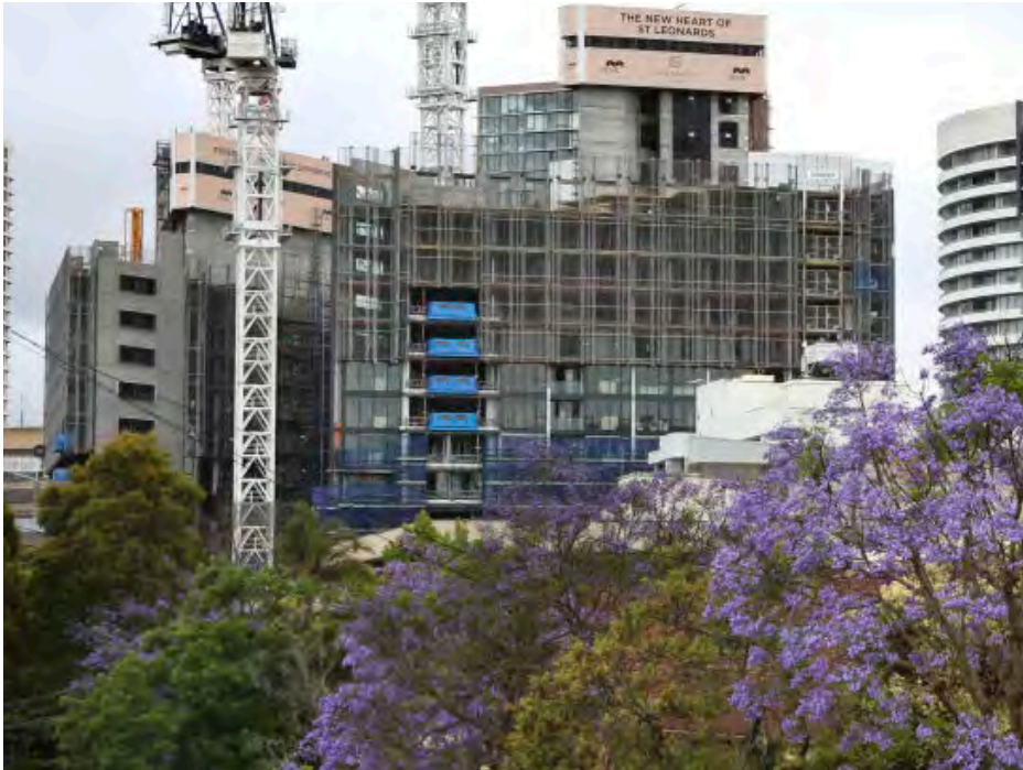
High-rise construction in Crows Nest town centre, circa. 2019.
