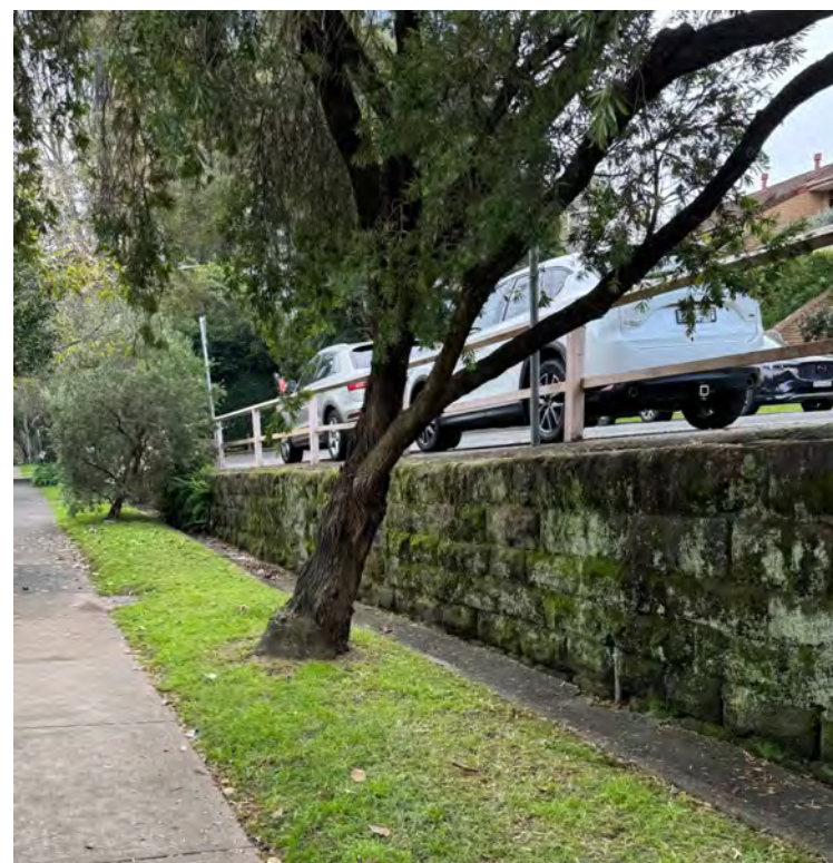
4. Existing sandstone retaining wall along Nicholson Street
