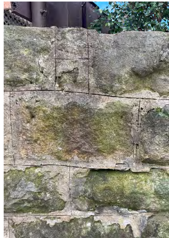
1. Existing sandstone fencing
